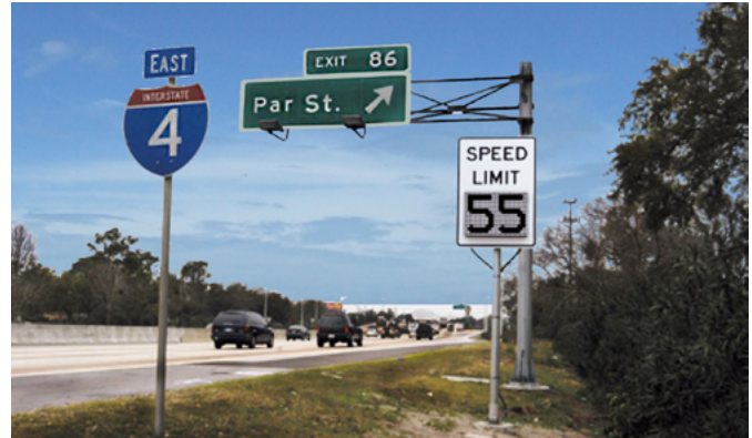
Variable speed limit (VSL) signage on I-4 in Orlando.
