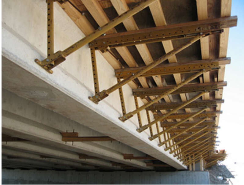
Figure 2.12 Cantilever overhang supported by overhang brackets (Photo credit: Clifton and Bayrak (2008))
