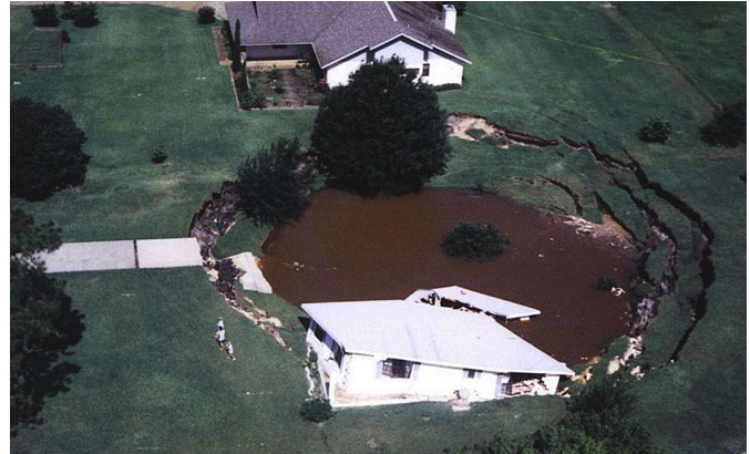
A sinkhole has destroyed one home and threatens another.
