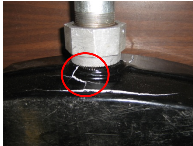
Figure A-75. DL3.2 failure mode, crack at top connection
