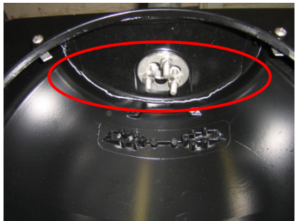
Figure A-90. SH4.1 failure mode, crack around top surface
