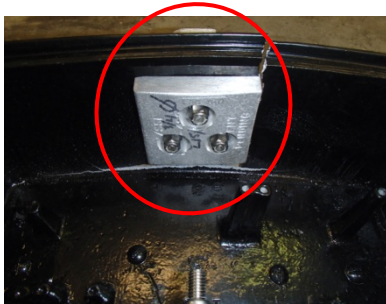
Figure A-102. RDL1.1 failure mode, crack around top reinforcement
