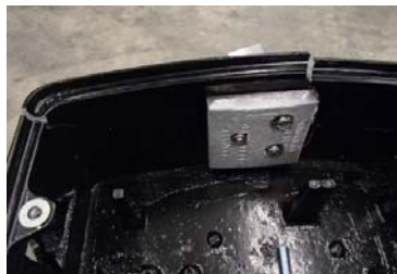
Figure 4-12. Reinforced combination failure mode, flexure (photo courtesy of author)
