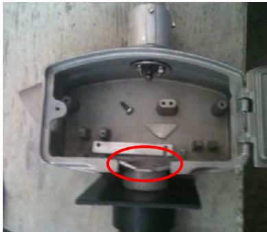
Figure A-6. DS2.1 failure mode, adapter hub failure
