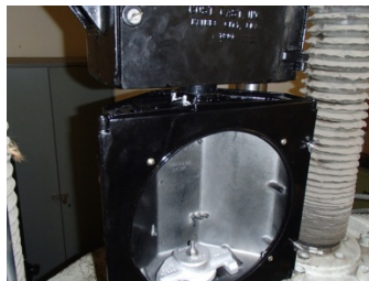
Figure 4-13. Combination failure mode, tension (photo courtesy of author)
