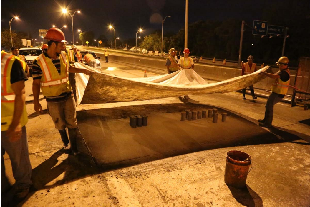
Figure 6-15. Curing of the concrete specimens and the replacement slab.
