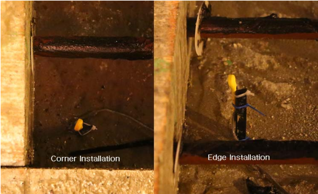
Figure 6-3. Installed temperature sensors at the corner and edge of the slab.
