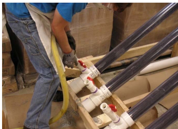
Figure 11—Attach grout hose to tube
