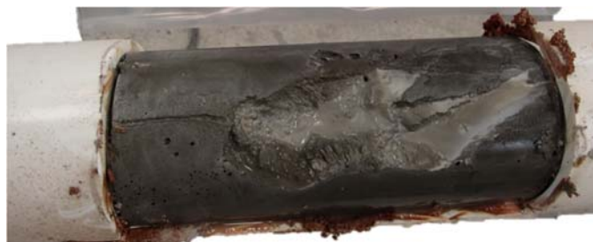
Figure 117—Soft grout located in segregation canal
