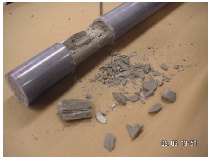
Figure 14—Grout sample removed with chisel
