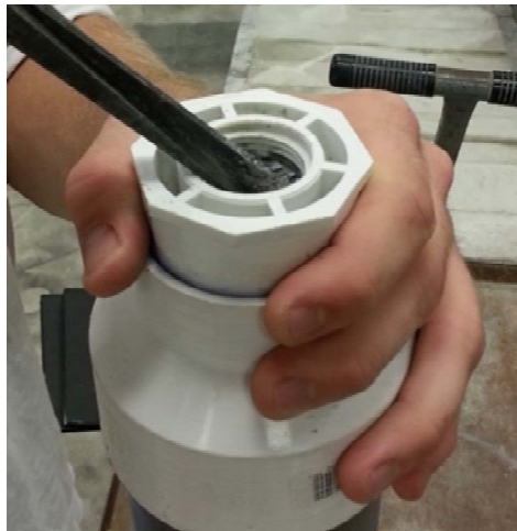
Figure 59—Soft grout found at top of constricted tube containing PT4-2 several months after injection
