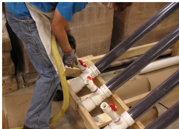
Figure 11—Attach grout hose to tube
