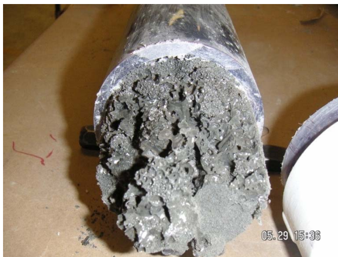
Figure 51—Porous grout observed in PT1-2 at 1.15·MWD
