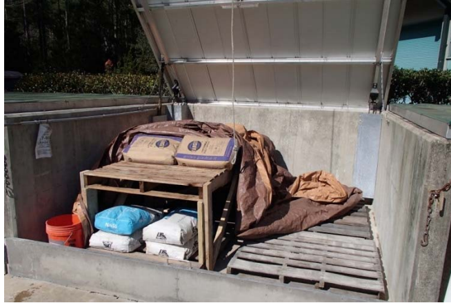
Figure 21— Field storage condition
