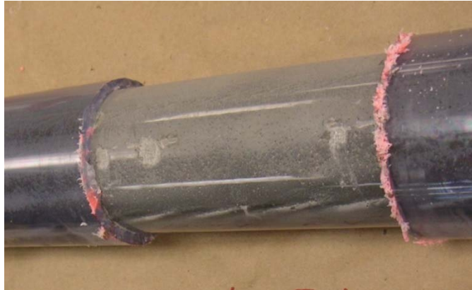
Figure 52—Smooth grout surface observed in PT2-2 mixed at MWD
