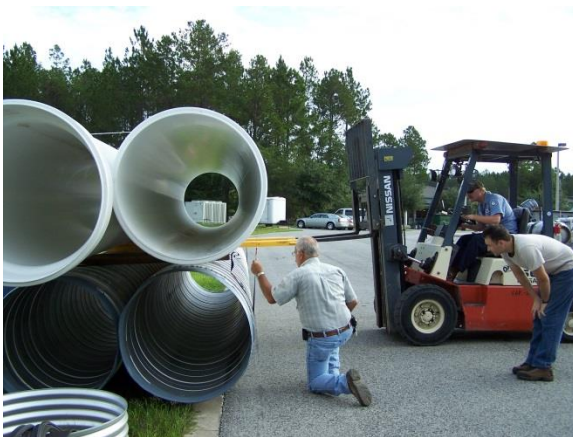
Figure 3-5: Forklift Loading PVC Pipe
