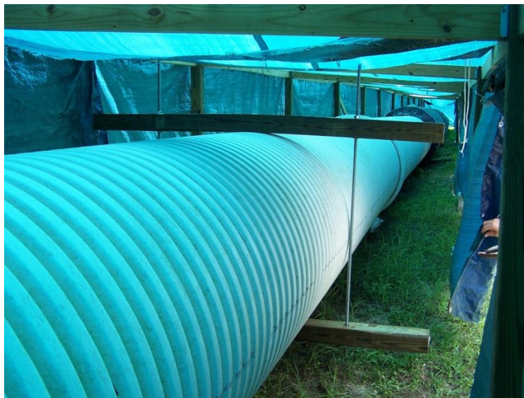
Figure 3-32: Deflection Vice on PVC Pipe
