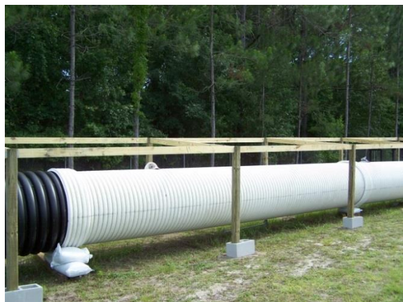
Figure 3-29: Posts with Cinderblocks
