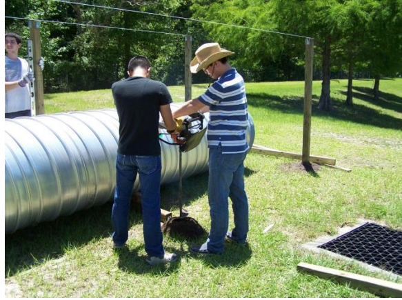
Figure 3-25: Drilling Post Holes
