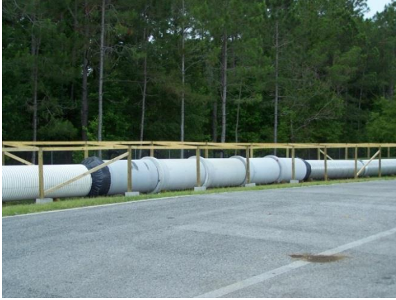
Figure 3-30: Diagonal Cross-Bracing
