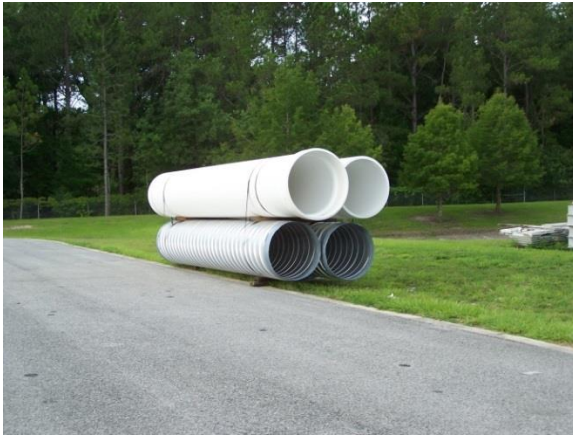
Figure 3-3: Delivery of PVC and CMP
