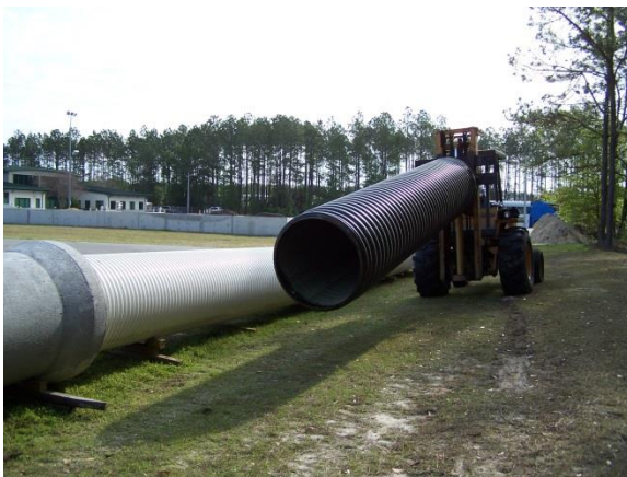
Figure 3-13: Relocating Pipe Segments
