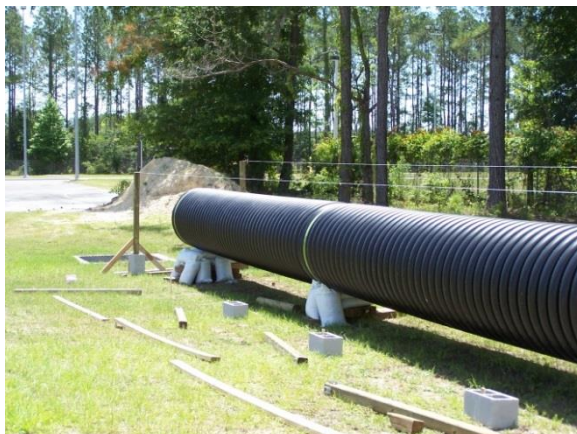
Figure 3-22: Corner Posts (East End)
