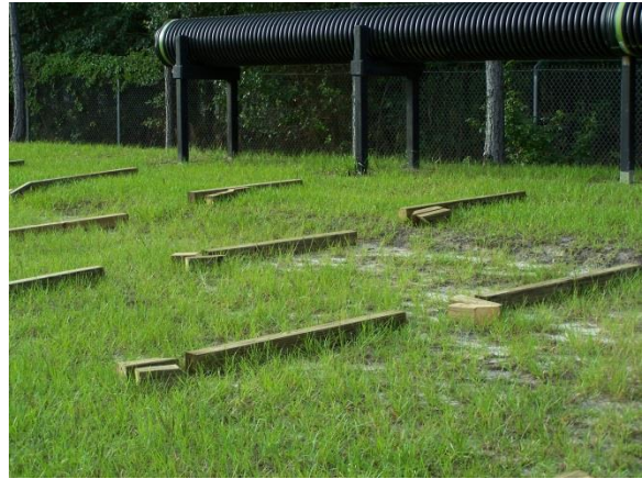
Figure 3-4: Lumber Supports and Chocks
