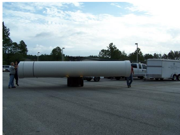
Figure 3-6: Forklift Moving PVC Pipe
