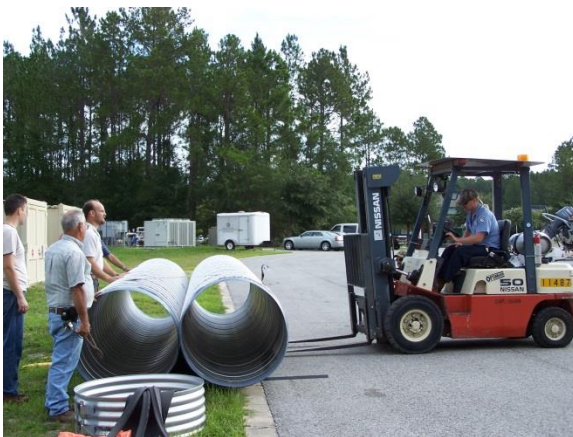
Figure 3-7: Forklift Loading CMP
