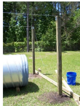
Figure 3-23: Corner Posts (West End)
