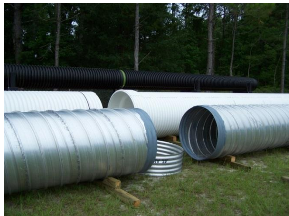
Figure 3-8: Positioned PVC and CMP
