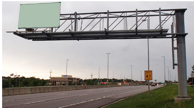
Wind loading on cantilevered highway signs creates large torsional forces on the base plate connections.
