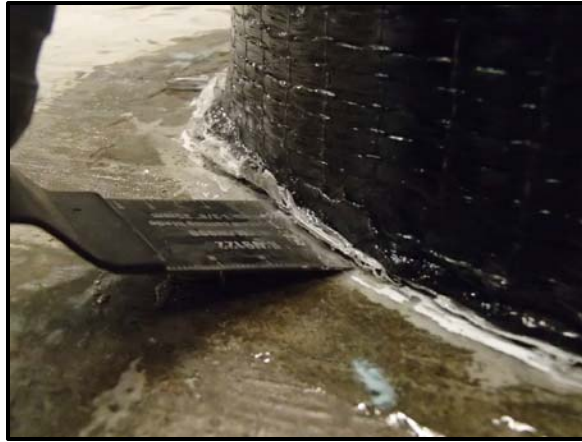
Figure 4-6. Cutting away excess epoxy material after cure
