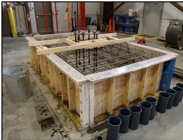
Figure 4-20. Full-scale anchor bolt and rebar and rebar placement before casting concrete
