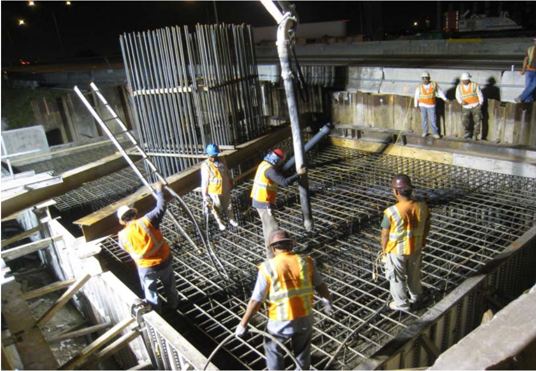
Figure 5-4. Concrete being placed for Footing 1.
