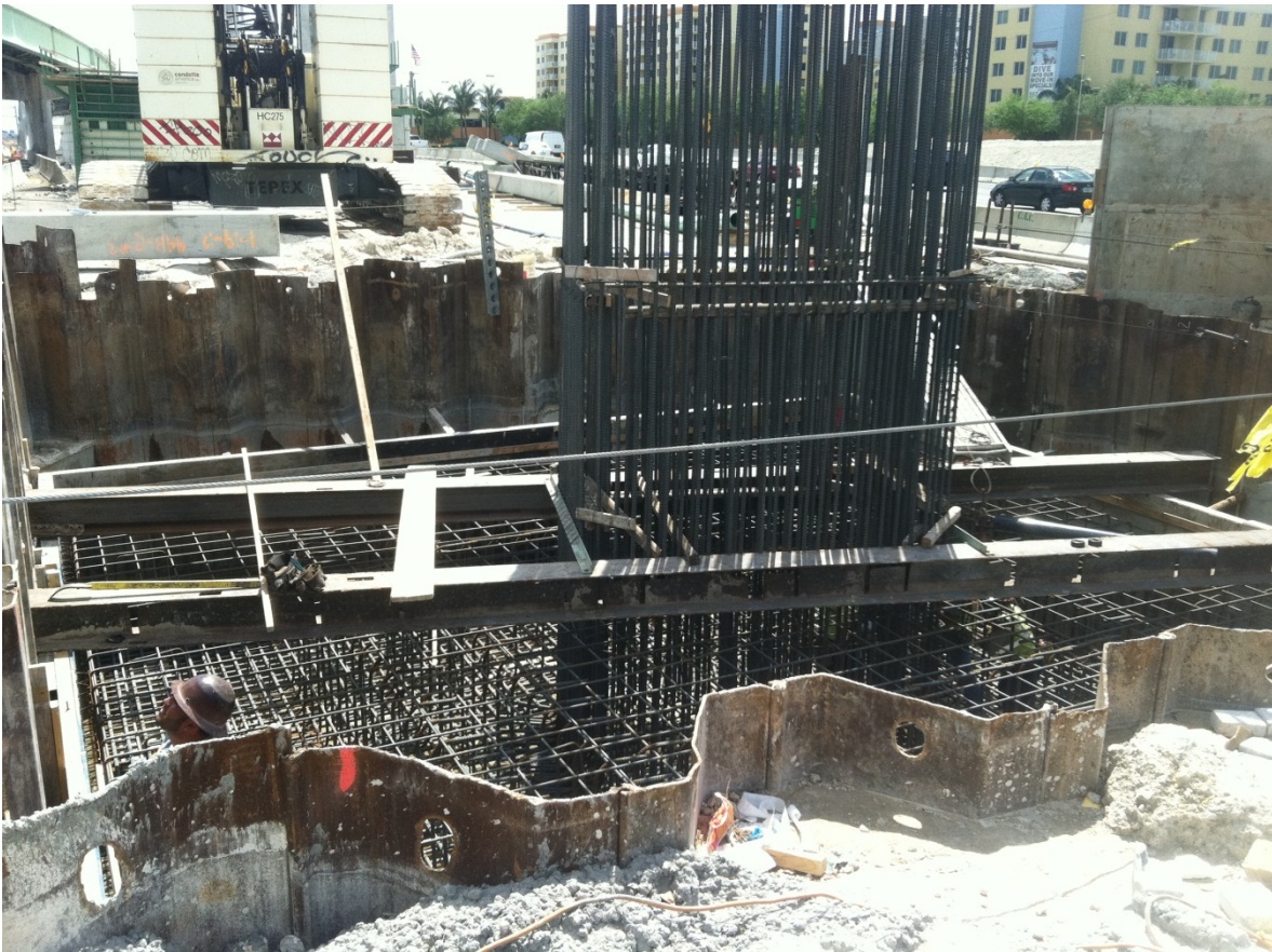
Figure 5-12. View of Footing 2.
