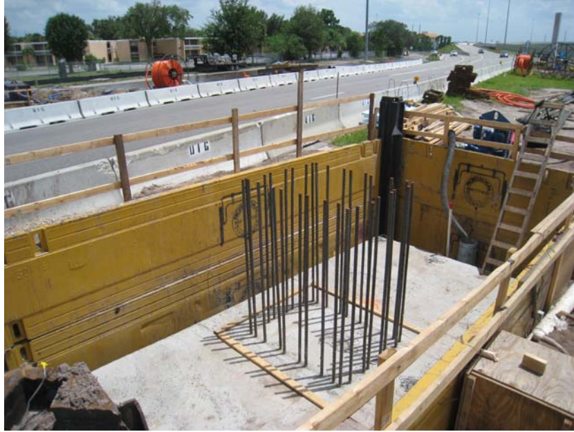
Figure 5-19. Footing at I-4 US-192 Braided Ramp, Orlando, FL.
