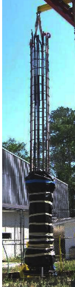
Rebar cage fitted with grouting system and side membrane is lowered into a prepared hole prior to concreting.
