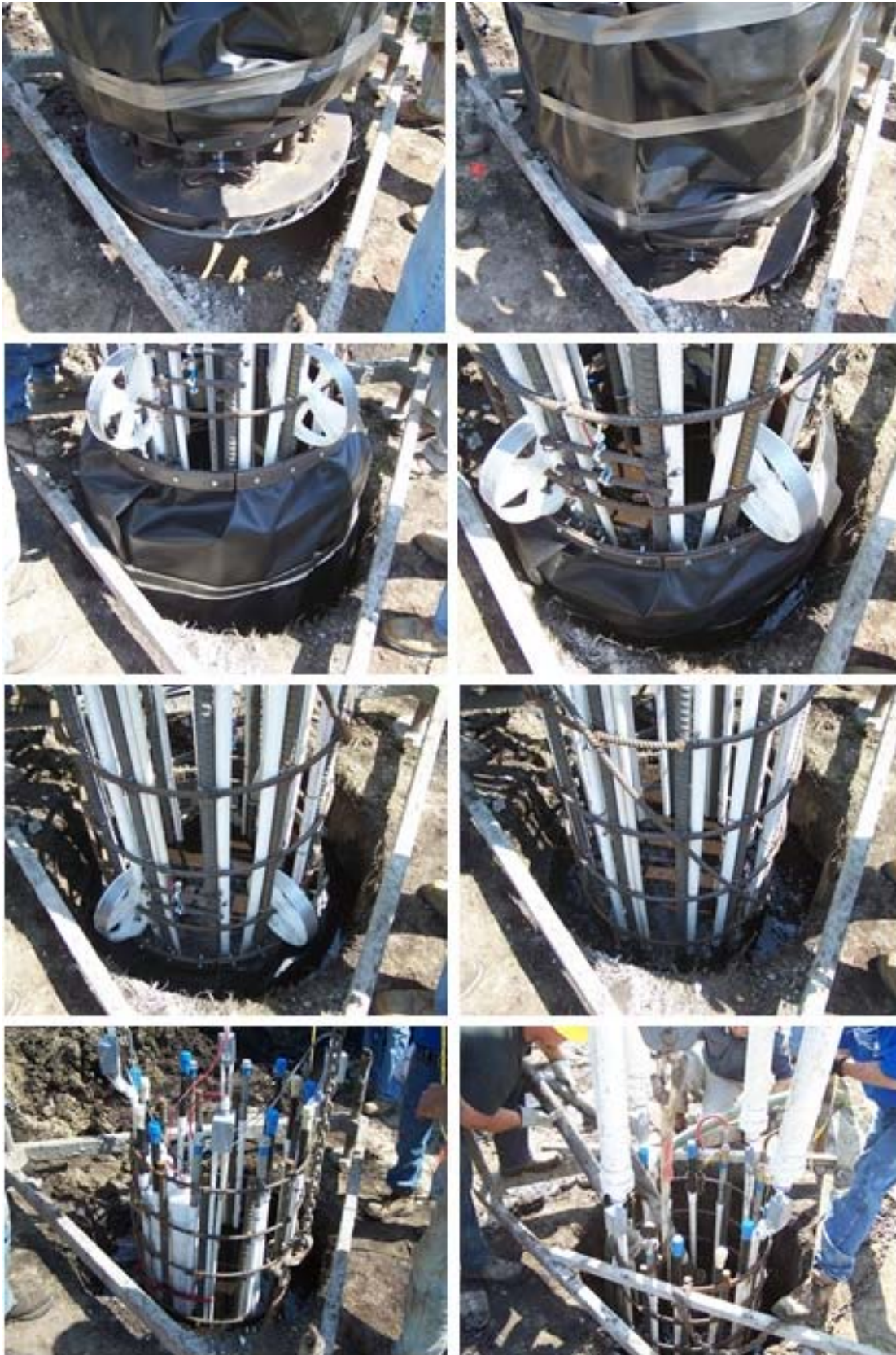
Figure 3-54: Lower cage with grout systems attached into hole
