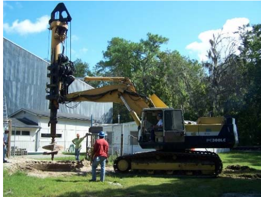
Figure 2-29: Track-mounted drill rig used to excavate soil from test chamber
