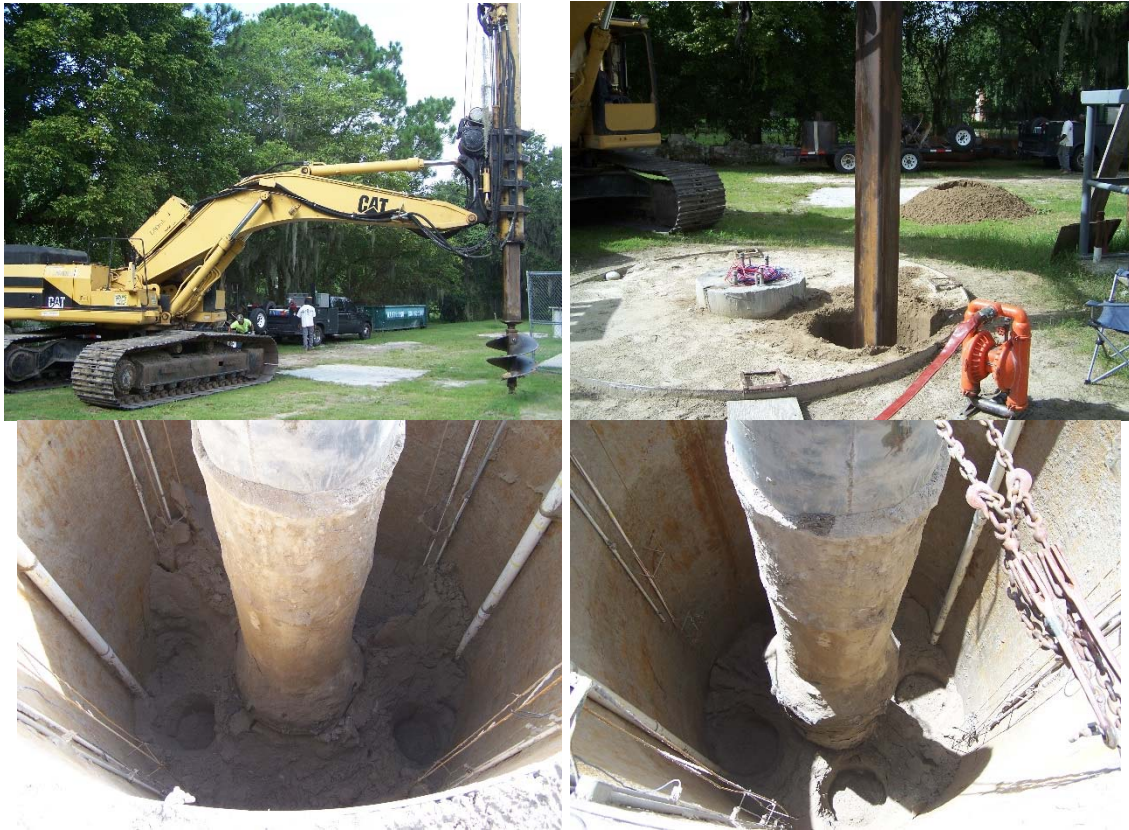
Figure 2-70: Excavate soil from test chamber using track-mounted drill rig
