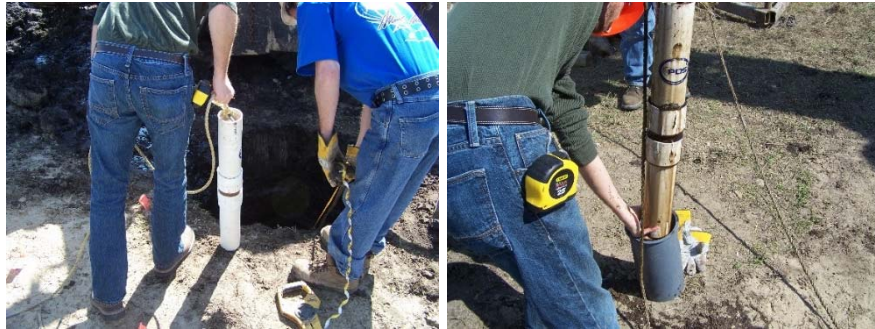
Figure 3-50: Recover slurry sample for quality check
