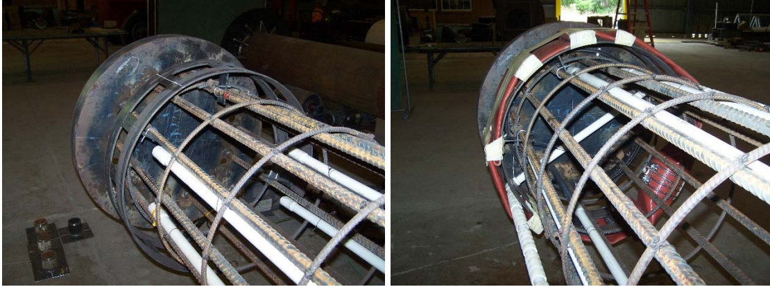
Figure 2-26: Membrane seal steel rings fabricated to prevent seal from inflating inwards
