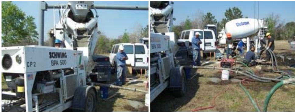
Figure 3-56: Concrete pump (left) used to place concrete with split tremie (right)
