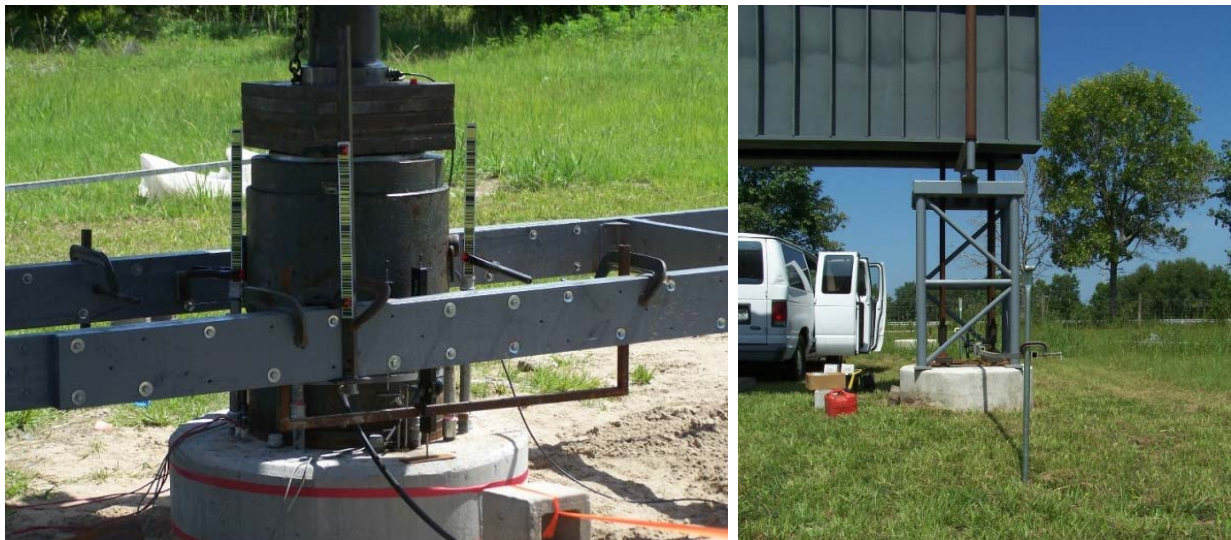
Figure 3-67: Digital dial gauge setup during static load test (left - grouted shaft; right - reaction shaft)
