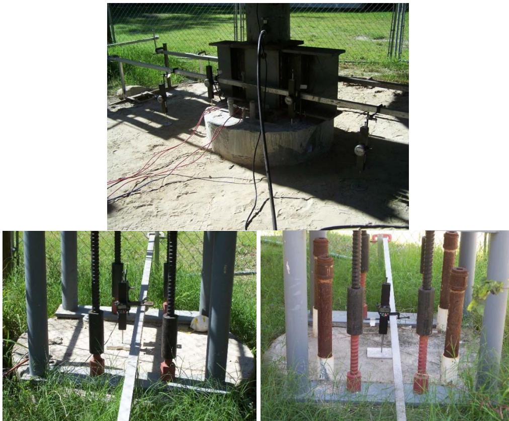
Figure 2-68: Digital dial gauge setup during static load test (test shaft and soil – top photo; reaction shafts – bottom photos)
