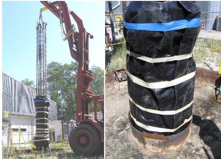
Figure 2-56: Placing long shaft rebar cage with grout systems attached in casing
