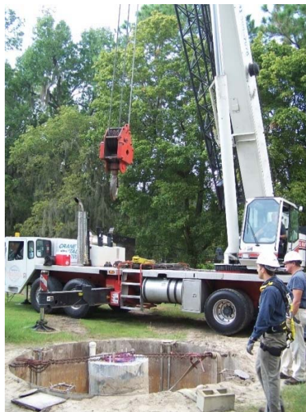
Figure 2-71: Crane used to exhume shaft from test chamber
