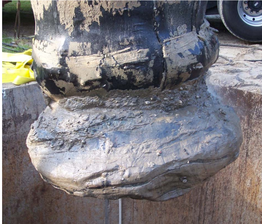
Figure 4-19: Close-up of tip-grouted zone as long shaft was removed from test chamber
