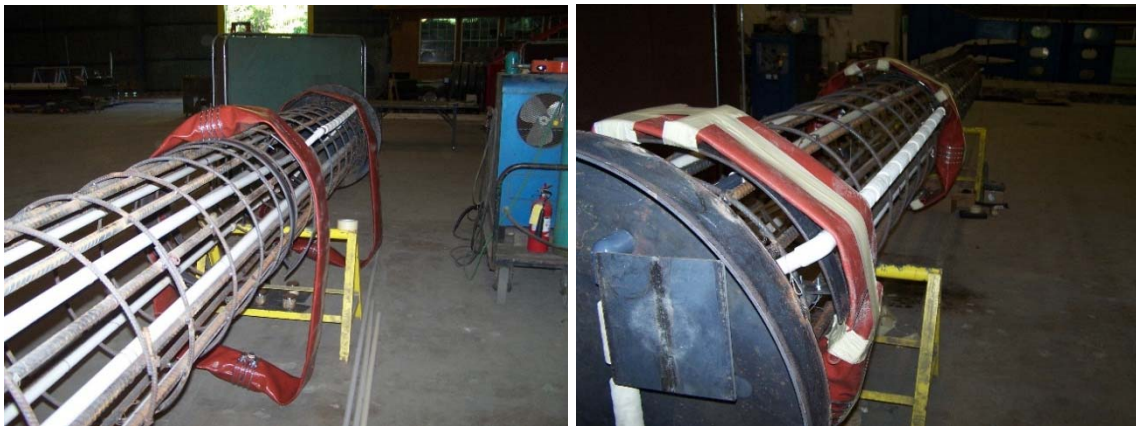
Figure 2-46: Securing membrane seals to inner steel rings
