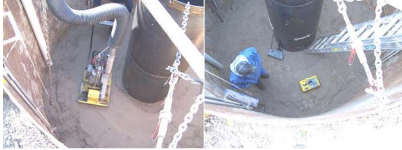
Figure 2-41: Backfilling soil in test chamber
