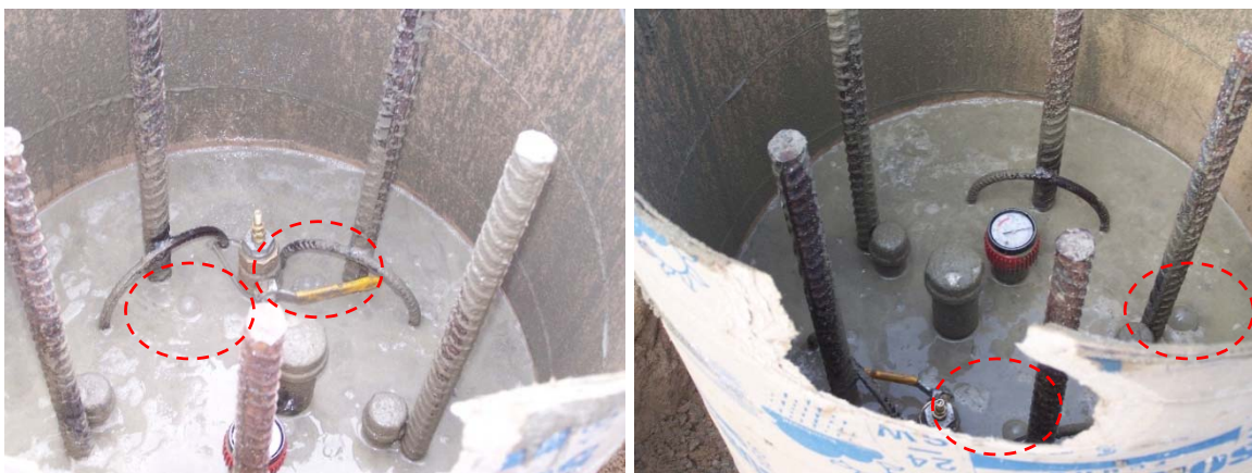
Figure 2-19: Air bubbles observed during shaft construction
