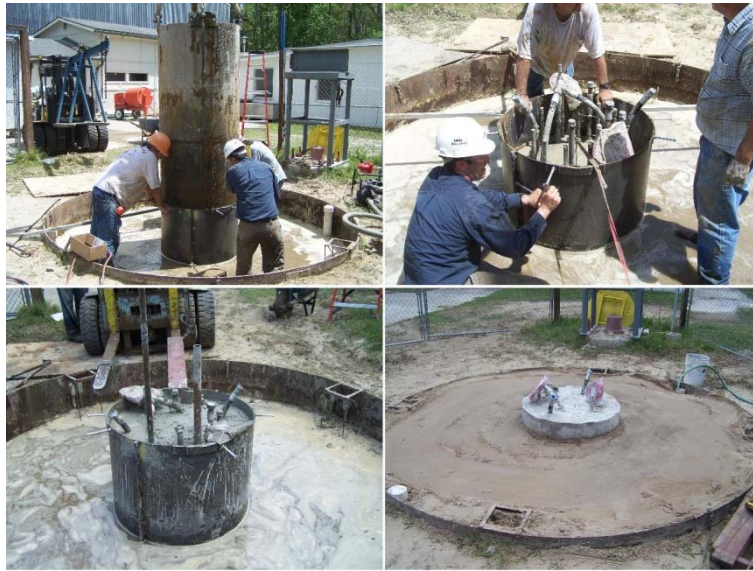
Figure 2-59: Securing the shaft form at the end of shaft construction
