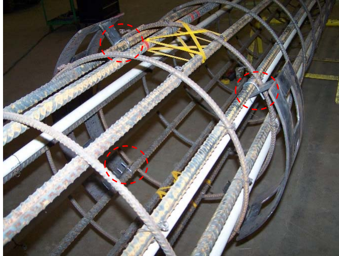
Figure 2-52: Inner rings for membrane seals attached to rebar cage using U-bolts
