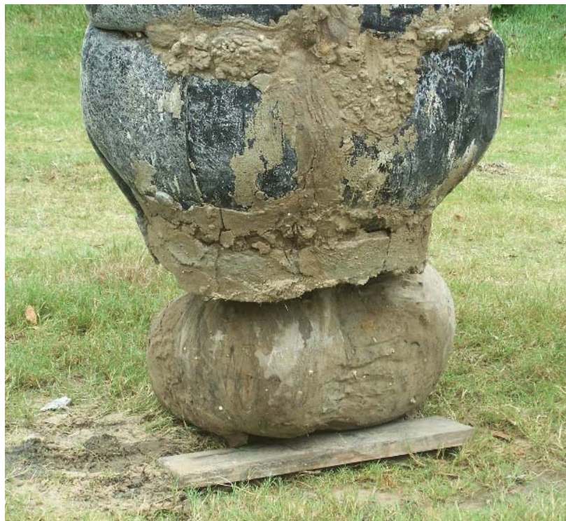
Figure 4-7: Tip grout bulb on short test shaft
