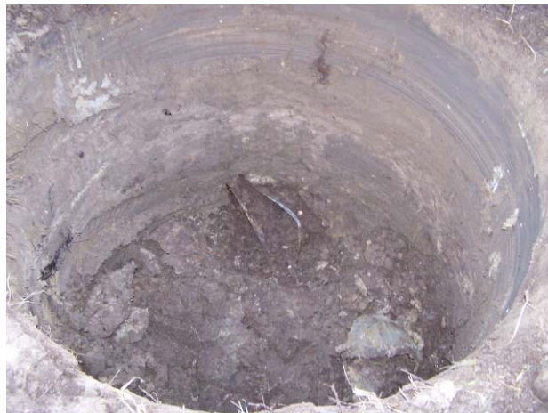
Figure 3-46: Debris struck at three-foot drilling depth
