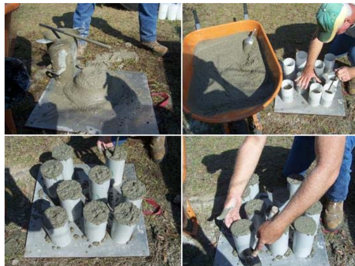
Figure 3-57: Check slump of concrete mix (top left) and prepare test cylinders
