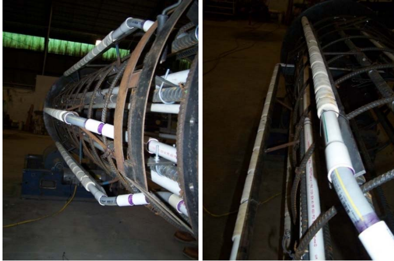
Figure 3-38: Side membrane grout delivery pipes with steel reinforcing members
