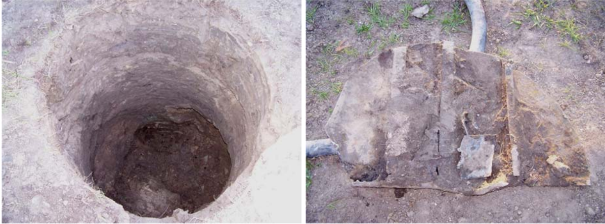
Figure 3-47: Debris struck at five and a half foot drilling depth
