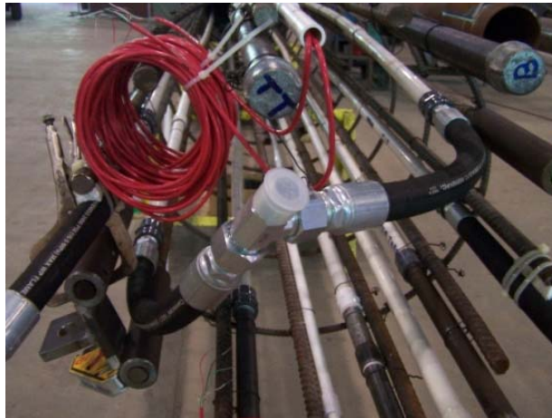
Figure 2-54: Steel nipples and high pressure hydraulic hose at the top of rebar cage
