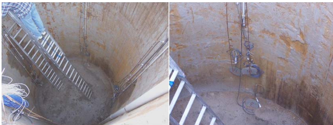
Figure 2-35: Securing the pressure cells to steel racks before backfilling soil
