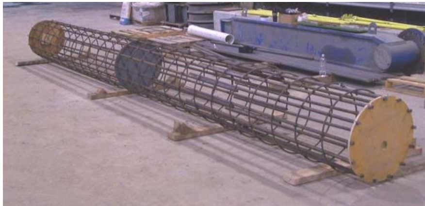
Figure 2-43: Long shaft rebar cage
