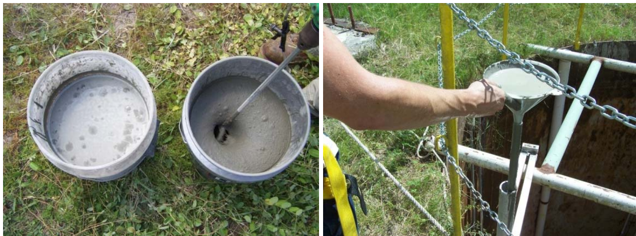
Figure 3-75: Small batches of non-shrink grout (left) and gravity-driven grout flow through tremie/frame (right)
