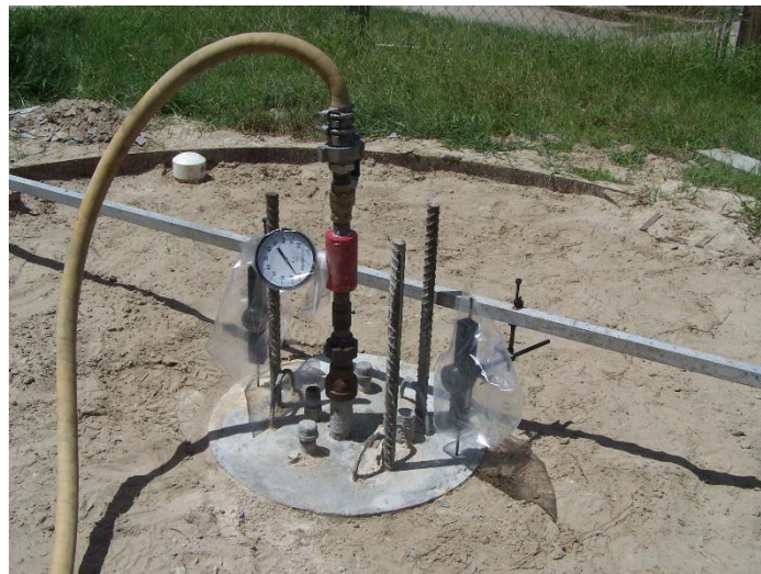
Figure 2-20: Top of short shaft during tip grouting
