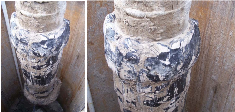
Figure 4-9: Top of side membrane/side grouted zone (location of top membrane seal)
