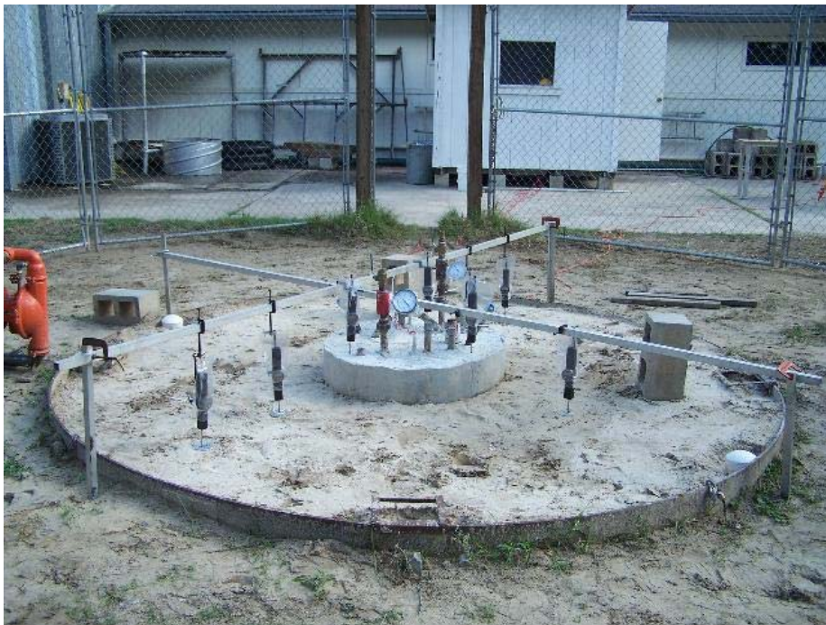
Figure 2-62: Digital dial gauge setup during side grouting
