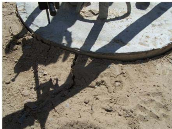
Figure 4-3: Ground surface during side grouting of short shaft
