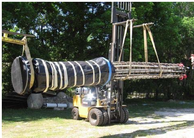
Figure 2-55: Completed long shaft rebar cage with grout systems attached
