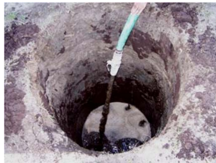
Figure 3-48: Use drilling slurry after drilling to depth of eight feet
