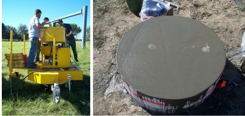
Figure 3-77: Small grout pump used to grout instruments and place grout for cap (left) and grout cap (right)
