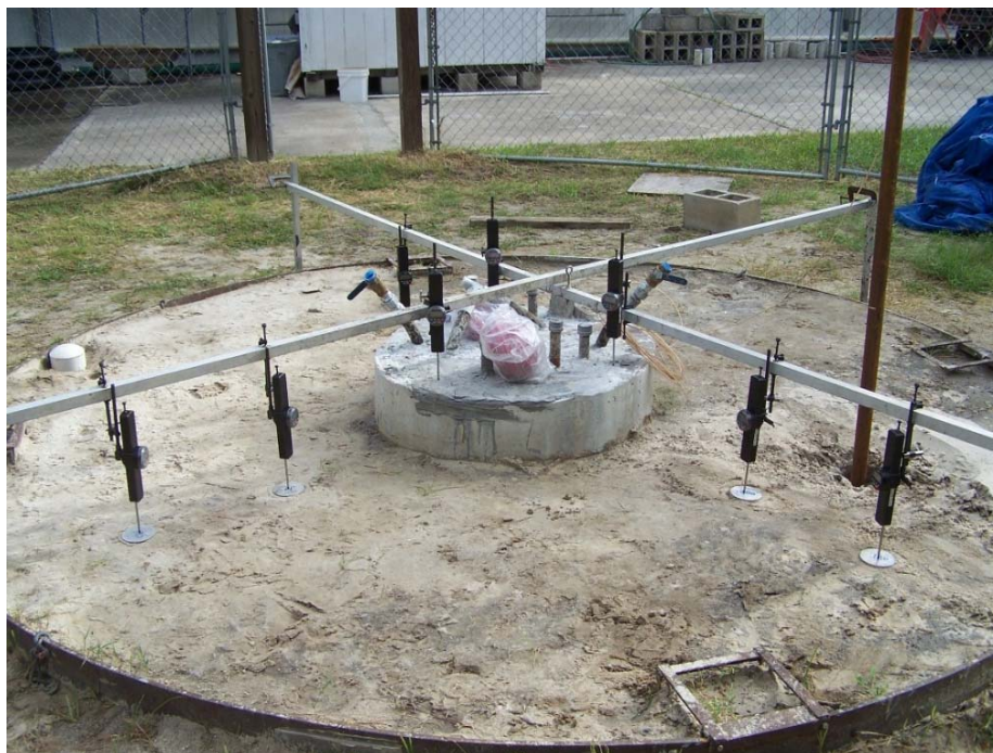
Figure 2-63: Digital dial gauge setup during tip grouting
