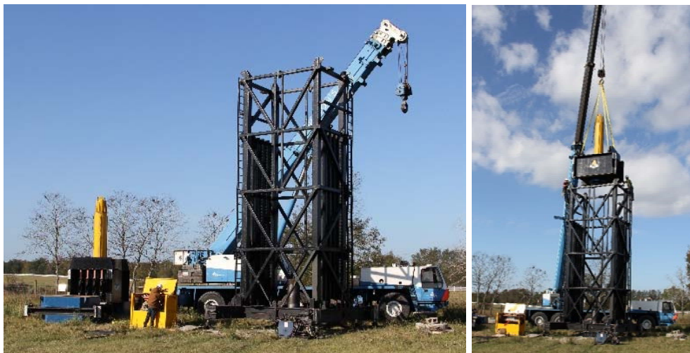
Figure 3-78: Statnamic system (crane, catch frame, and dead weights)
