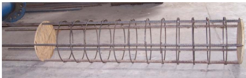
Figure 2-5: Short shaft rebar cage
