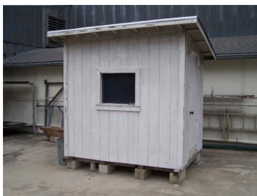
Figure 2-36: Shed where pressure cell wires convene
