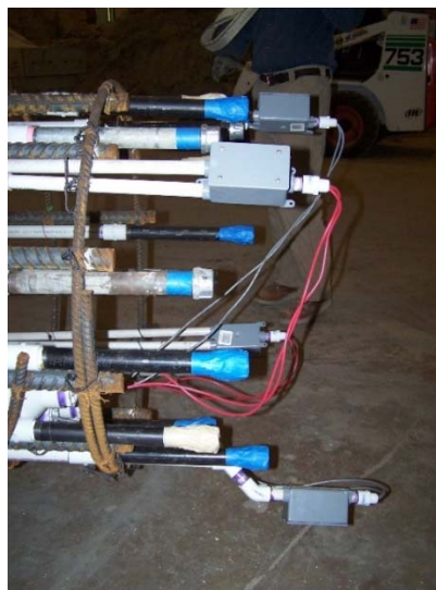
Figure 3-43: Steel nipples at the top of cage
