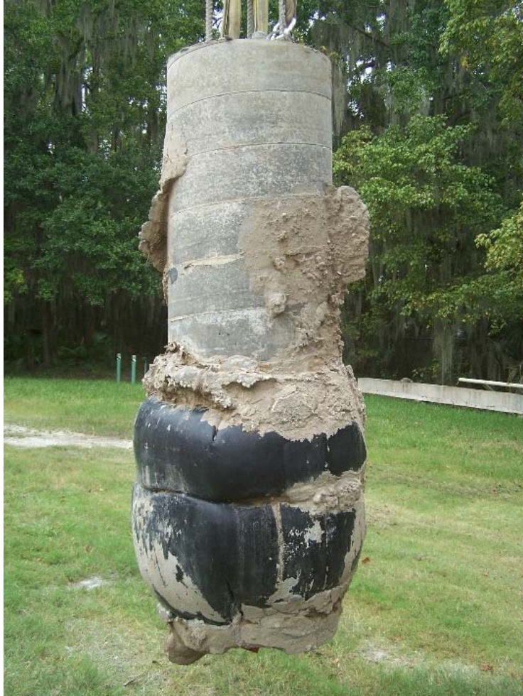
Figure 4-1: Short test shaft being removed from test chamber (tip grout bulb not shown)
