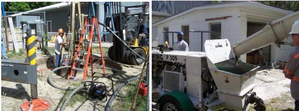
Figure 2-57: Concrete pump (right) and tremie (left) used to place concrete during long shaft construction
