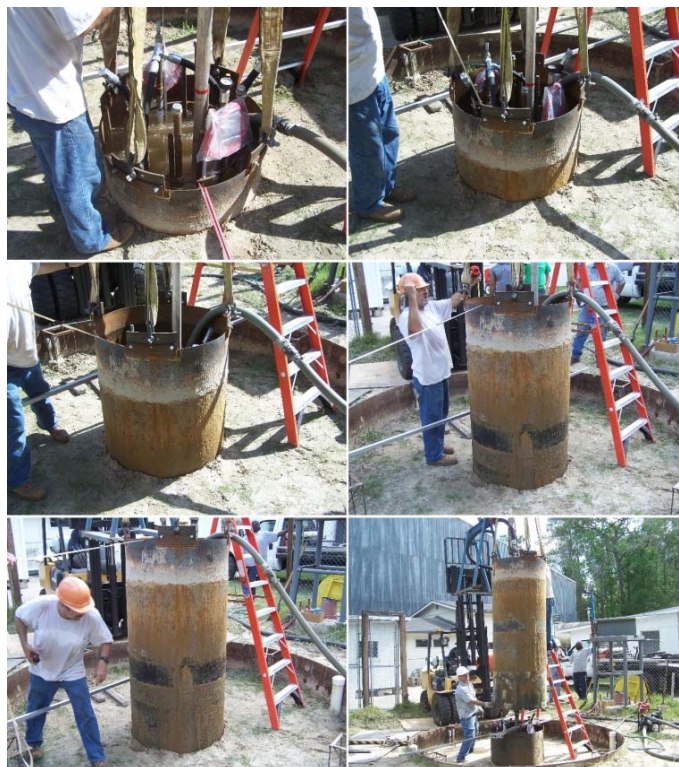
Figure 2-58: Removing temporary casing during concrete placement
