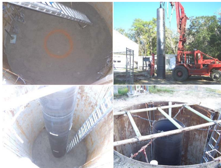
Figure 2-40: Casing placement before backfilling soil
