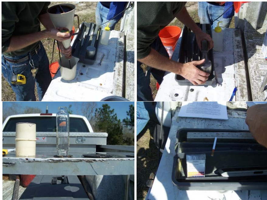
Figure 3-51: Checking slurry quality during shaft construction
