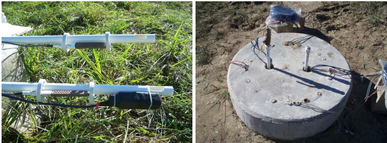
Figure 3-76: Final tremie/frame with instruments attached (left) and tremie/frame with instrumentation attached fully lowered in holes before grouting (right)
