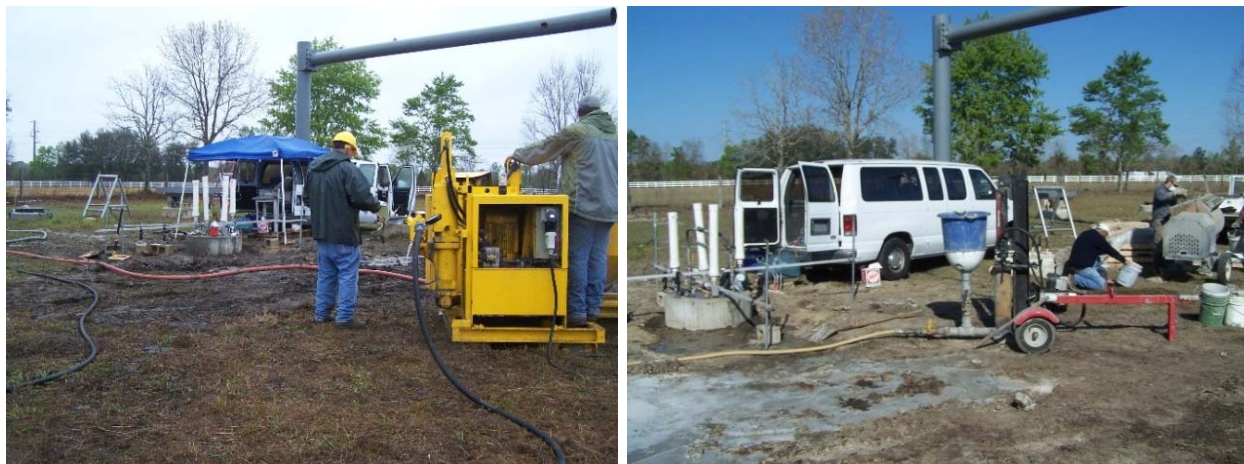
Figure 3-60: Side grouting using AFT's grout pump (left) and UF's grout pump (right)
