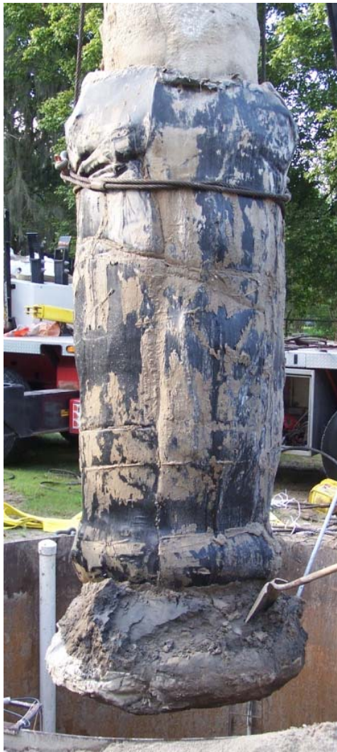
Figure 4-17: Close up of side grouted zone as long shaft was removed from test chamber
