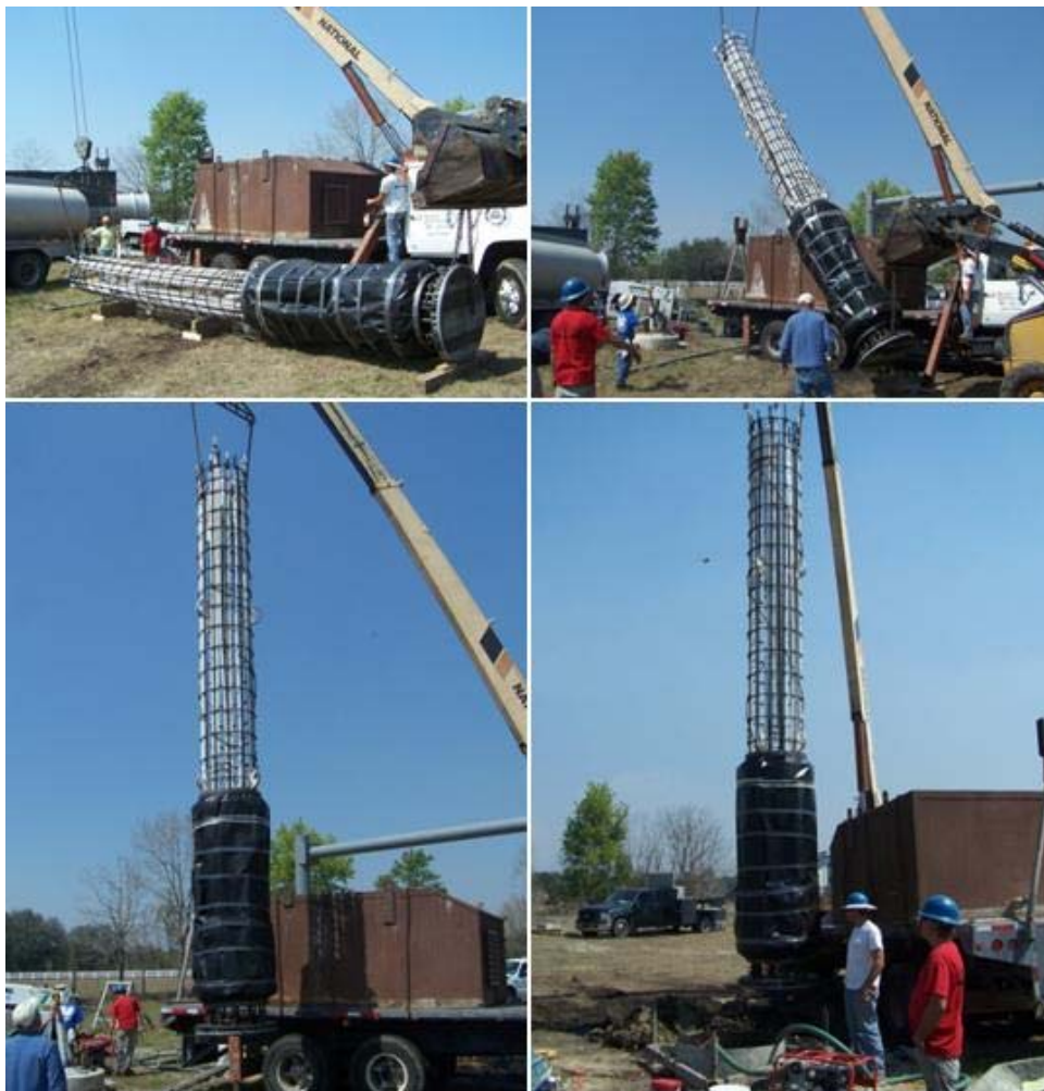
Figure 3-53: Lift rebar cage and maneuvered to hole
