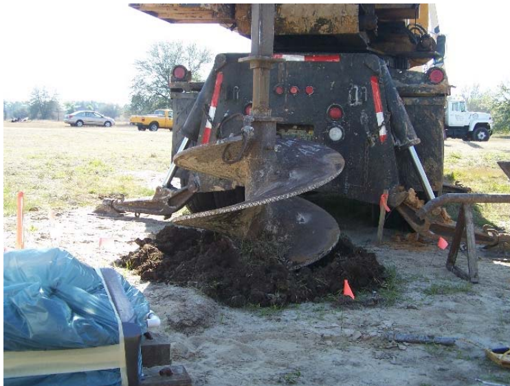
Figure 3-45: Truck-mounted drill rig used to drill hole
