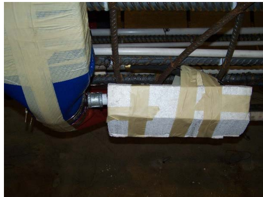
Figure 3-36: Styrofoam used to prevent flexible hose from becoming embedded in shaft
