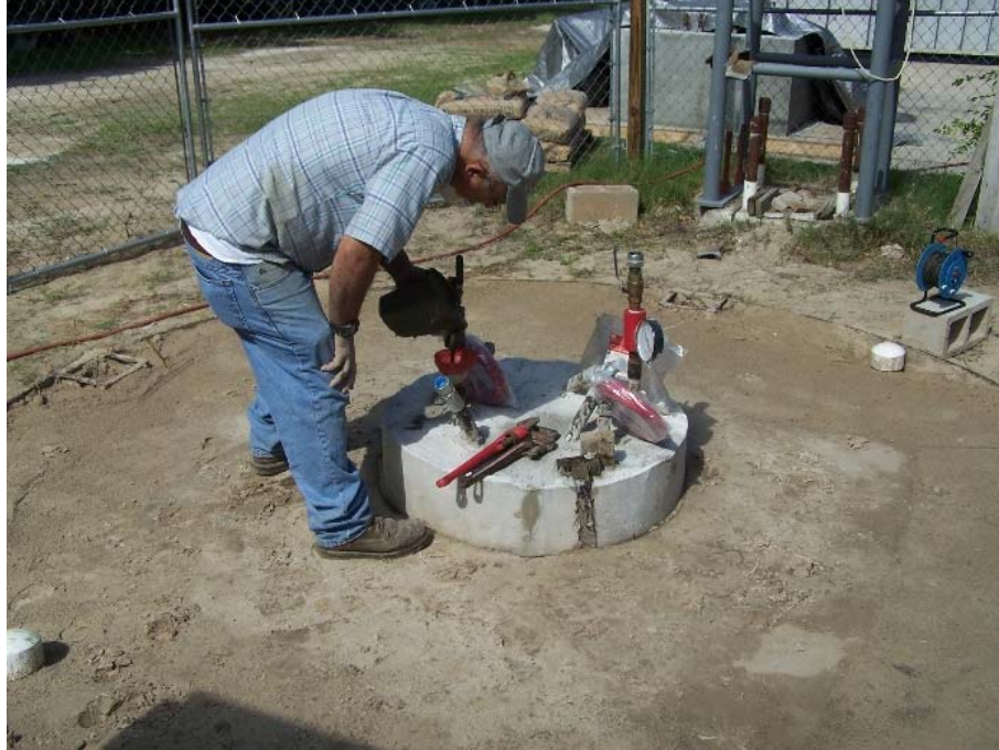
Figure 2-60: Filling grout pipes (priming) with grout before pumping under pressure
