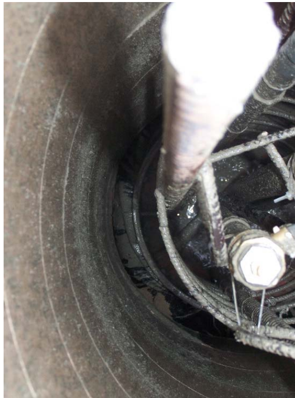
Figure 2-18: Pressurized membrane seal successfully pressing side membrane against wall of shaft
