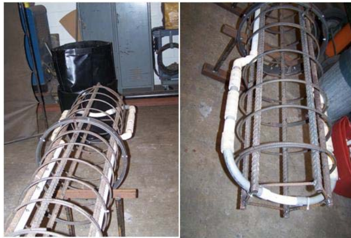
Figure 2-12: Grout delivery pipes for side membrane (side-manchette)
