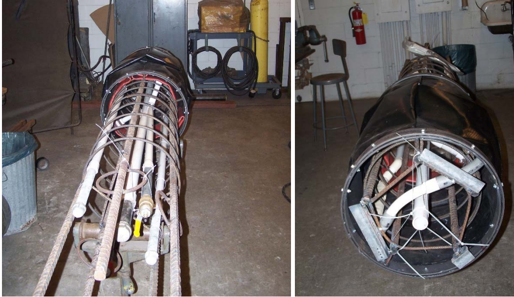
Figure 2-14: Completed short shaft rebar cage with grout systems attached
