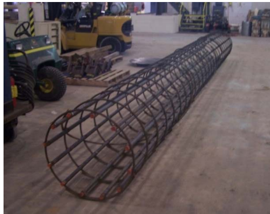
Figure 3-27: Field shaft rebar cage
