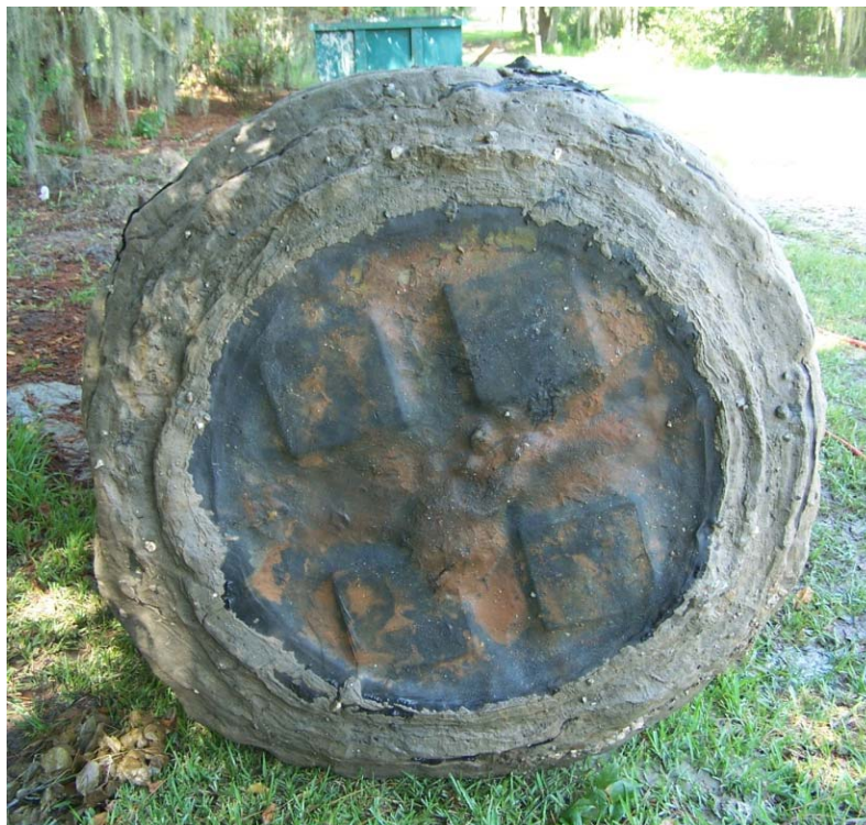
Figure 4-20: Bottom of tip-grouted zone of long shaft
