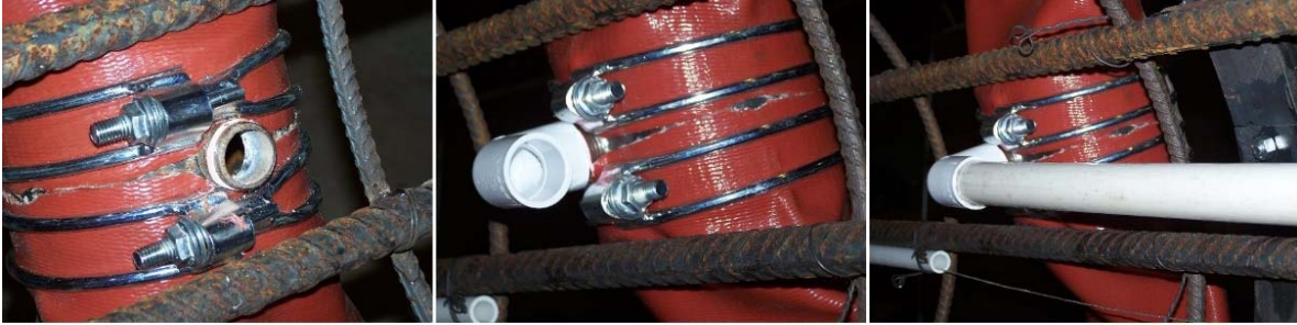
Figure 2-45: Grout delivery pipe connection to membrane seal
