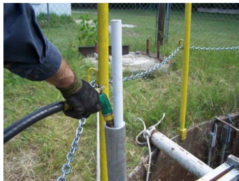
Figure 3-74: Fill pipe with water before placing grout
