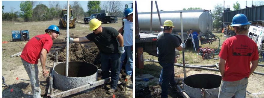
Figure 3-52: Shaft form centered and leveled at top of hole (42 inch diameter)
