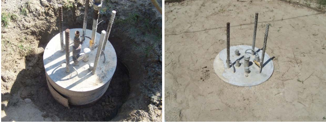
Figure 2-17: Removed Sonotube and backfill around short shaft
