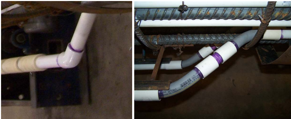
Figure 3-15: Replace short radius 45^\circ elbows (left) with long radius 45^\circ elbows (right)
