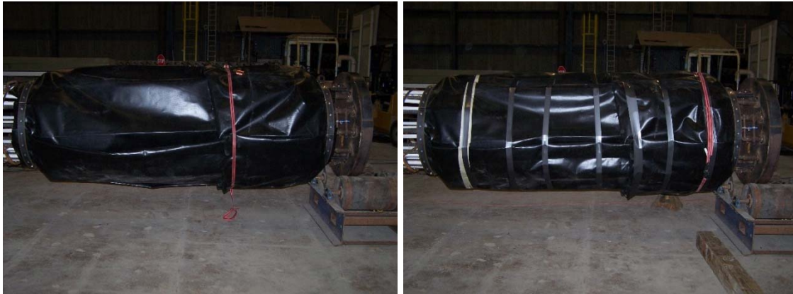
Figure 3-40: Side membrane pleated and secured to rebar cage
