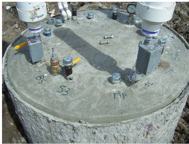
Figure 3-58: Top of shaft before grouting membrane seals
