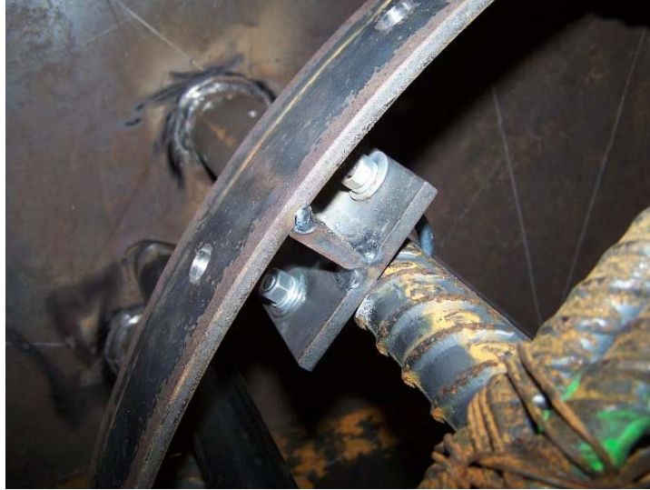
Figure 3-37: Mechanical connection used to secure inner side membrane steel rings
