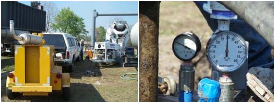
Figure 3-55: Air compressor (left) and pressurize membrane seals (right)
