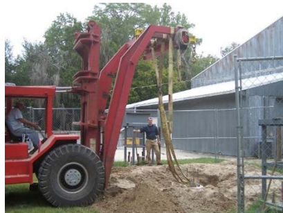
Figure 2-22: Large forklift used to remove the short shaft from test chamber
