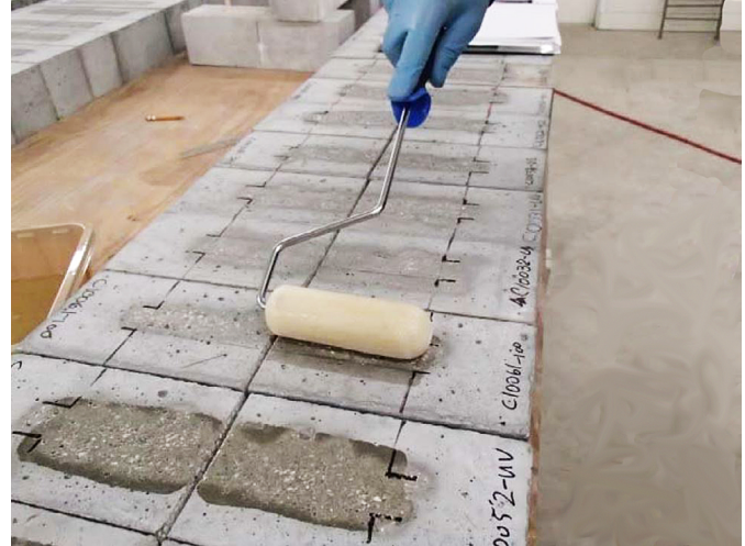
Concrete test beams are primed to receive FRP strips adhered with epoxy.
