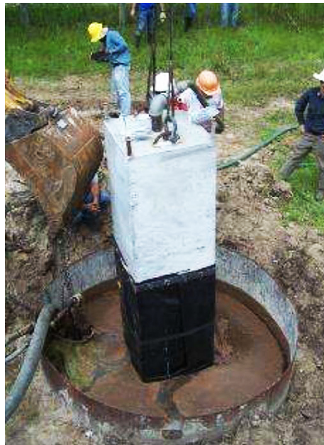
The precast pile is jetted into the ground.
