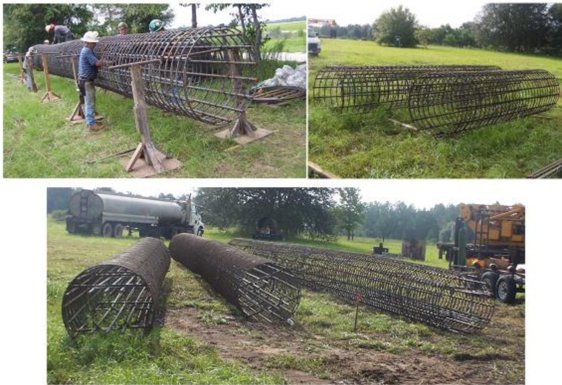
Figure 4-6. Construction of reinforcing cage
