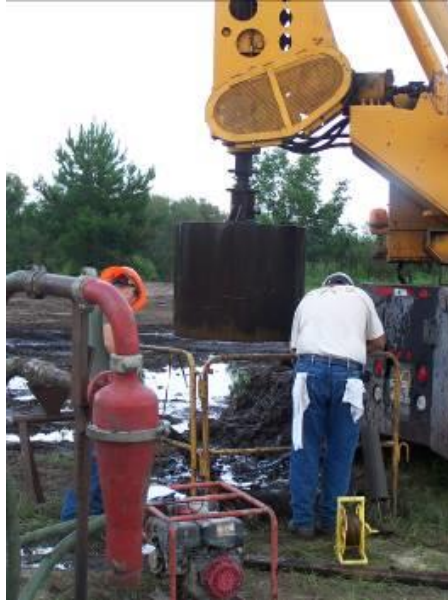
Figure 4-12. Bailing bucket used for cleaning the excavation bottom
