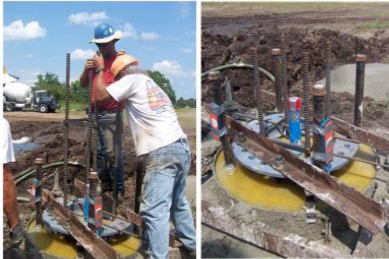
Figure 4-22. Installation of Dywidag cage within pipe and flange section
