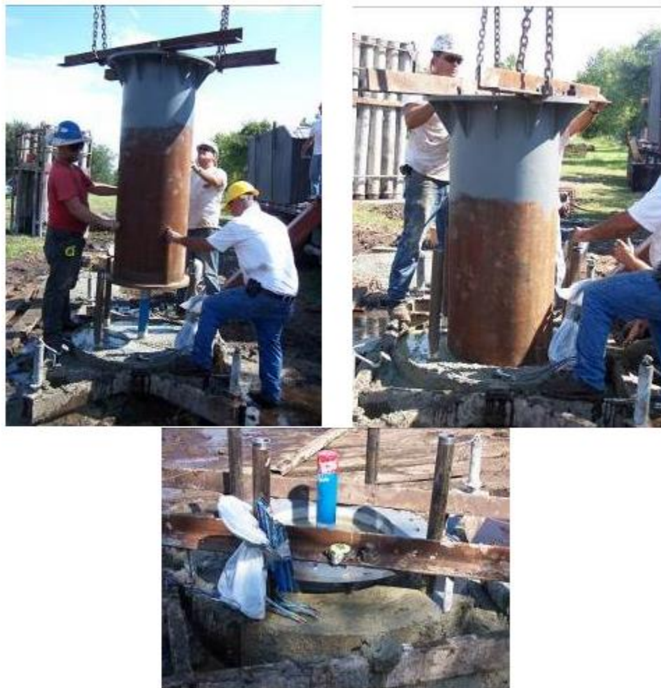
Figure 4-21. Installation of embedded pipe and flange section
