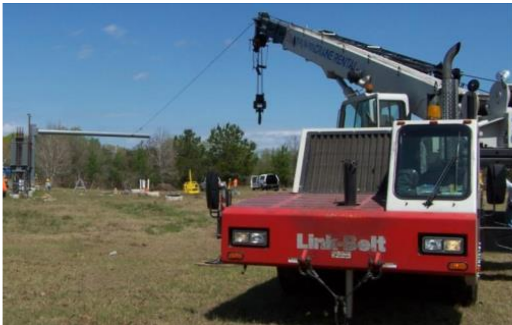
Figure 7-25. Application of lateral load on the arm by pulling with a crane
