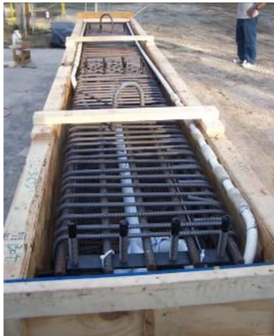
Figure 5-7. Reinforcement cage within the formwork ready for concrete placement
