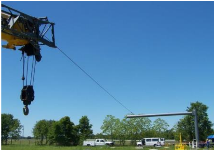
Figure 7-14. Combined torsion and lateral loading on the 18-ft-long drilled shaft (TS2)
