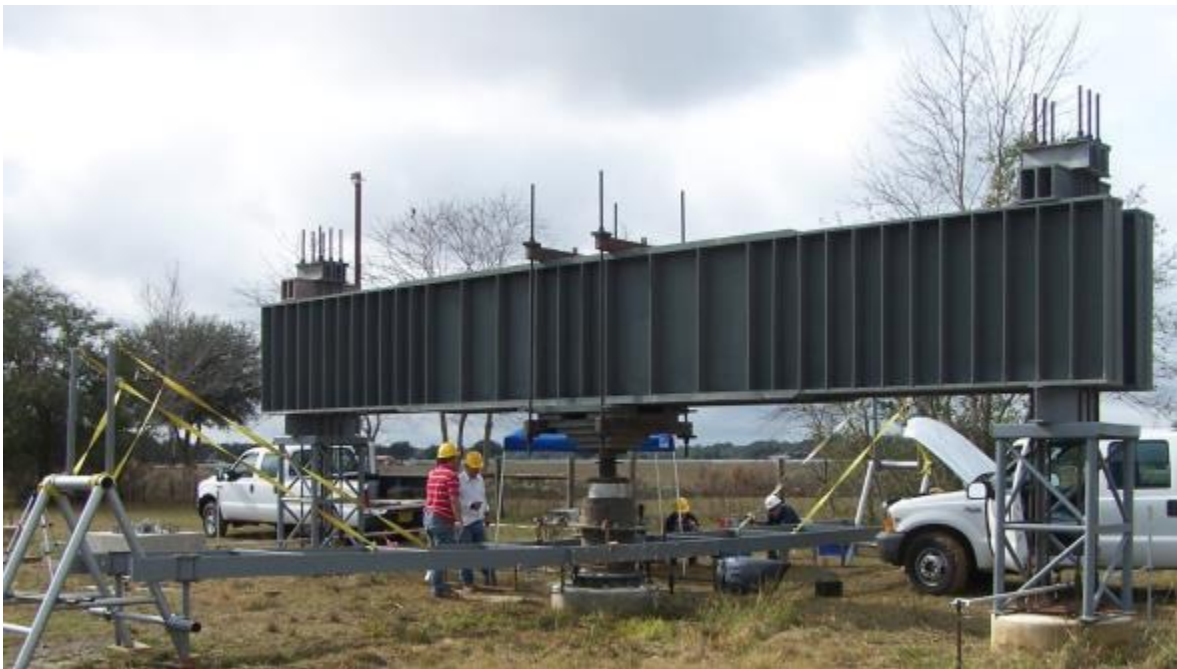
Figure 6-2. Load test setup for the 4-ft diameter x18-ft-long drilled shaft (TS2)
