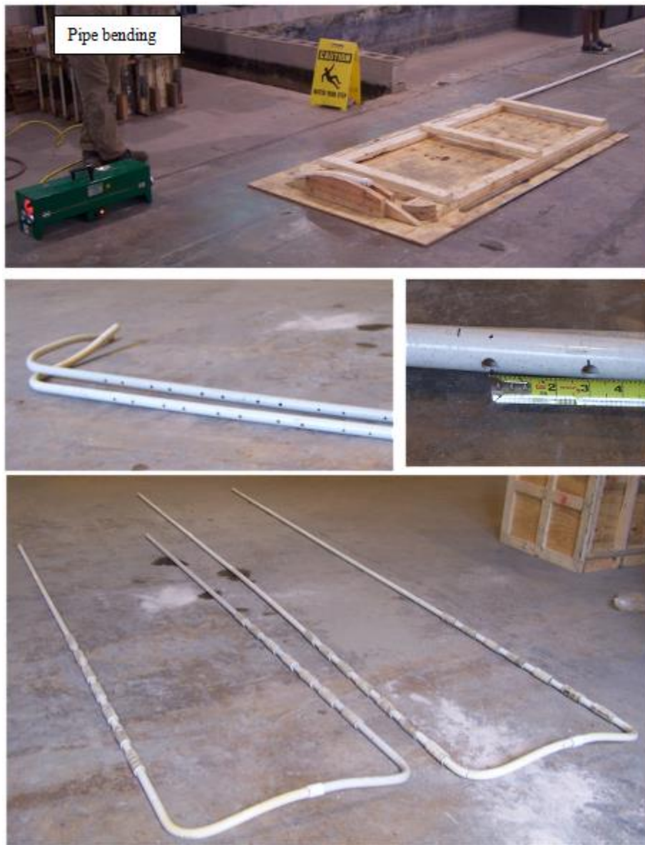
Figure 5-3. Grout delivery systems for side grouting
