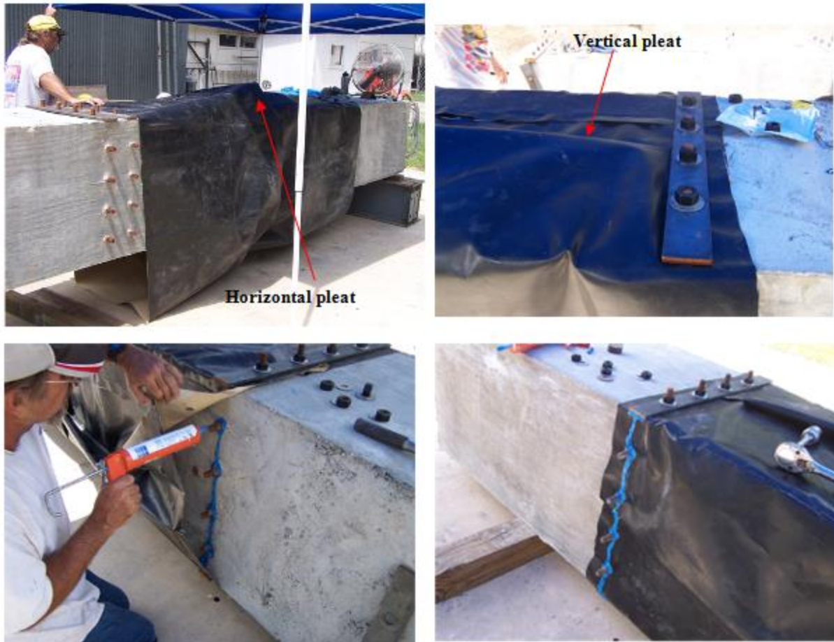
Figure 5-13. Attaching membrane to pile
