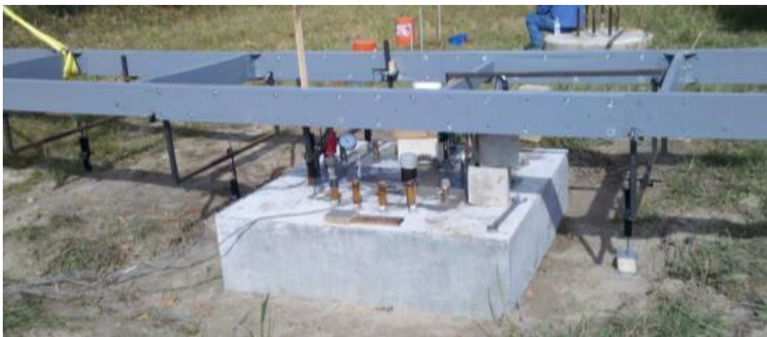
Figure 5-29. Grout pressure and displacement measurement
