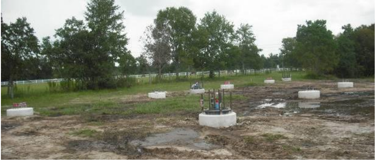
Figure 4-23. Test site with reaction and test drilled shafts.
