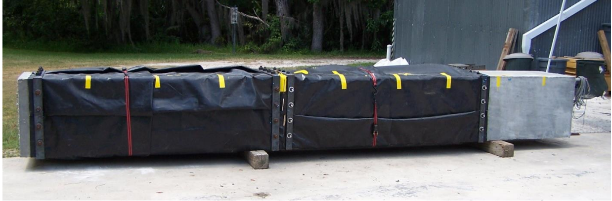
Figure 5-14. Pile after attaching the grout membranes
