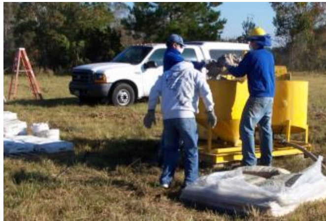
Figure 5-28. Grout mixing
