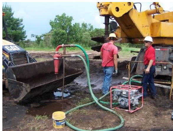
Figure 4-11. Desanding the bentonite slurry
