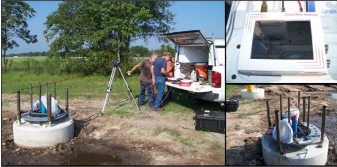
Figure 4-24. CSL testing setup for test shaft
