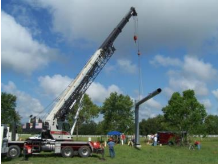
Figure 7-3. Setting mast arm assembly on the top of shaft using a crane
