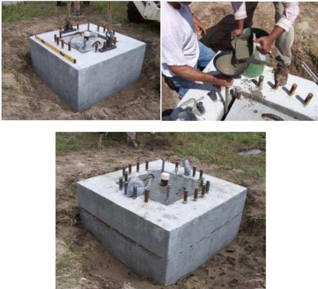
Figure 5-27. Precast cap placement and grouting
