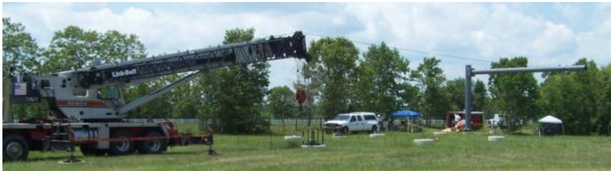
Figure 7-8. Applying lateral load to mast arm
