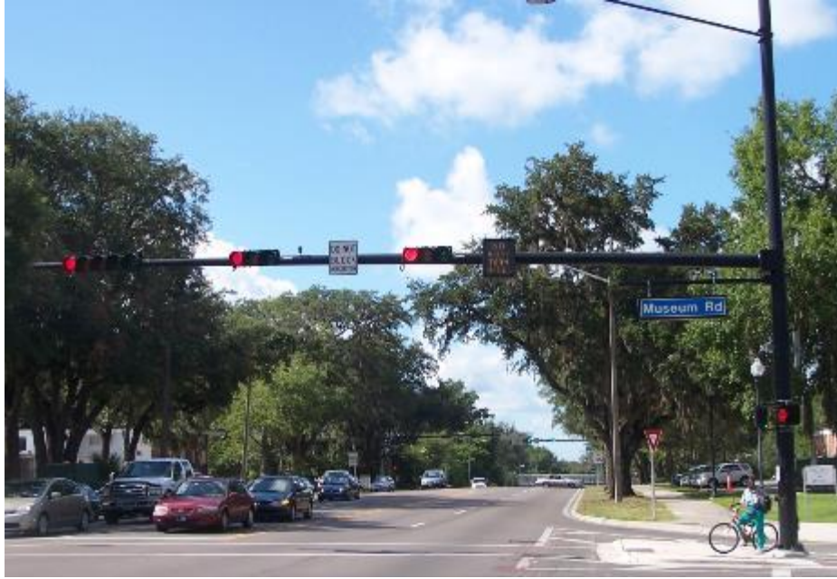
Figure 2-7. Mast arm structures supporting highway signs, signals, and luminaries
