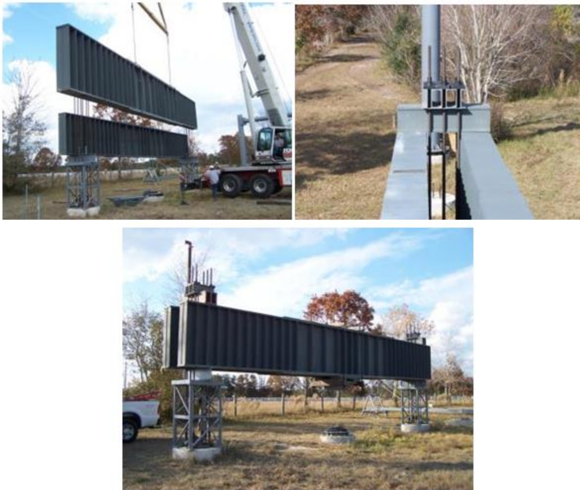
Figure 6-1. Setting reaction beam girders on the top of reaction support stands
