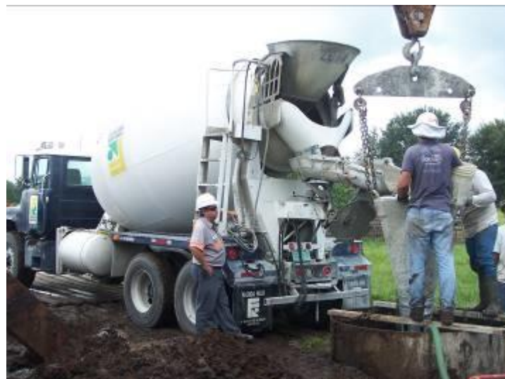
Figure 4-14. Concrete placement
