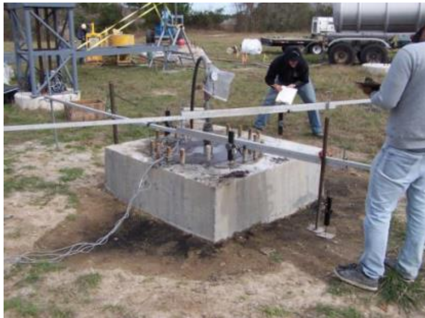
Figure 5-33. Grout pressure and displacement monitoring
