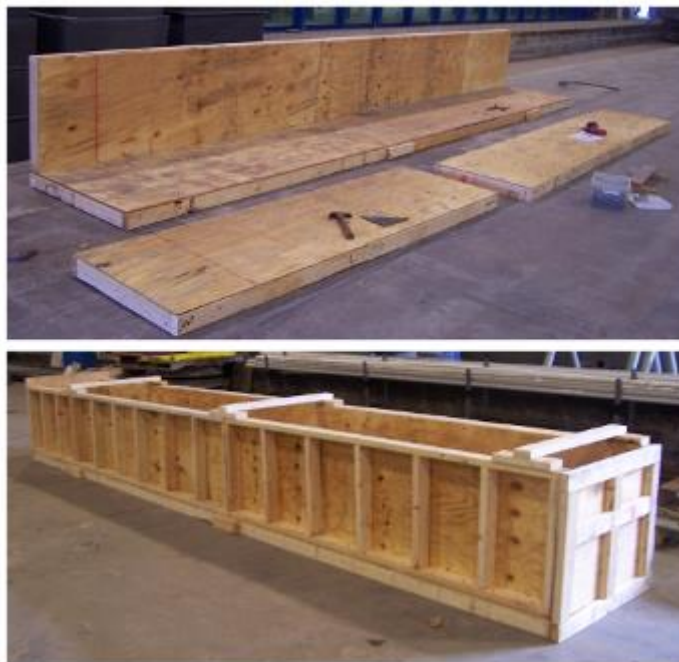
Figure 5-5. Formwork for precast piles
