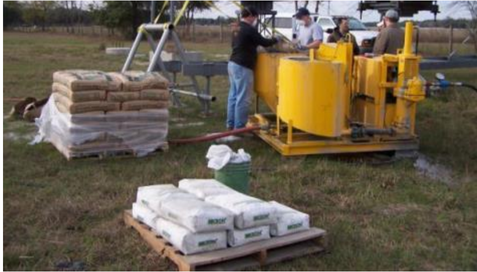
Figure 5-32. Grout mixing and pumping
