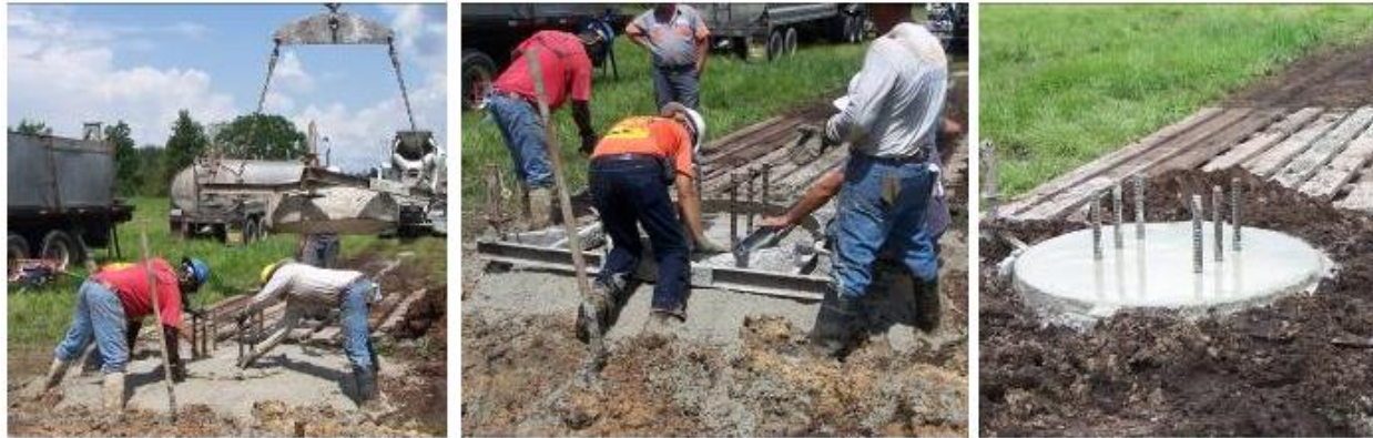
Figure 4-15. Forming the shaft top with the use of a template
