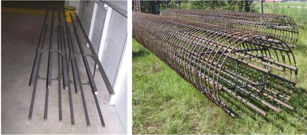
Figure 4-8. Reinforcing cage with Dywidag bars
