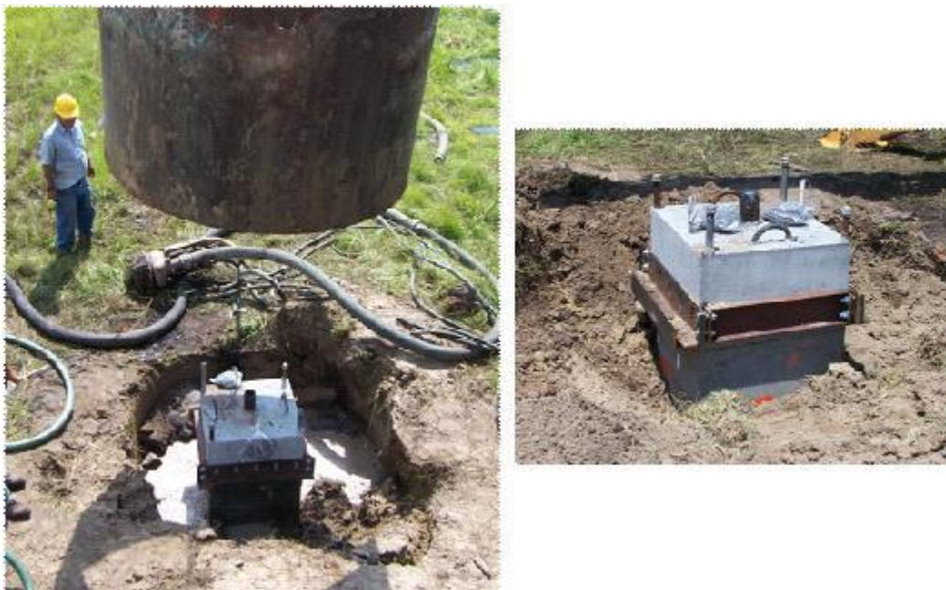
Figure 5-18. Pulling out the casing after jetting and soil backfilled
