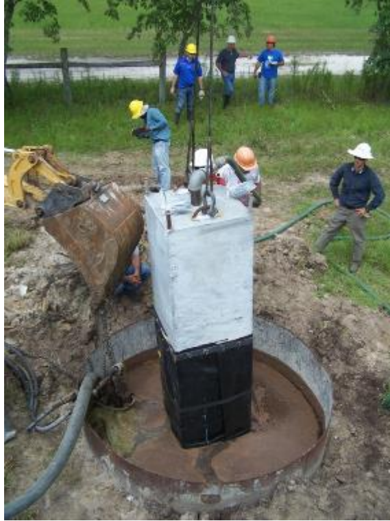
Figure 10-1. Pile jetting
