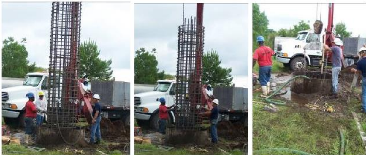
Figure 4-13. Setting rebar cage in the excavation
