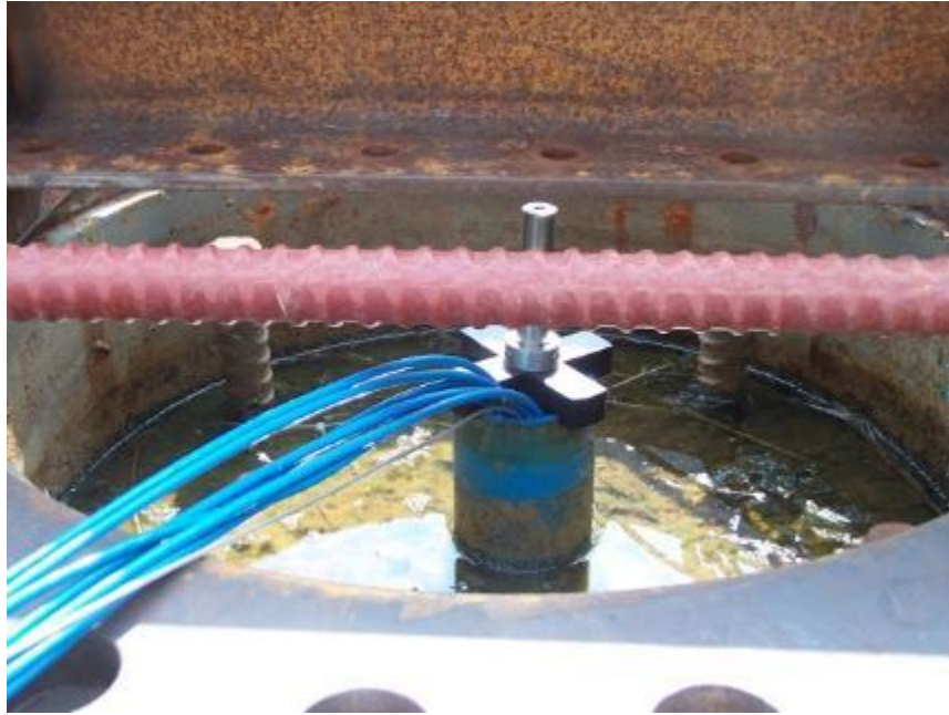
Figure 8-2. In-place inclinometer installation in the test shaft
