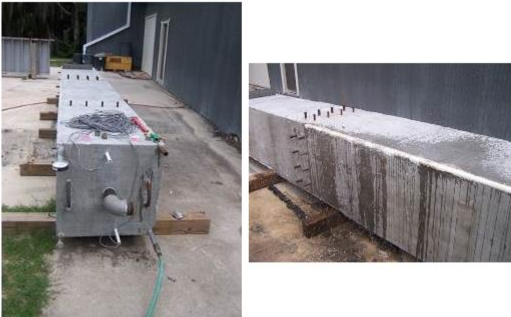
Figure 5-9. Flushing the grout delivery systems
