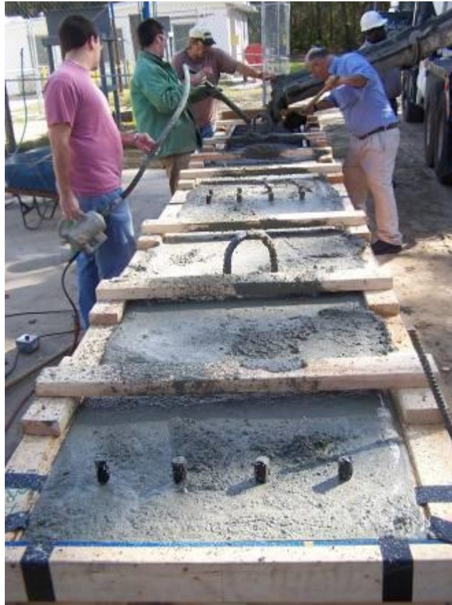
Figure 5-8. Concrete placement
