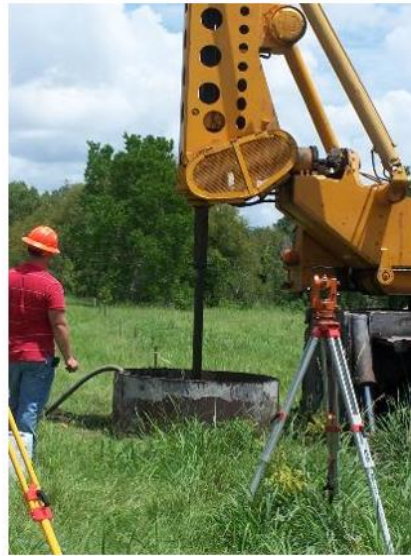
Figure 4-10. Excavating hole for drilled shaft construction
