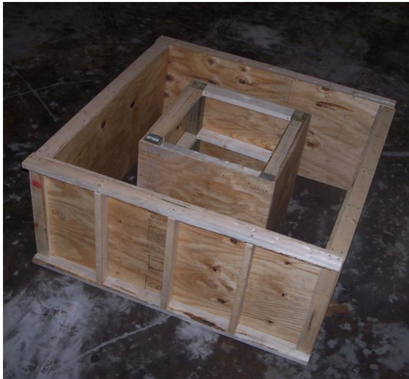
Figure 5-22. Formwork for concrete cap
