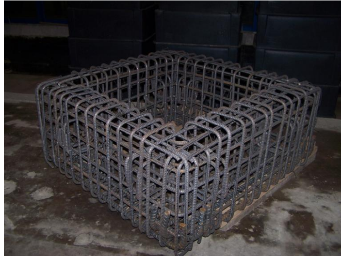
Figure 5-23.: Reinforcement cage for concrete cap
