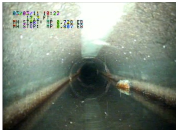
Figure 4-3. Screenshot from pipe inspection video of Site #000, showing inside of the pipe.
