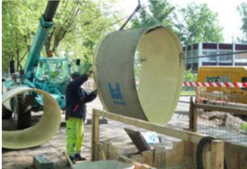
Figure 2-12. Pipe rehabilitation by paneling (TI 2009).
