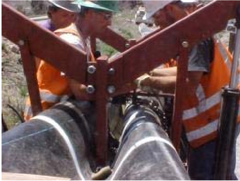
Figure 2-15. Liner being mechanically deformed prior to installation (Caltrans 2003b).
