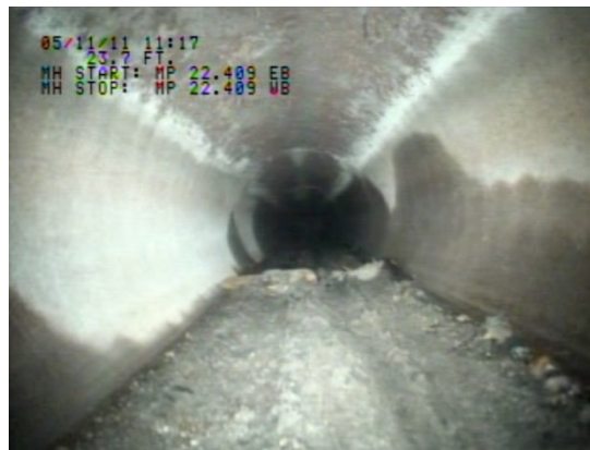
Figure 4-37. Screenshot from pipe inspection video of Site #011, showing the inside of the pipe.
