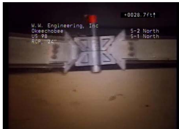
Figure 4-46. Screenshot from pipe inspection video of Site #005, showing a joint which has been repaired using an NPC Internal Joint Seal.
