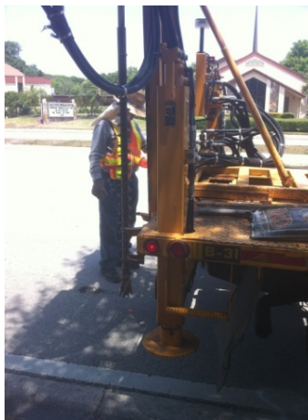
Figure 3-3. The crew from District 1 boring through roadway pavement to obtain a soil sample on top of the pipe in Indian River County.
