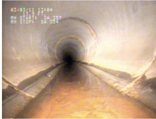
Figure 4-10. Screenshot from pipe inspection video of Site #002, showing the inside of the pipe.
