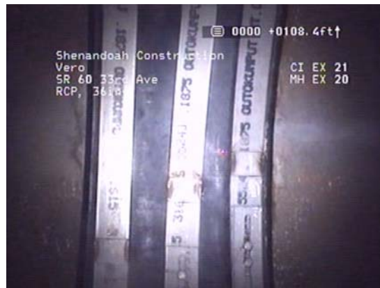
Figure 4-49. Screenshot from pipe inspection video of Site #005, showing a joint which has been repaired using a set of band seals.
