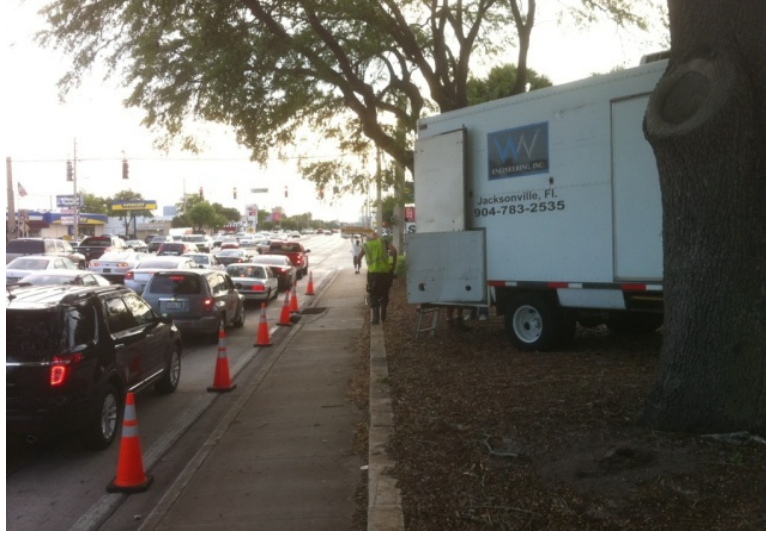
Figure 3-2. Pipe inspection crew from WW Engineering preparing to inspect a pipe connected to a curb and gutter system in an extremely urban area in Orange County.
