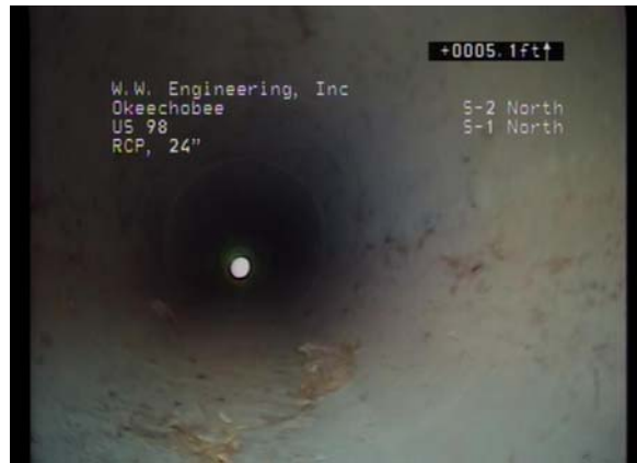
Figure 4-47. Screenshot from pipe inspection video of Site #013, showing the inside of the pipe.
