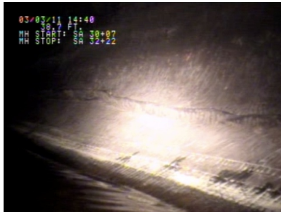
Figure 4-23. Screenshot from pipe inspection video of Site #005, showing the pipe liner.
