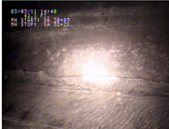
Figure 4-25. Screenshot from pipe inspection video of Site #005, showing the pipe liner and the wrinkle.
