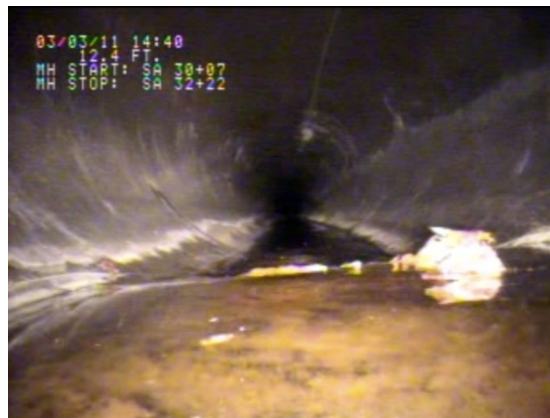
Figure 4-24. Screenshot from pipe inspection video of Site #006, showing the inside of the pipe.
