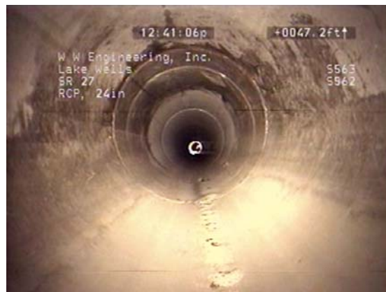
Figure 4-44. Screenshot from pipe inspection video of Site #015, showing the inside of the pipe.
