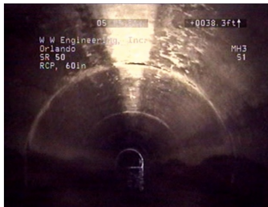
Figure 4-15. Screenshot from pipe inspection video of Site #004, showing the inside of the pipe.
