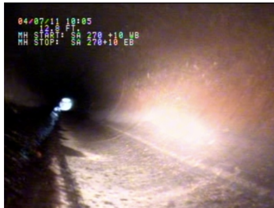
Figure 4-29. Screenshot from pipe inspection video of Site #009, showing the inside of the pipe and the pipe liner placed along the entire run of the pipe.
