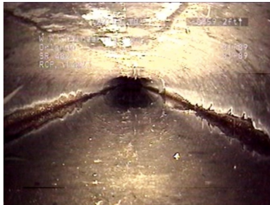
Figure 4-27. Screenshot from pipe inspection video of Site #008, showing the inside of the pipe and the pipe liner.
