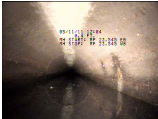
Figure 4-40. Screenshot from pipe inspection video of Site #012, showing the inside of the pipe.
