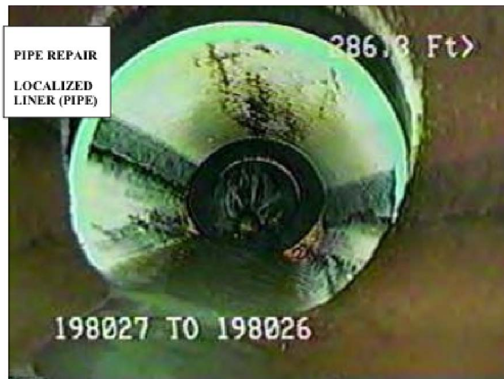
Original pipe section(s) repaired using localized liner.
