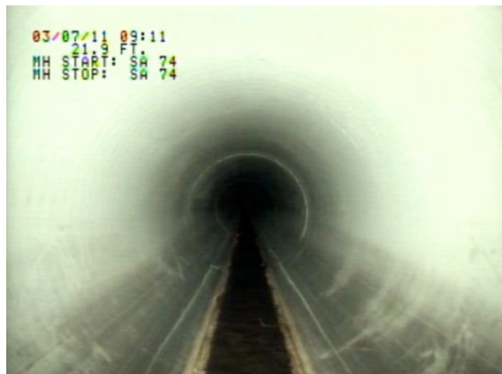
Figure 4-20. Screenshot from pipe inspection video of Site #005, showing the inside of the pipe.
