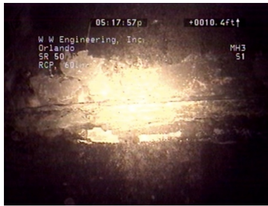
Figure 4-17. Screenshot from pipe inspection video of Site #004, showing a joint which has been repaired with chemical grout. The joint is completely sealed with grout.
