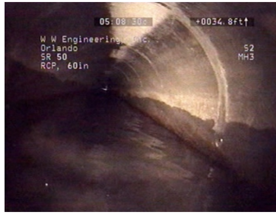
Figure 4-14. Screenshot from pipe inspection video of Site #003, showing the inside of the pipe.
