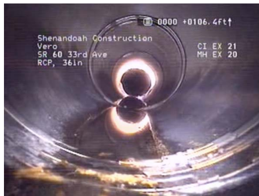
Figure 4-50. Screenshot from pipe inspection video of Site #014, showing the inside of the pipe.
