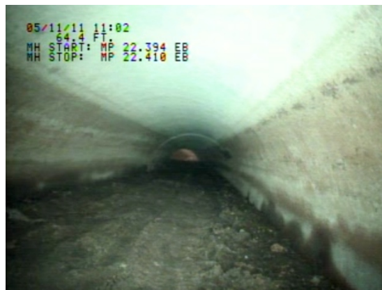
Figure 4-34. Screenshot from pipe inspection video of Site #010, showing the inside of the pipe.
