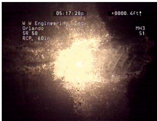
Figure 4-16. Screenshot from pipe inspection video of Site #004, showing a close up of a joint which has been repaired with chemical grout. The joint is completely sealed with grout.
