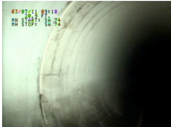
Figure 4-21. Screenshot from pipe inspection video of Site #005, showing a joint of the pipe liner.
