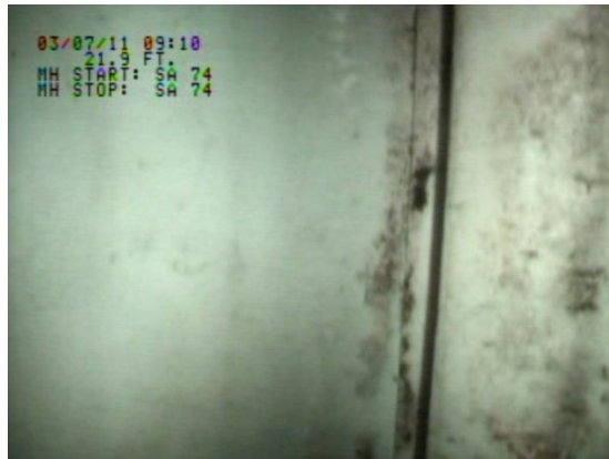
Figure 4-19. Screenshot from pipe inspection video of Site #005, showing a joint of the pipe liner.
