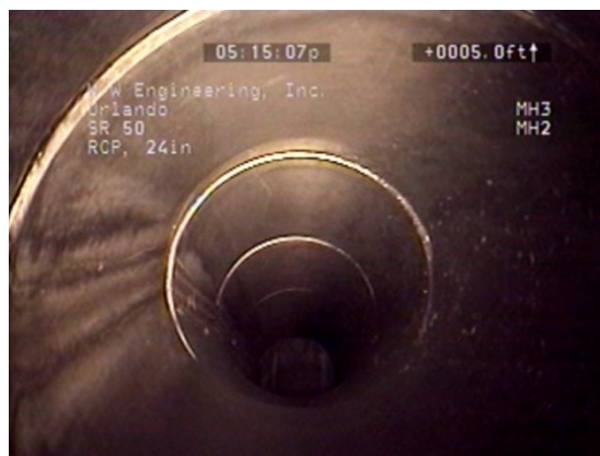
Figure 4-31. Screenshot from pipe inspection video of Site #007, showing the inside of the pipe and the sectional liner placed from joint to joint.
