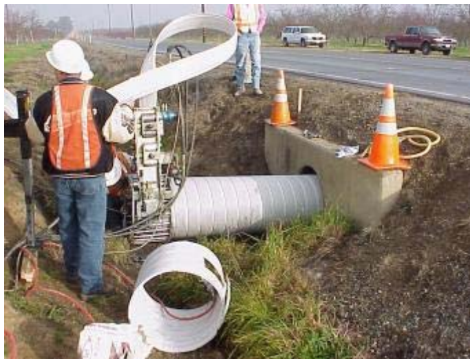
Figure 2-11. Liner installation by spiral wound method (Caltrans 2003b).
