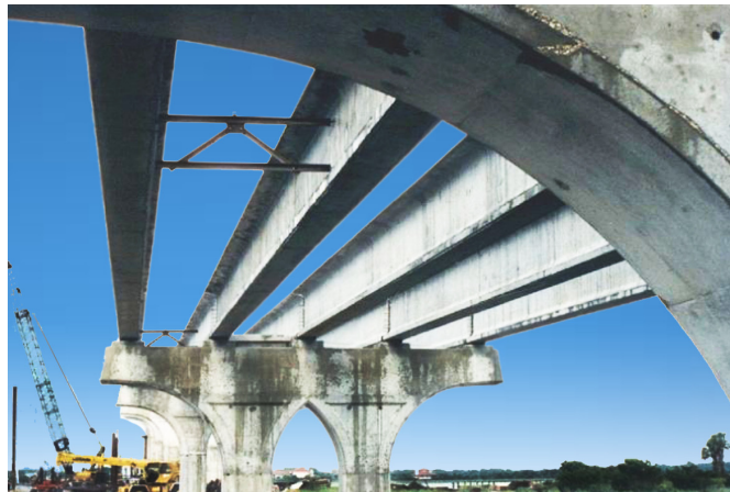
Cross-bracing between bridge girders.
