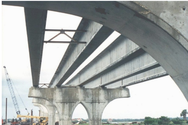
Figure 1.1 Prestressed concrete girders braced together for stability
