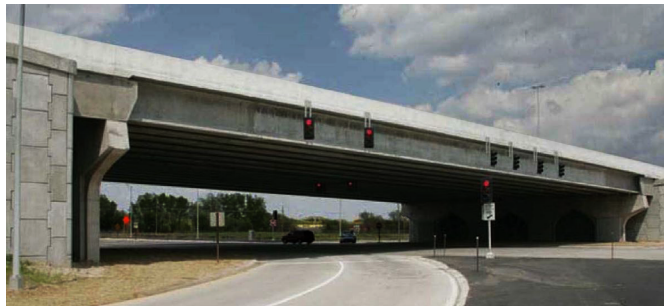
This bridge in Nebraska uses 207-ft spliced girders, similar to the type explored in this project.
