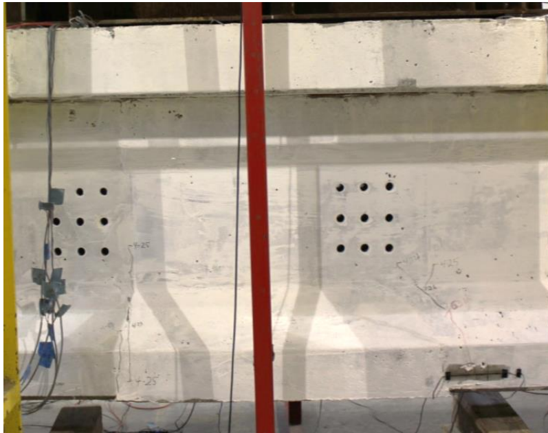
Figure 173–F2: Cracking after 2 million cycles
