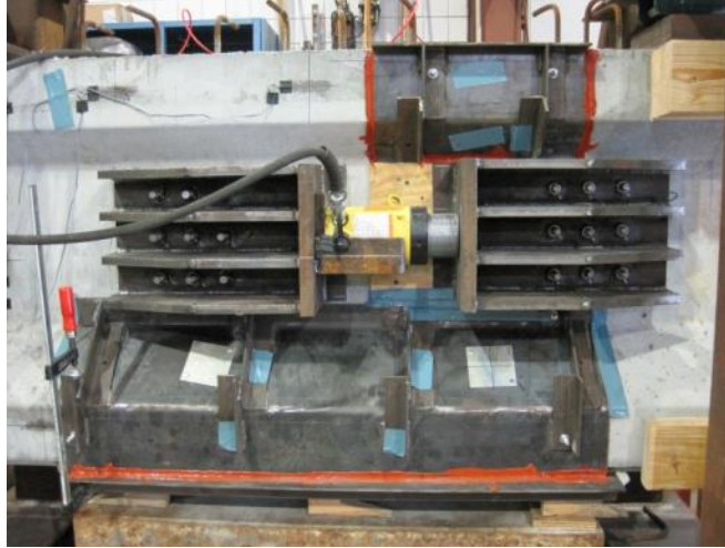
Figure 56—Closure formwork in place
