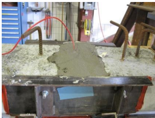
Figure 59–Top of finished closure pour
