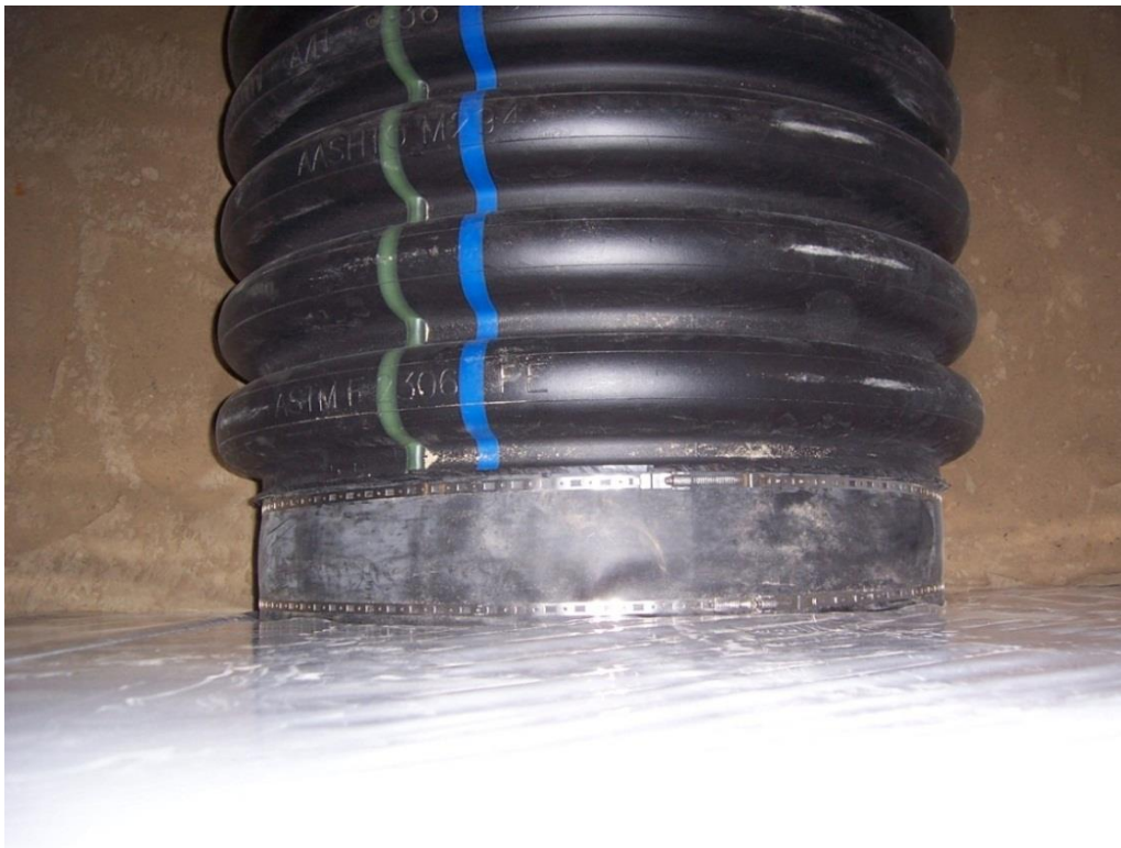
Figure 3-4. Installed flexible membrane system.
