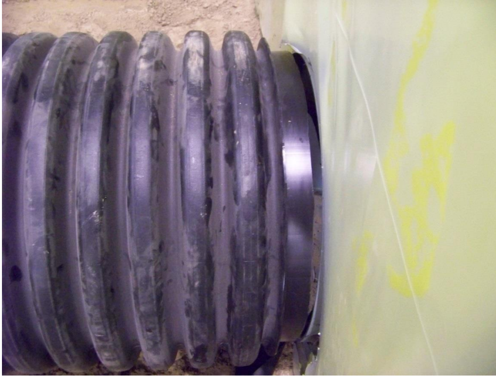
Figure 5-7. Properly positioned pipe before flexible membrane system installation.
