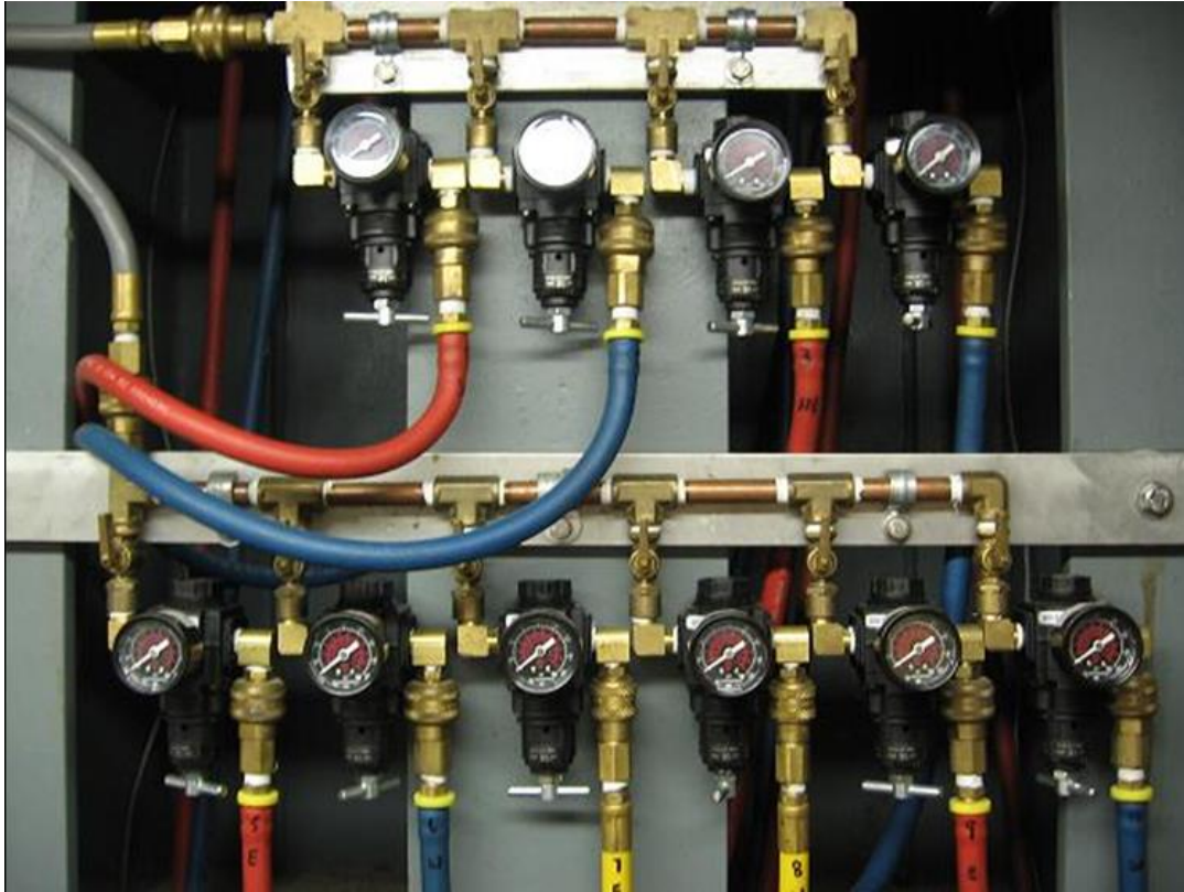
Figure 7-3. Regulators used to control lift bag pressure over individual load plates.
