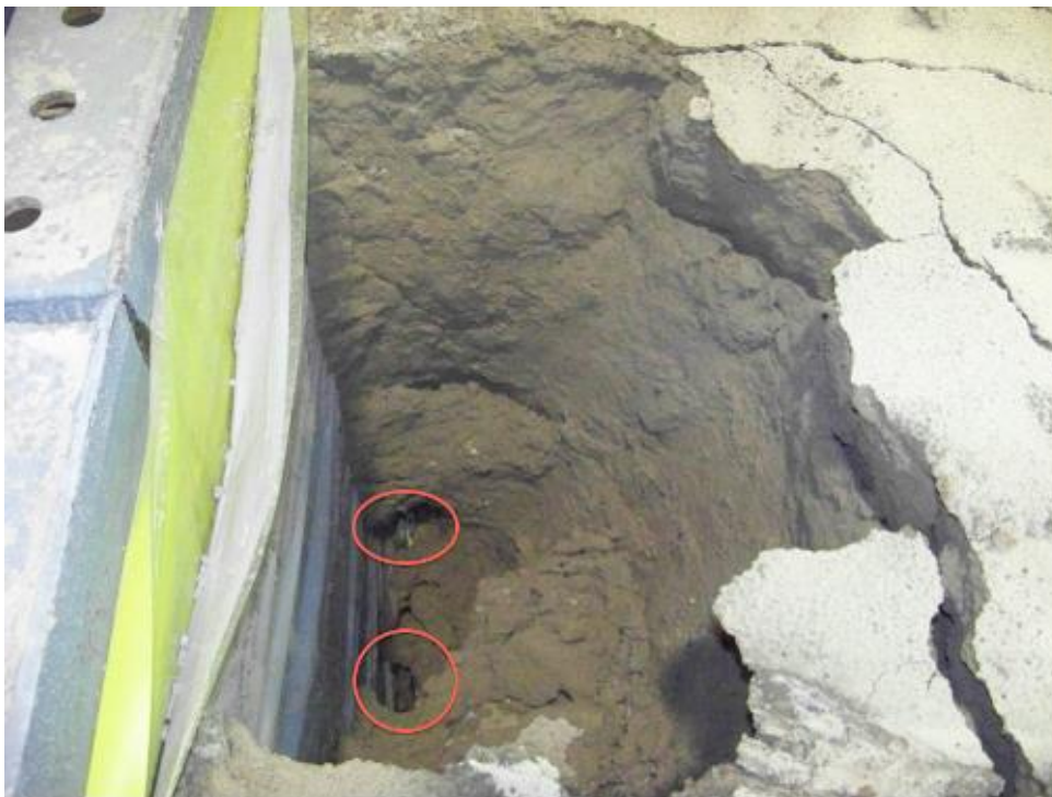
Figure 9-11. Top view of void (circle showing HDPE pipe)
