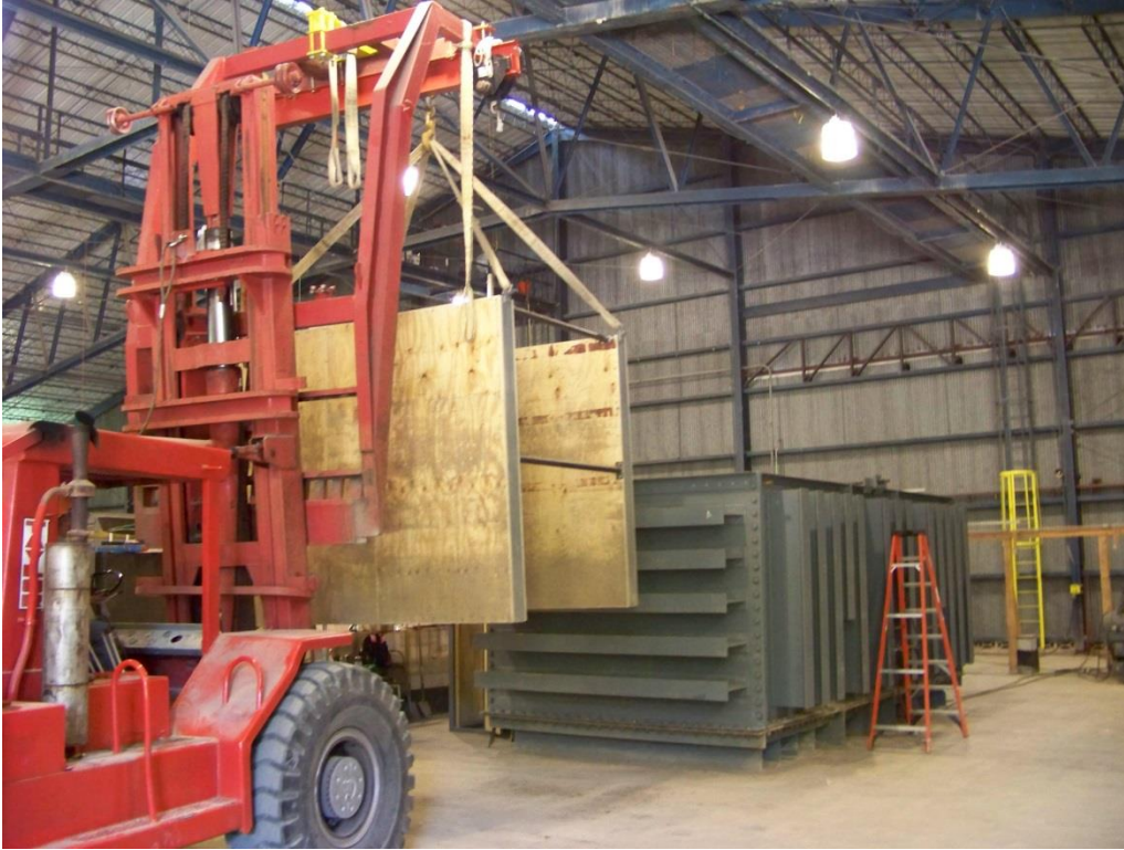
Figure 8-7. Hoisting trench box into Soil Box.
