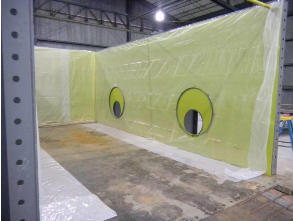
Figure 2-19. Two layers of lubricated polyethylene sheets.
