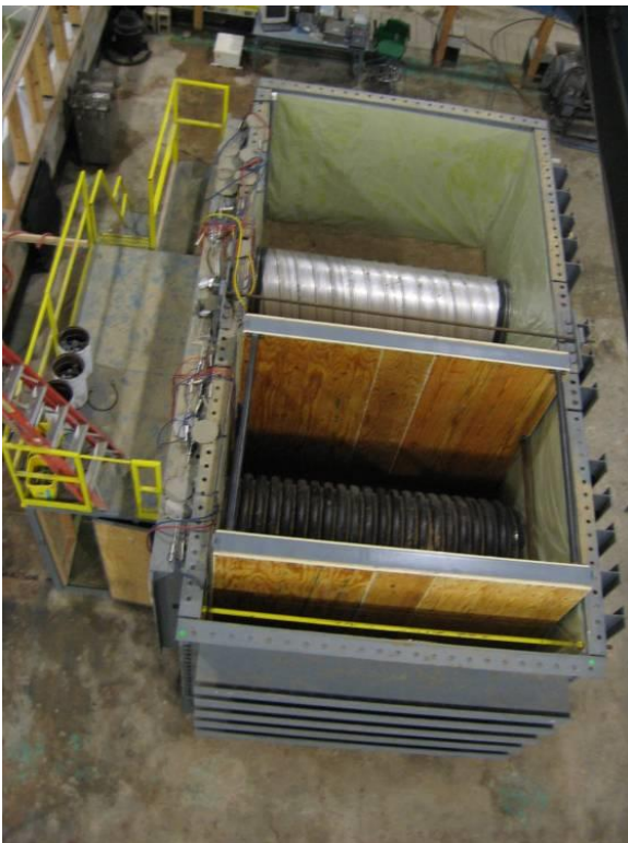
Figure 8-8. Installed trench box.
