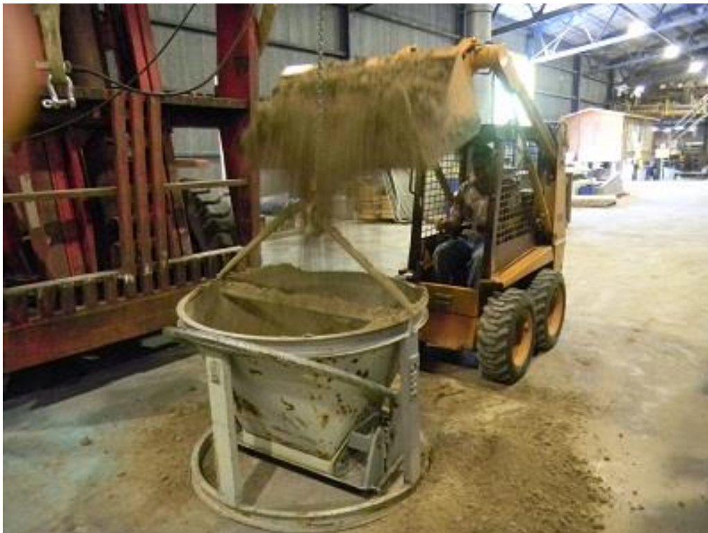
Figure 5-10. Filling concrete bucket with front end loader.
