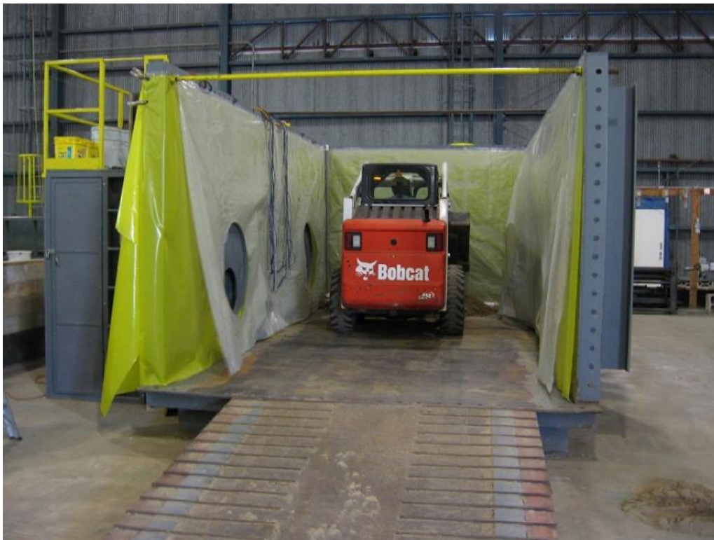
Figure 5-4. Soil being placed with front end loader.
