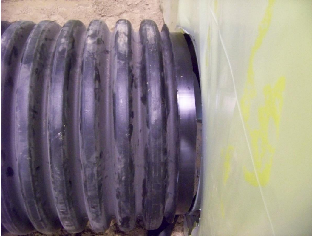
Figure 10-8. Shaved corrugation on HDPE pipe prior to flexible membrane installation
