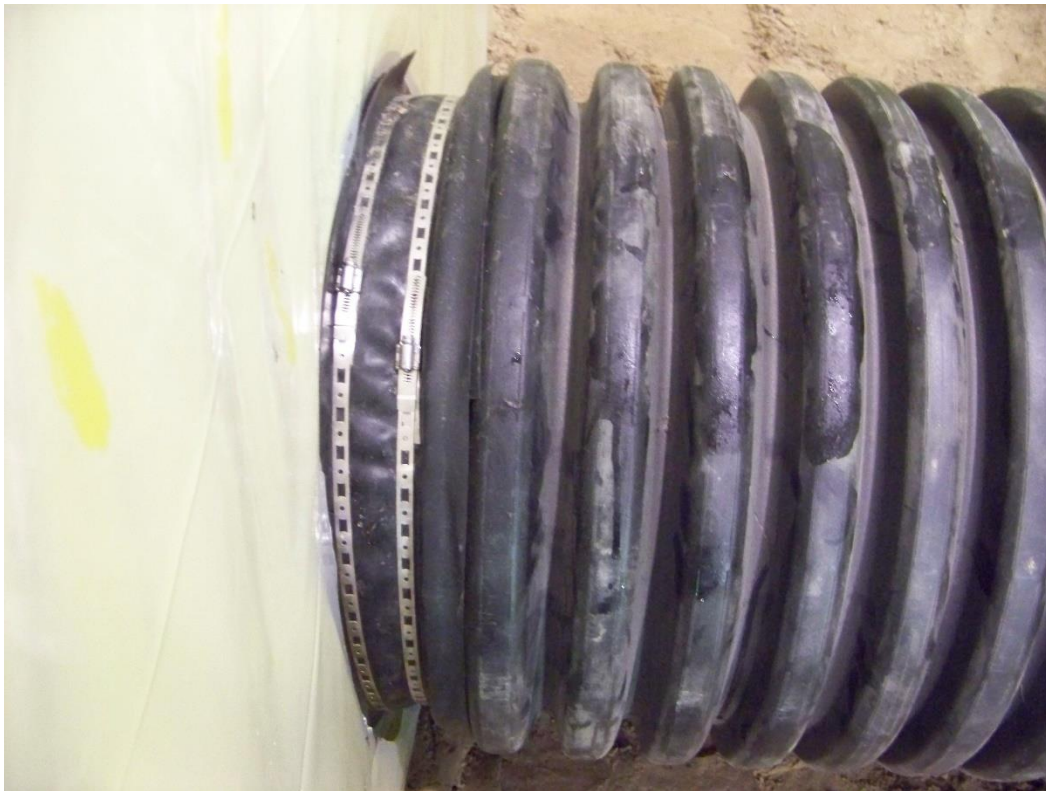
Figure 10-9. Installed flexible membrane system
