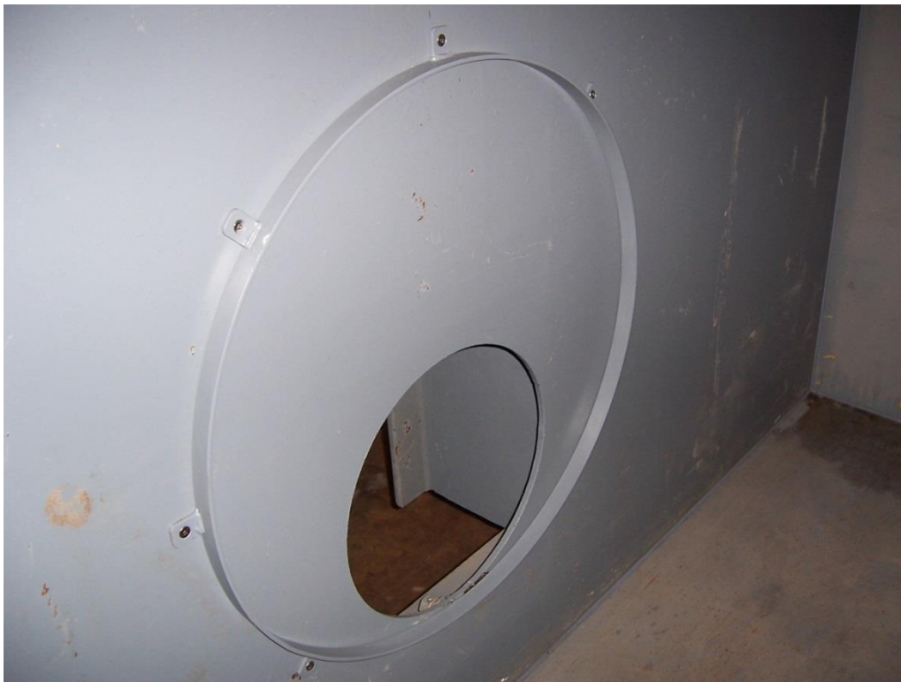
Figure 3-2. Rigid steel angle, part of the flexible membrane system.
