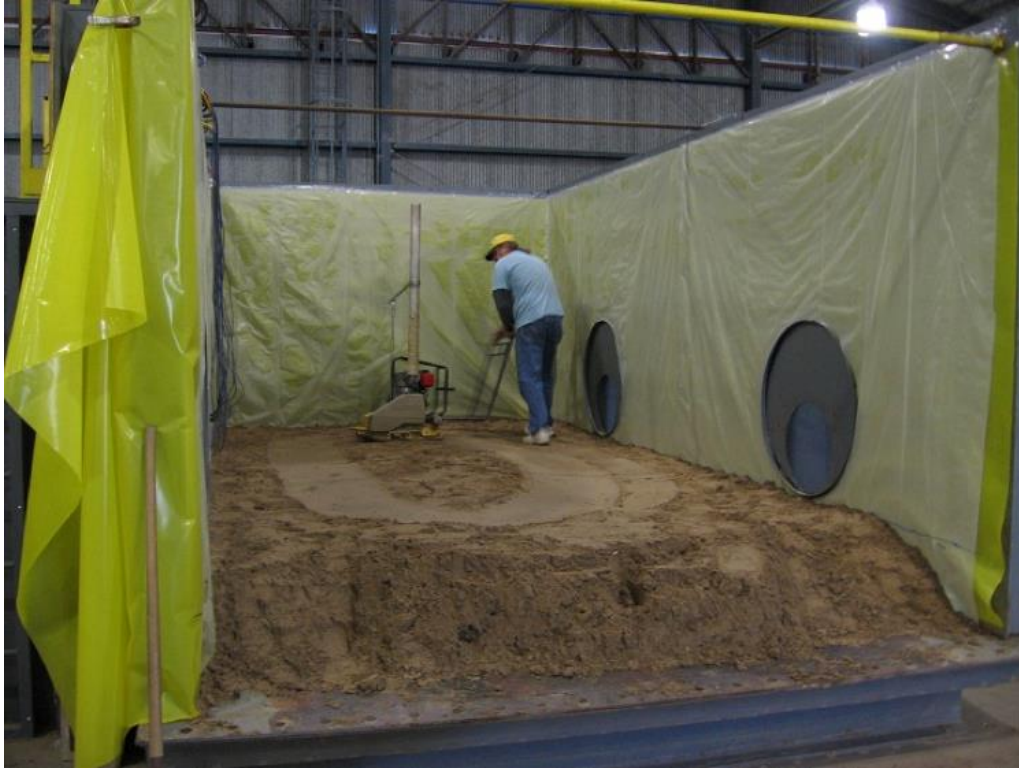
Figure 5-5. First lift during compaction.
