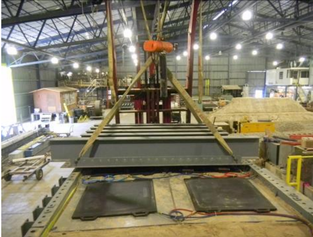
Figure 5-13. Top partition hoisted onto Soil Box via lift truck.
