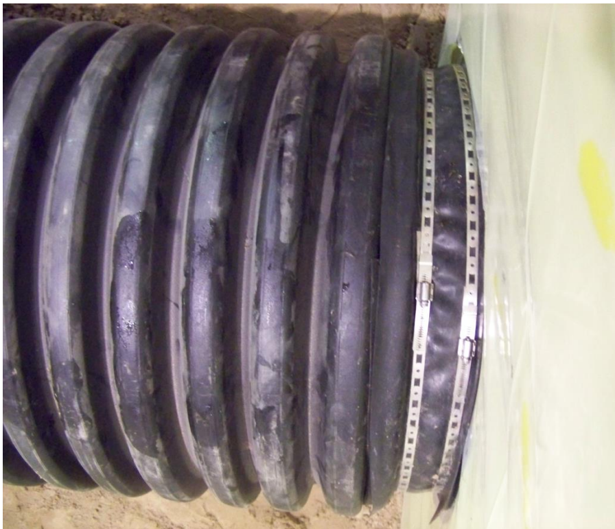
Figure 5-8. Installed flexible membrane system.
