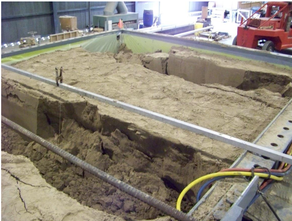
Figure 8-10. Installed trench box.
