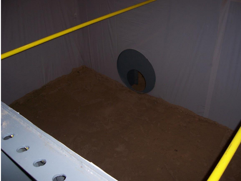
Figure 3-3. 12 inch thick layer of compacted soil.
