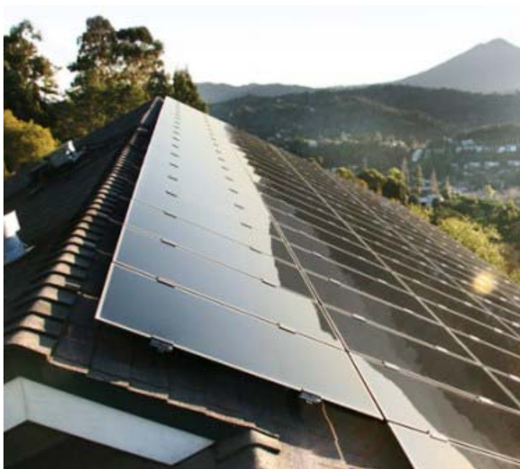
Figure 2.10 Thin film PV module: cadmium telluride (CdTe) type (Courtesy: http://www.pv-tech.org/images/uploads/solarcity/solarcity_fslrmodules.jpg )
