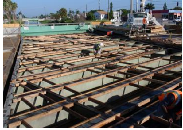
Figure 11 – Formwork for grout pads
