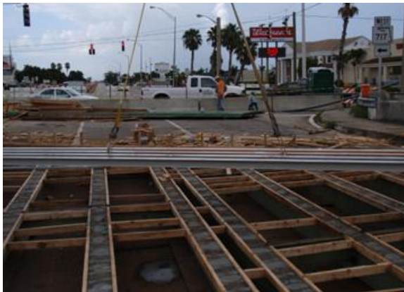
Figure 12 – Installation of bottom GFRP panels
