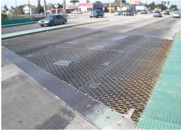
Figure 10 – Existing steel grid deck
