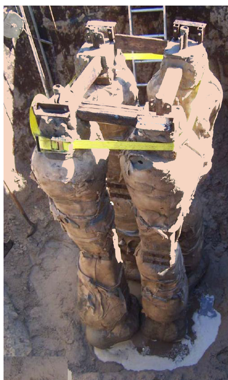
A freshly excavated group of jet-grouted piles is readied for removal from the test chamber after testing.
