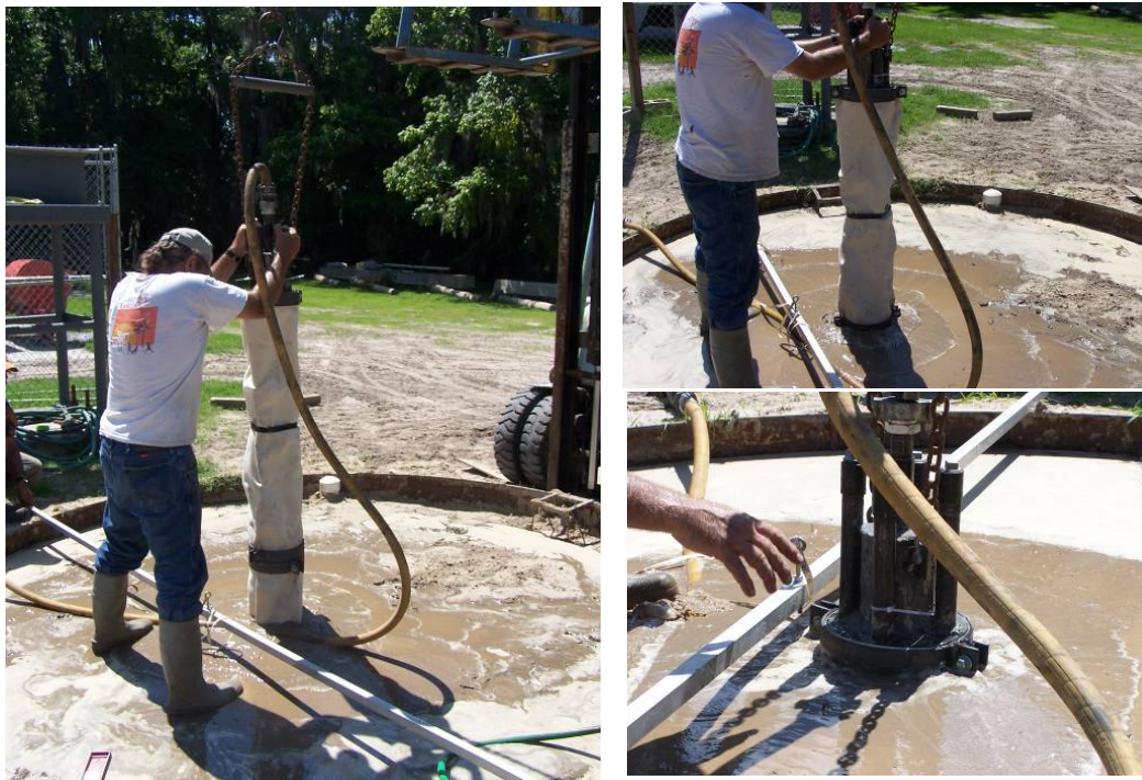
Figure 4-63 Pile jetting.
