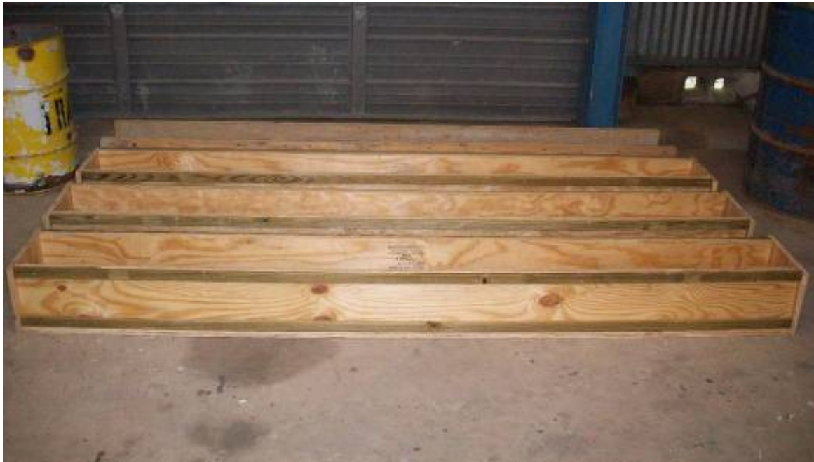
Figure 4-3 Formwork for casting piles.
