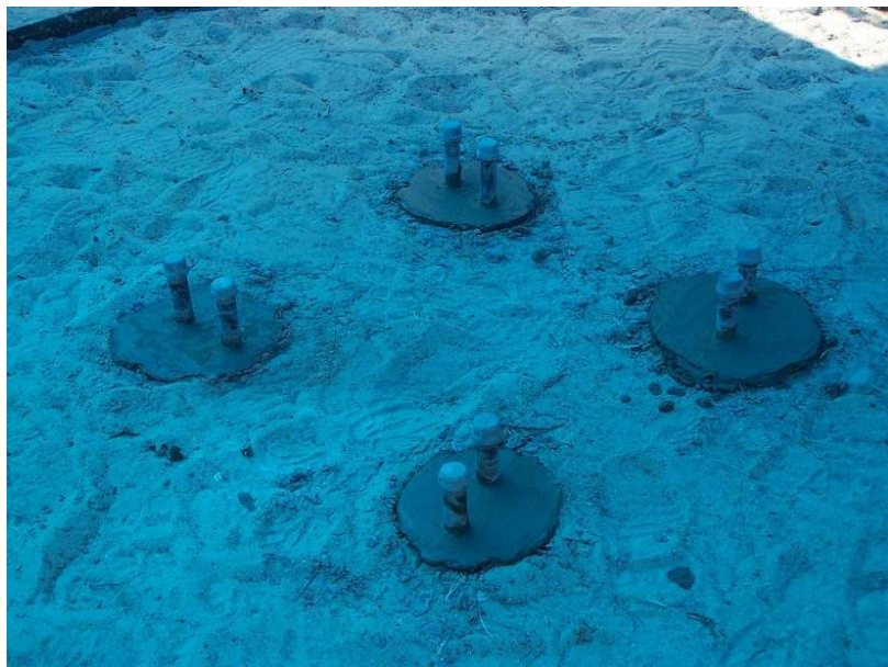
Figure 5-8 Drilled shafts.
