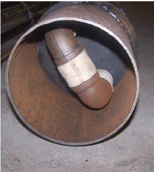
Figure 5-35 Grout exit and membrane covering.
