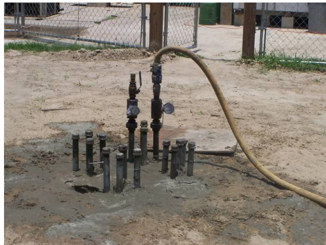
Figure 4-64 Side grouting.
