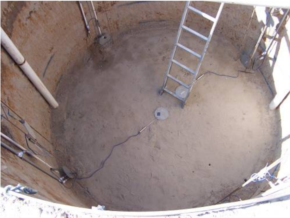
Figure 4-14 Stress gages placed horizontally at 10-ft. depth.
