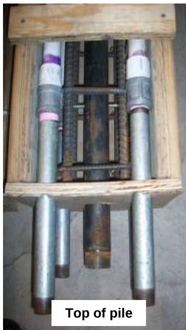
Figure 4-5 Rebar cage, jetting pipe, and grouting systems positioned in the formwork.
