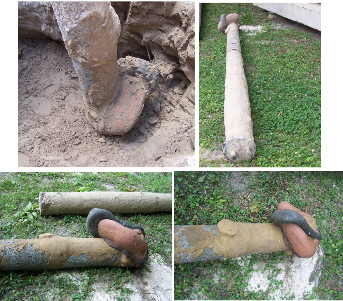
Figure 5-44 Grout zone–North shaft.
