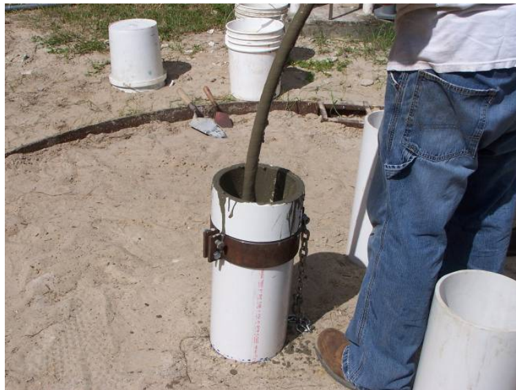
Figure 5-6 Concrete vibrated with a wand.
