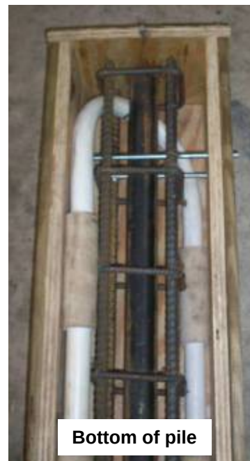
Figure 4-5 Rebar cage, jetting pipe, and grouting systems positioned in the formwork.
