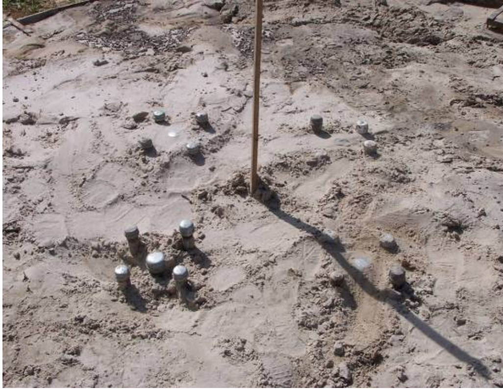
Figure 4-19. Piles jettied into the ground.
