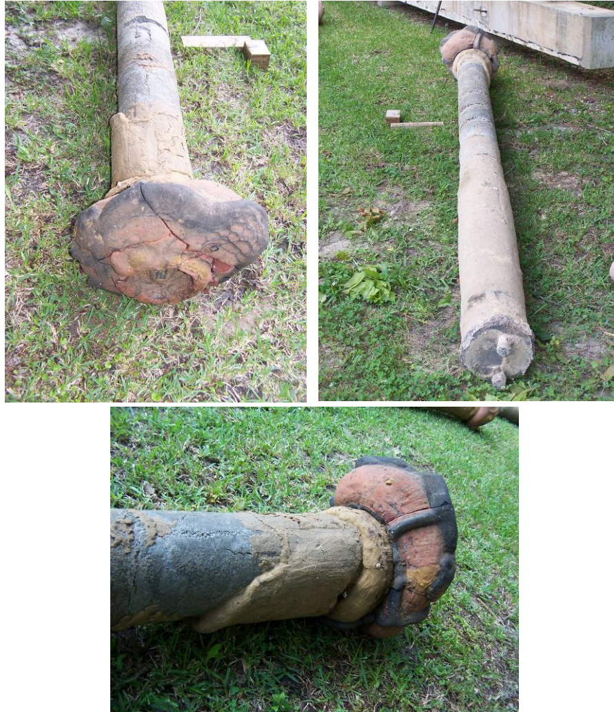
Figure 5-45 Grout zone–West shaft.
