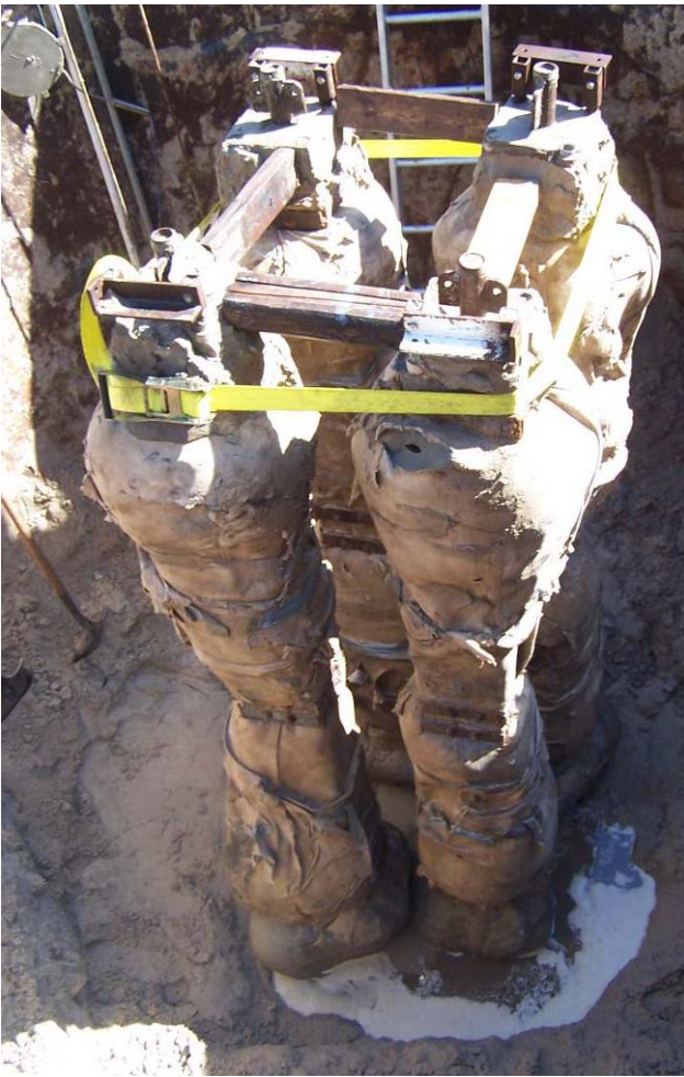
Figure 4-33 Exposed pile group.
