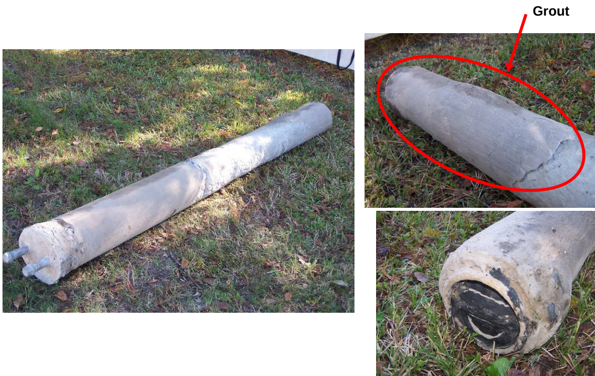
Figure 7-9 Grout-tipped drilled shaft after excavation.
