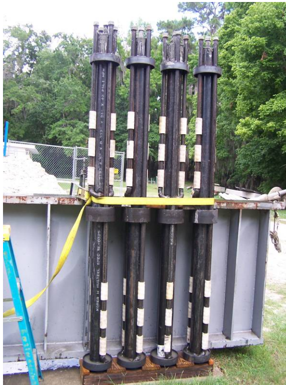
Figure 4-59 Piles after pouring concrete.
