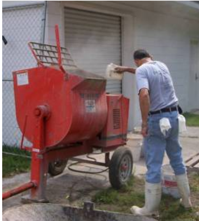
Figure 4-20 Grout mixing using mortar mixer.
