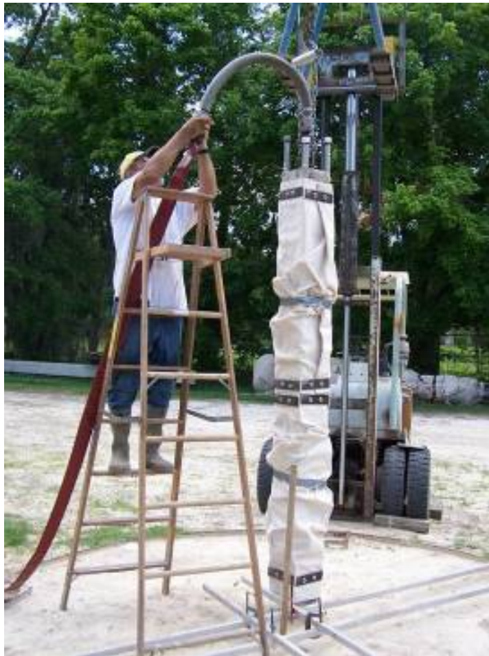
Figure 4-17 Pile prior to jetting.
