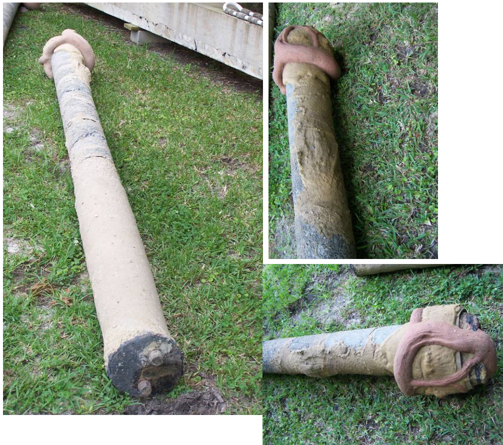
Figure 5-43 Grout zone–South shaft.
