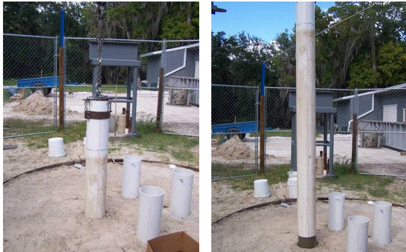
Figure 5-7 Pulling the casing out.
