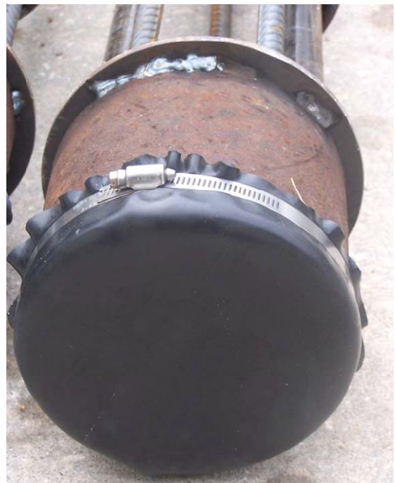
Figure 5-35 Grout exit and membrane covering.
