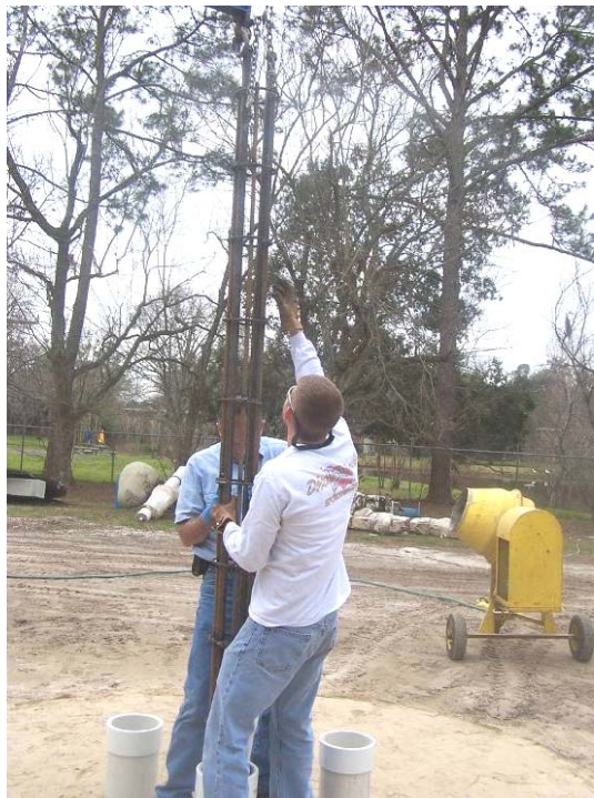
Figure 5-38 Lowering the rebar cage into PVC casing.
