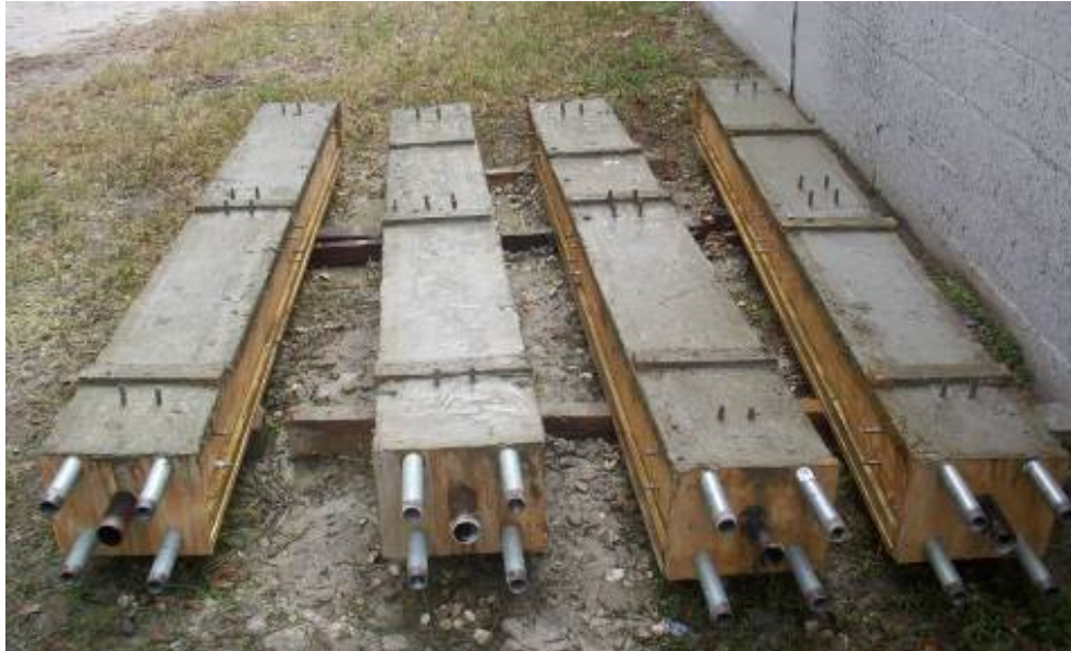
Figure 4-6 Piles with formwork (after pouring concrete).
