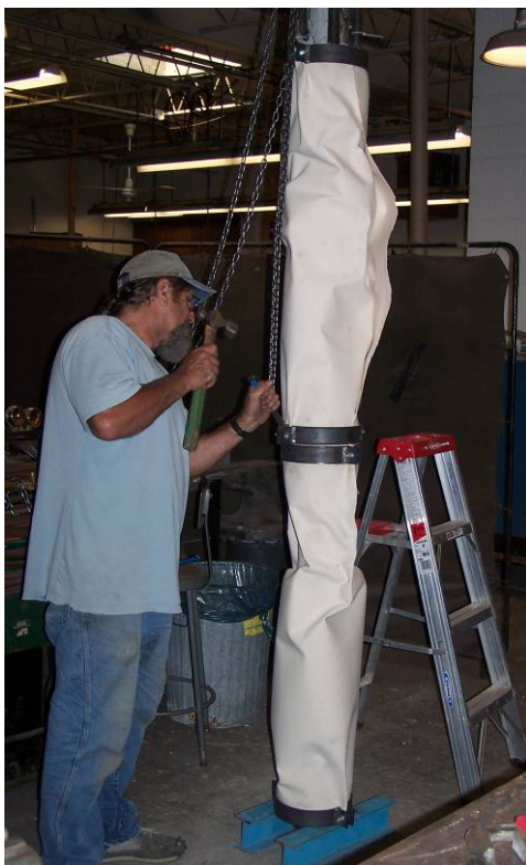
Figure 4-60 Attachment of semi-rigid membrane to pile.
