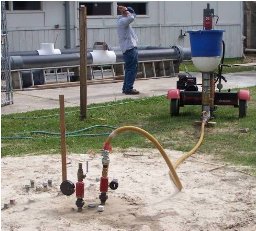
Figure 4-22 The 1.5-inch high pressure line connected from the grout pump to the pile.
