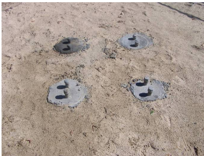
Figure 5-39 Drilled shaft group after concreting.
