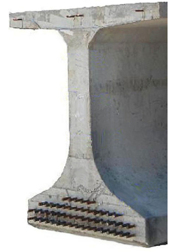
Left: close-up of pretensioning strands and reinforcing bar in the Florida I-Beam (FIB) form before concrete is added. Right: end view of the FIB.
