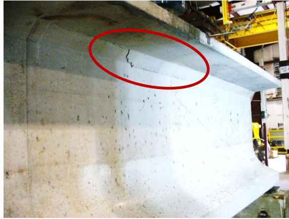
Figure 76–Punching shear failure in specimen SL
