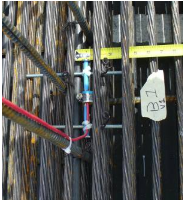
Figure 37—V gage installation (view from above)
