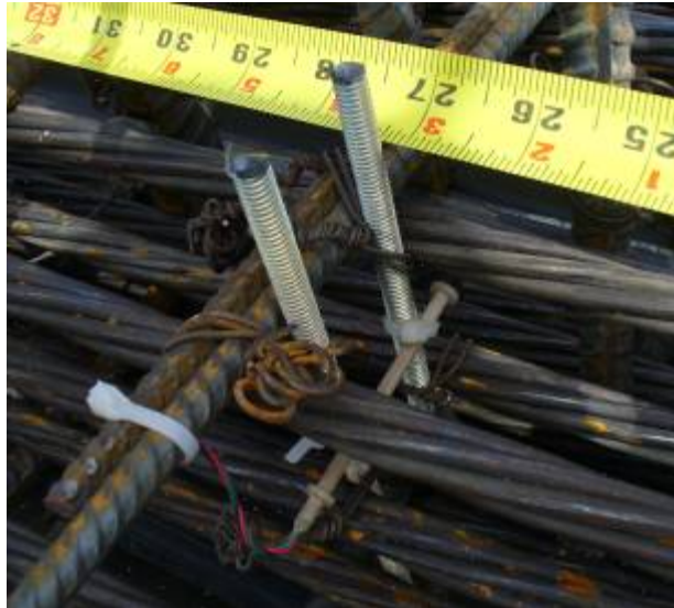
Figure 36—ES gage installation
