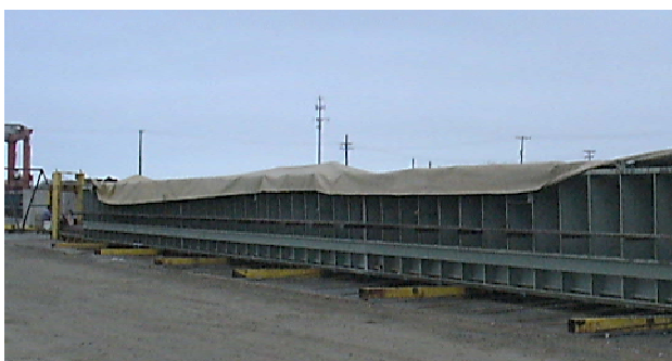
Figure 23–Top flange finish (left) and tarp covers (right)
