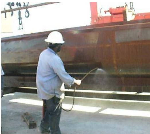
Figure 21–Form release application (left) and form cross-ties (right)
