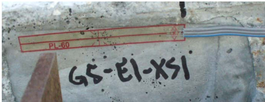
Figure 35—XS gage installation
