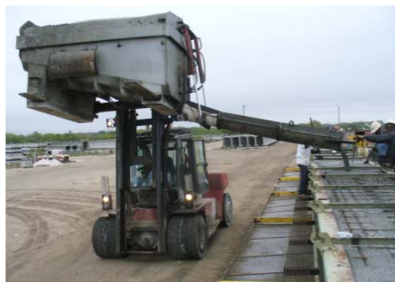
Figure 22–Concrete delivery (left) and placement (right)
