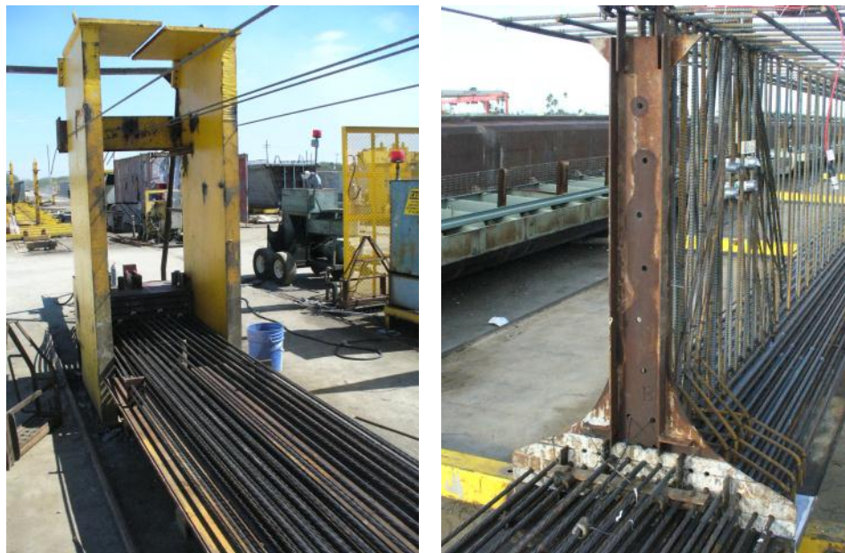
Figure 12–Jacking frame (left), and steel bulkhead (right).
