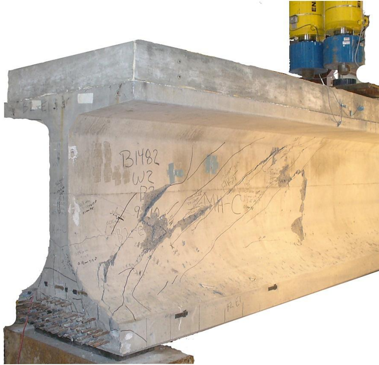
Figure 94–VC after load test
