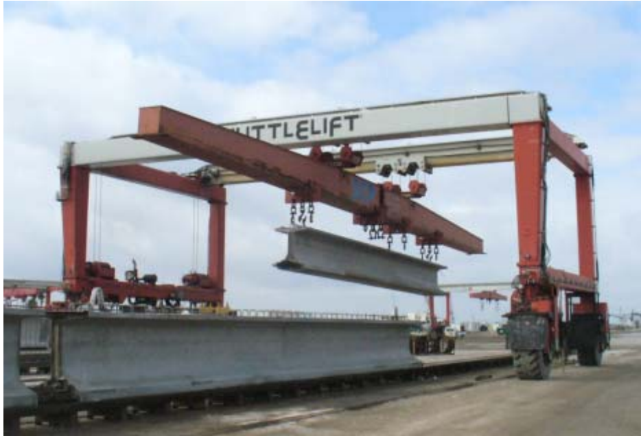
Figure 29–Test girder lifted by crane
