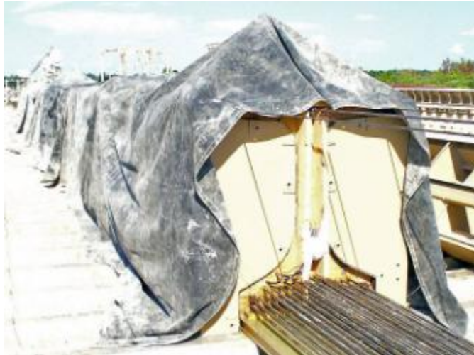
Figure 27–Girders covered with tarps
