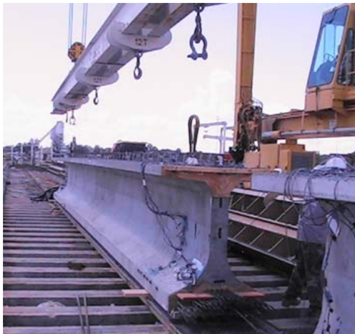
Figure 30–Girder resting on dunnage above stressing bed
