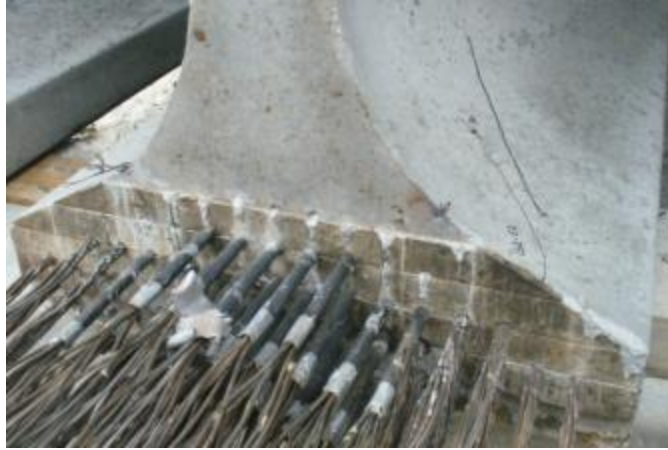
Figure 76—End of bottom flange covered by portion of steel bulkhead
