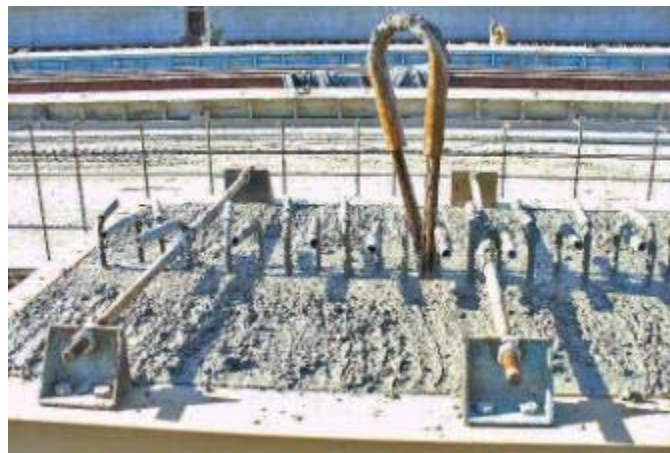
Figure 26—Girder finished surface
