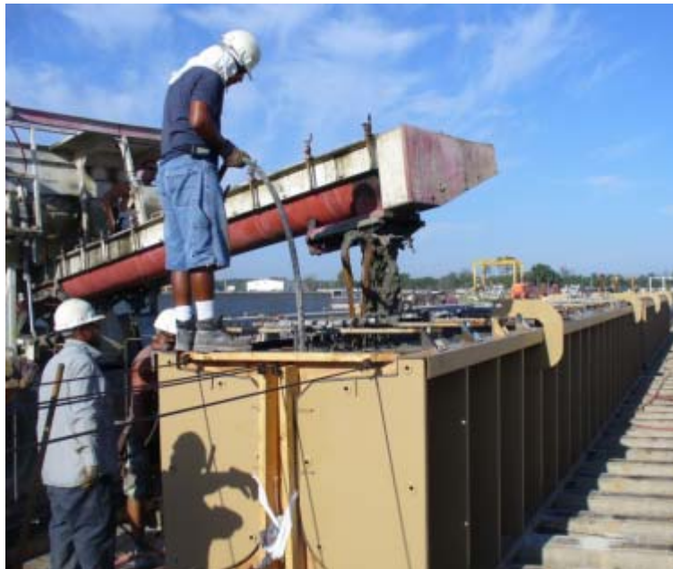
Figure 24–Concrete placement and internal consolidation phase 1
