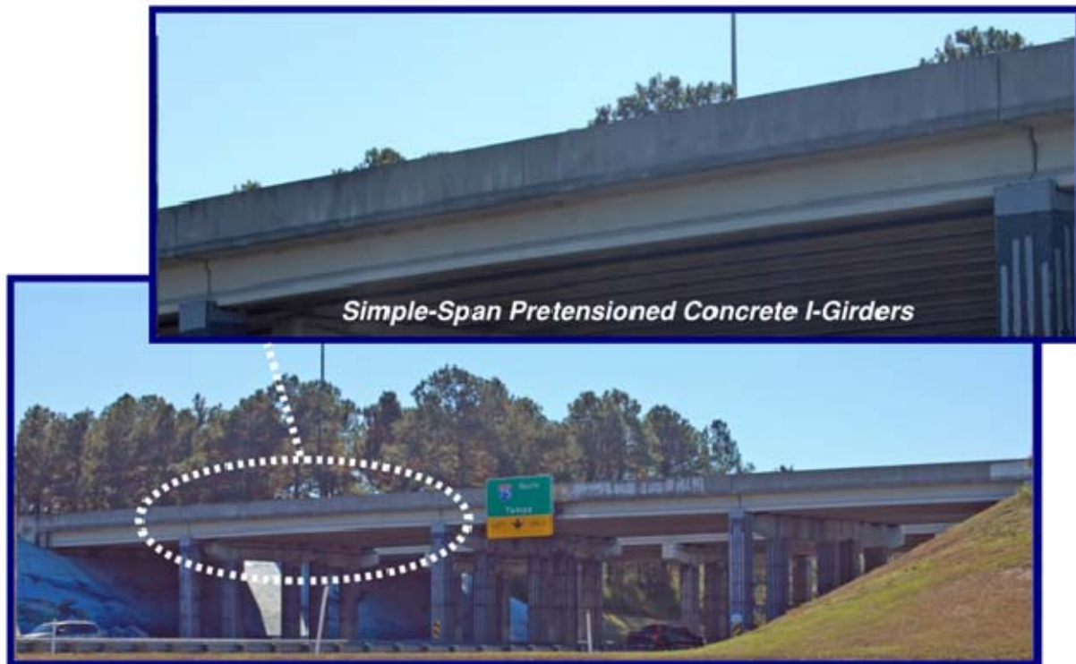
Figure 1—I-Girder highway bridge
