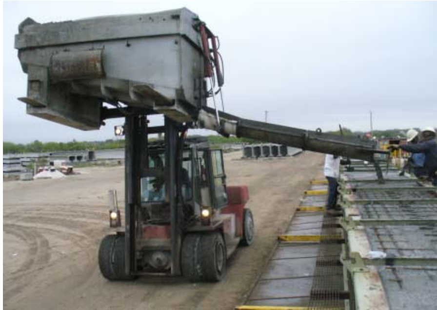
Figure 25—Concrete placement phase 2
