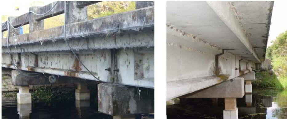
Figure 1—Existing bridge prior to girder removal
