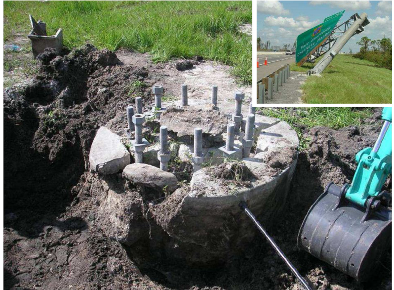
Partially excavated foundation showing concrete breakout that leads to collapse of the sign structure (inset, upper right).
