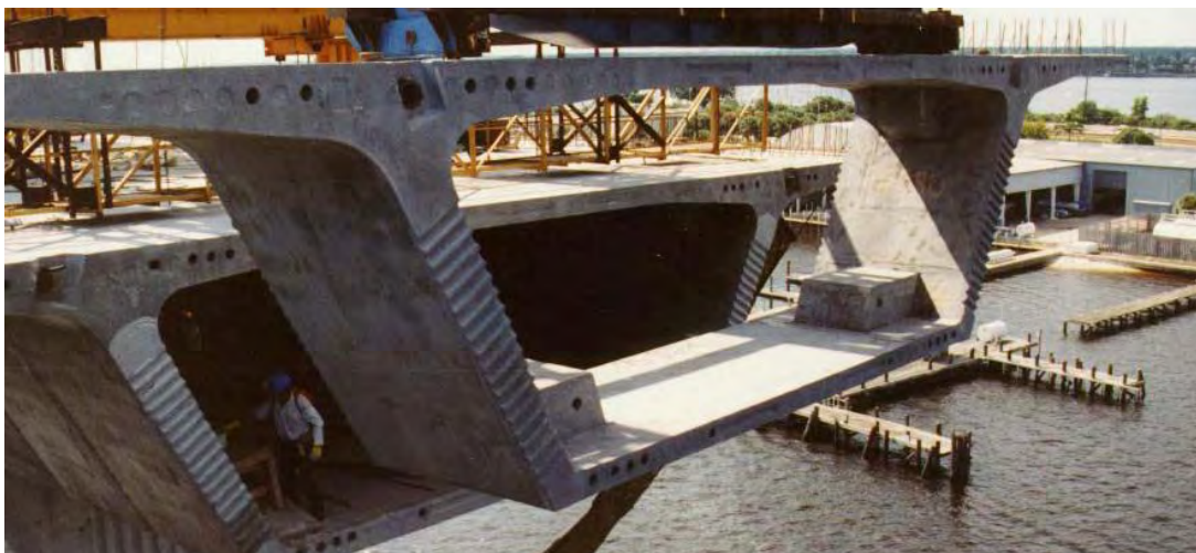
Figure 1-2: Segmental Box Girders
