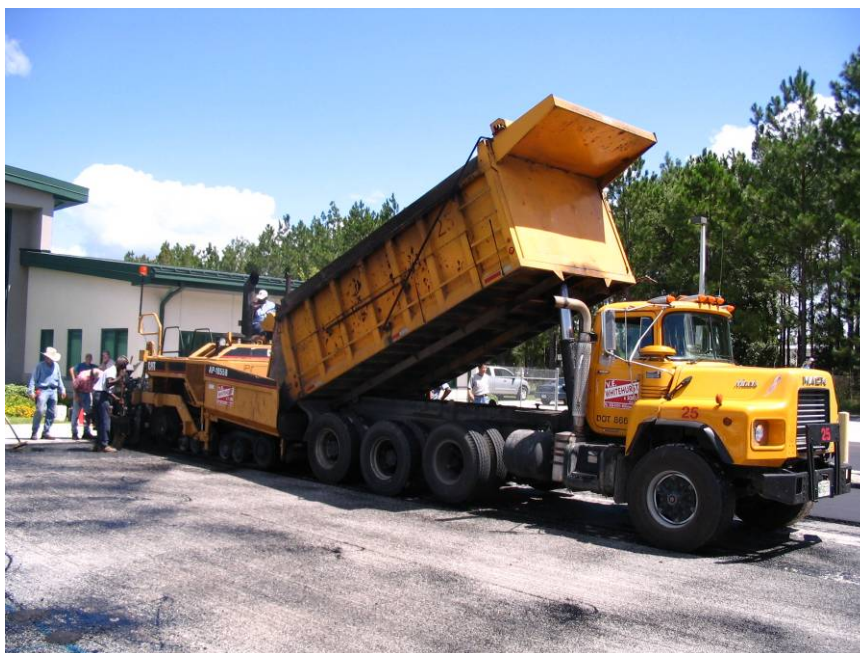
Figure 4-9. Paving operations
