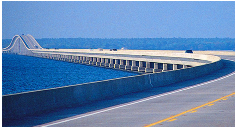
Building bridges like the 3.6-mile-long Mid-Bay Bridge in Okaloosa County depends on the design flexibility offered by post-tensioning technology.
