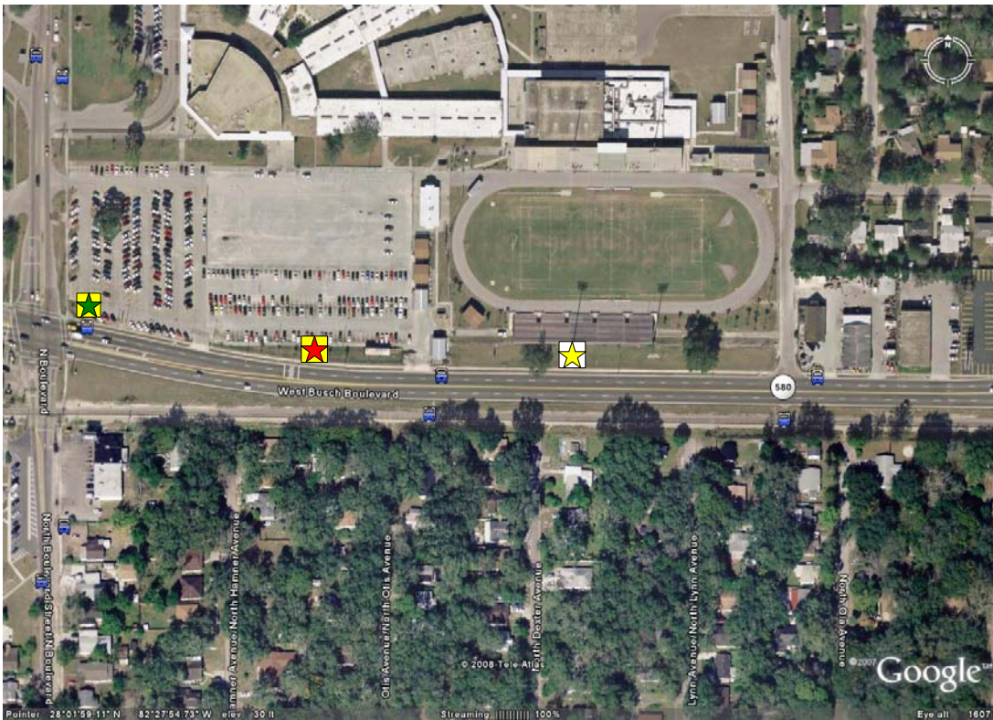
Route 39-West Busch Boulevard and N. Boulevard
