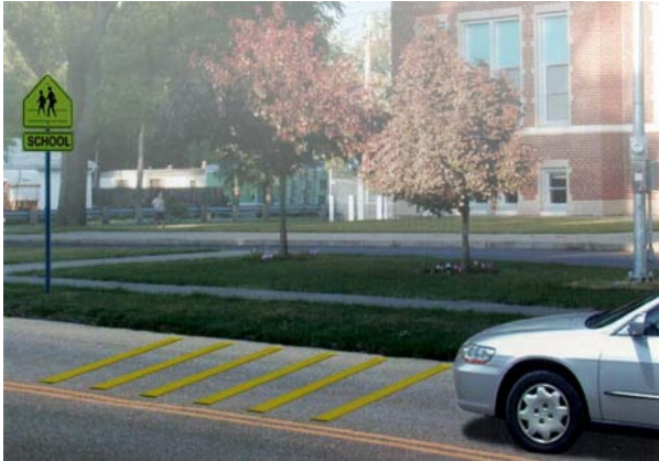
Figure 4-1: Rumble Strips Installation
