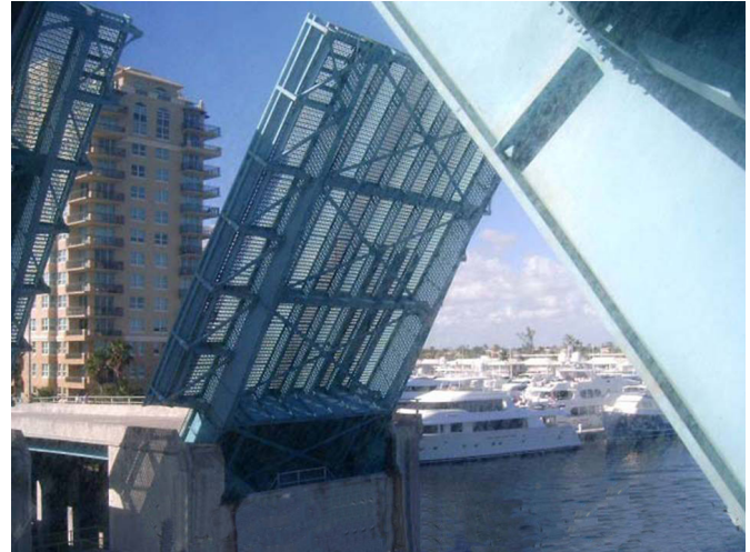
The Sunrise Boulevard Bridge, Ft. Lauderdale, Fla.
