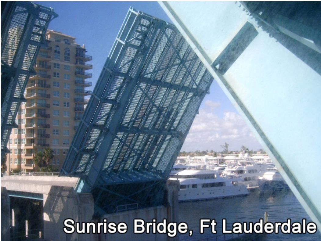
Figure 5.27 – Main girders in open position
