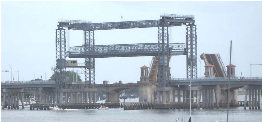
Figure 2.3 – Temporary bridge adjacent to the Bridge of Lions in open position (St. Augustine, FL)
