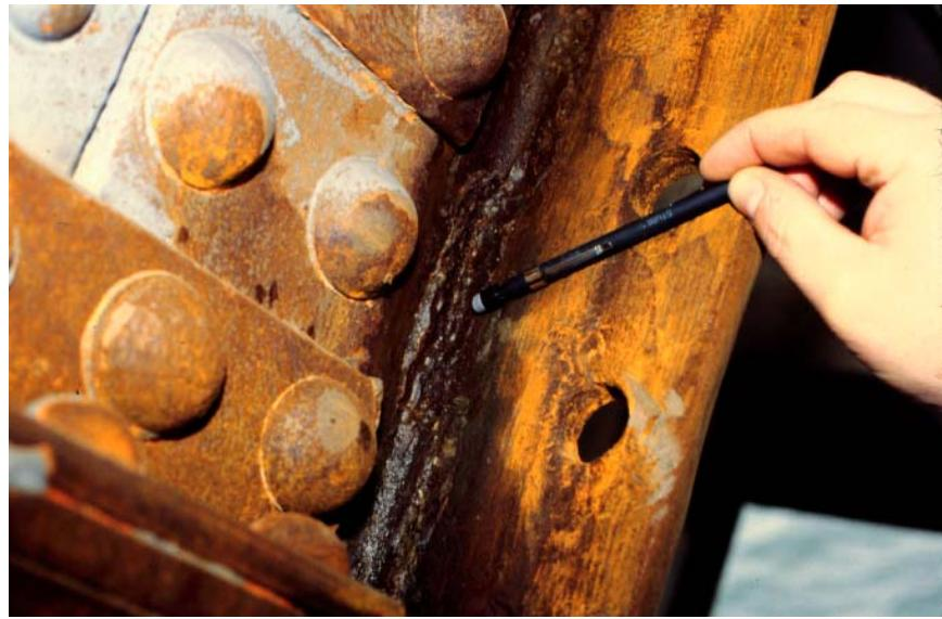
Figure 2.10 – Deterioration effects of corrosion on Michigan Street Bridge, Sturgeon Bay, Wisconsin
