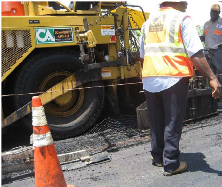
Figure 6.3: Pavetrac Mesh Curling under the Paver Tires
