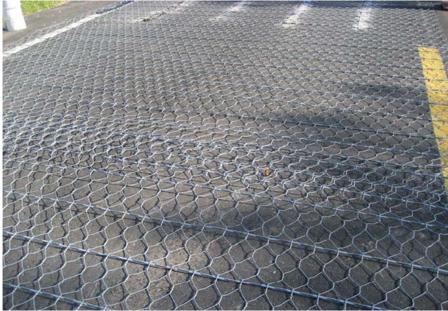
Figure 6.2: Pavetrac in Place, Showing a Transverse Overlap
