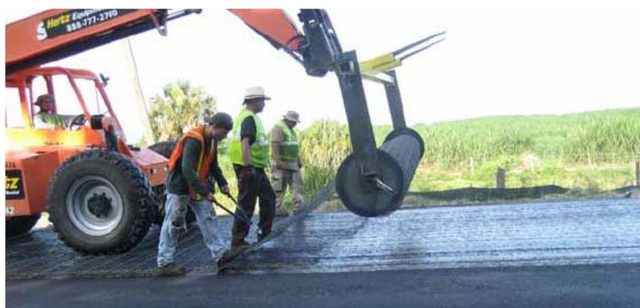
Figure 6.9: PaveTrac Mesh being Unrolled Correctly
