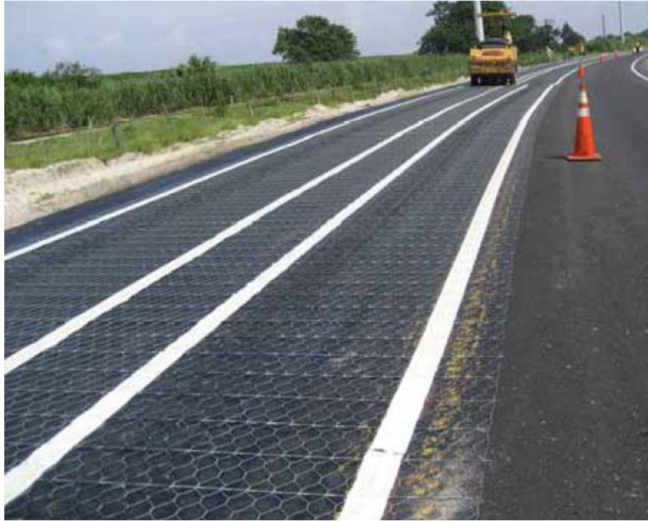
Figure 6.4: PaveTrac being Rolled with Qwick Seal Tape in Place
