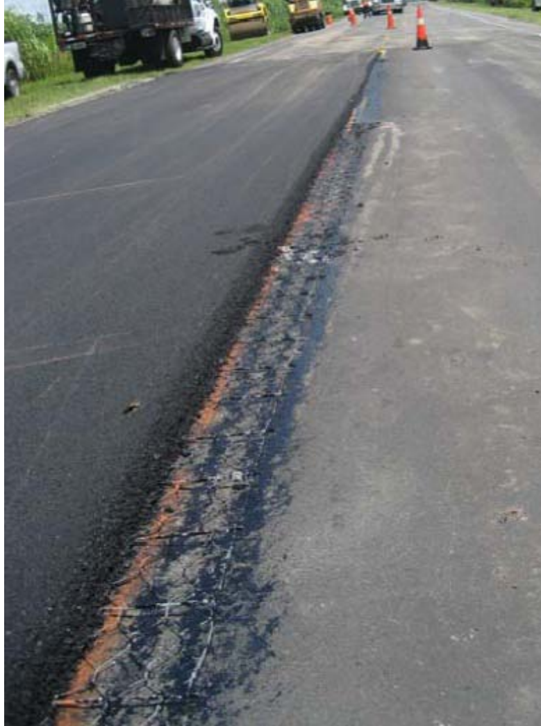
Figure 6.10: Six Inch Overlap of Material at Center of Road
