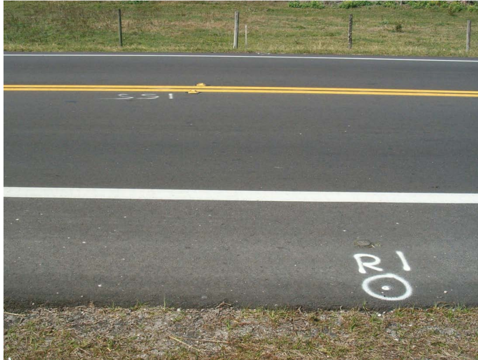
Figure 7.1: Smooth Road Surface on the Day of the 6-month Post-construction Tests
