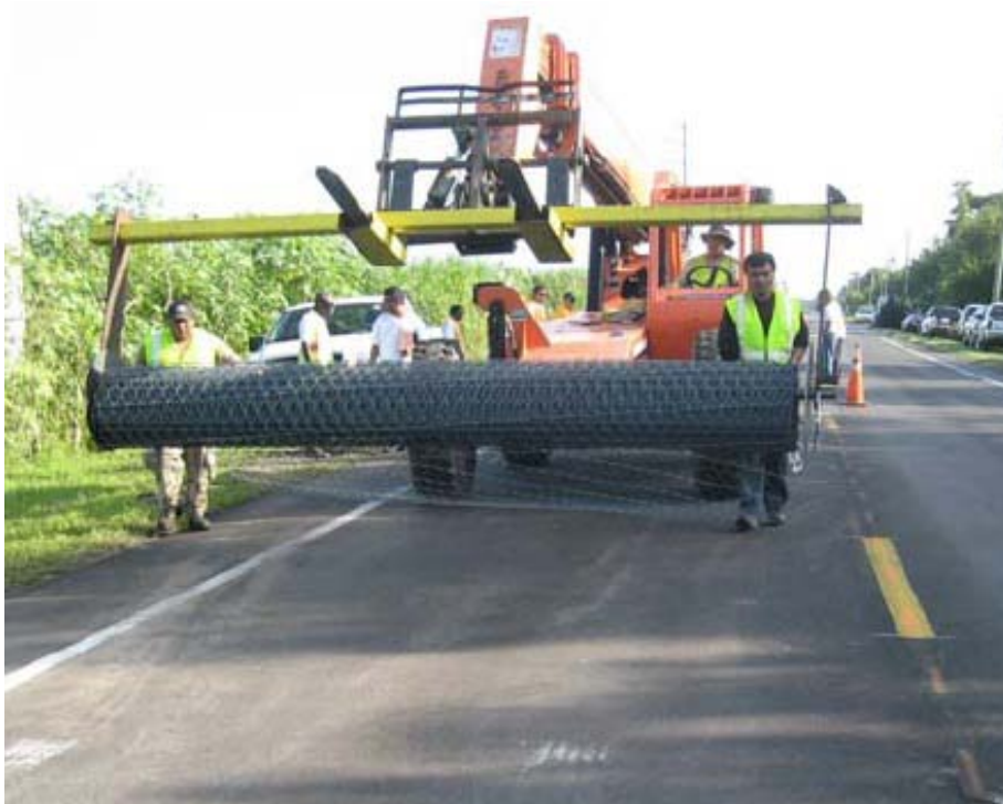
Figure 6.1: PaveTrac Installation, Section 2.3S
