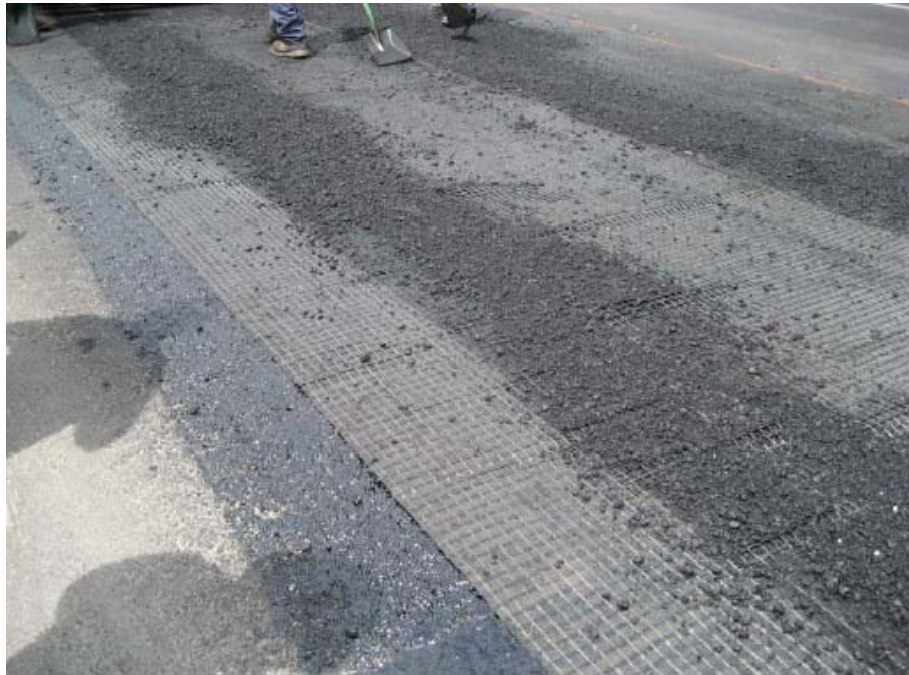
Figure 6.14: HMA Spread before the Paver Wheels
