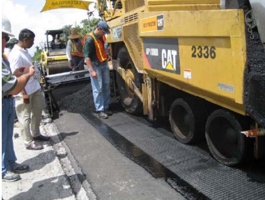
Figure 6.13: Pressing Down Wrinkles in the PetroGrid Mesh by Walking on it
