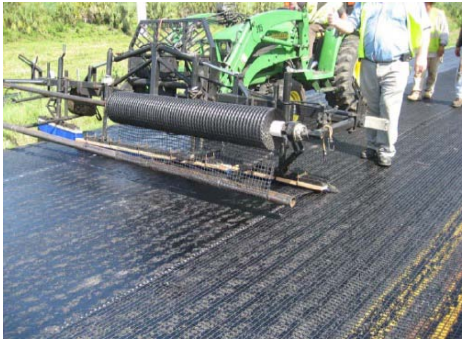
Figure 6.11: Special Fixture used to Place GlasGrid
