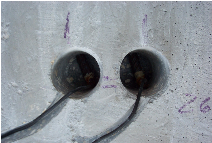
Figure 14: Photograph of two core holes with positioned reinforcing steel probes.
