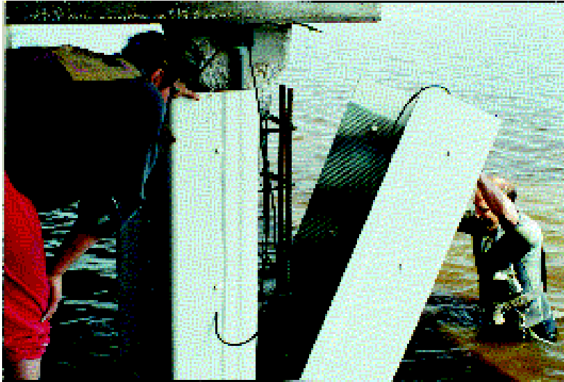
Figure 4: Photograph of a zinc mesh jacket installation (courtesy of D. Leng).
