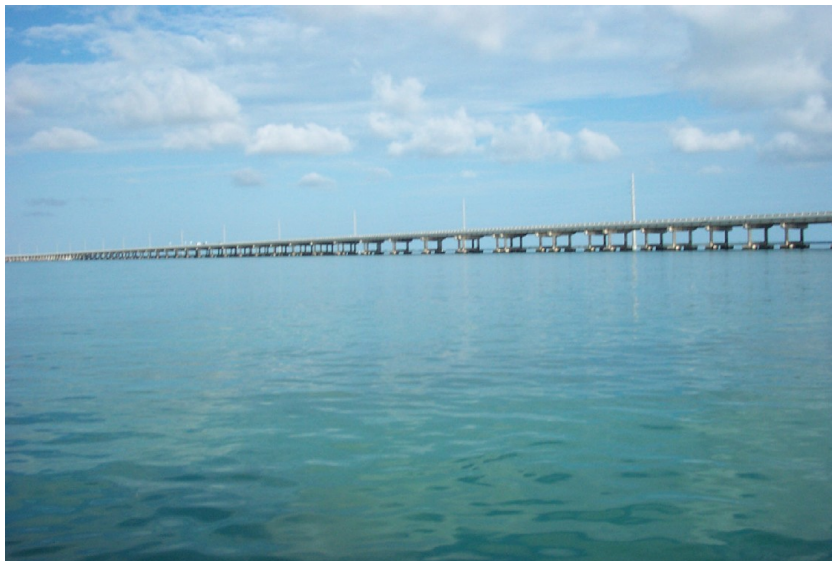
Figure 7: General view of the Bahia Honda Bridge.
