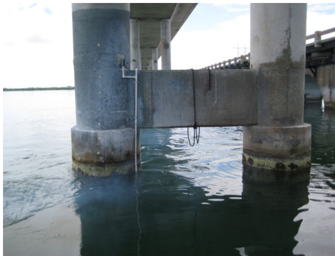
Figure 33: Photograph of Pier 2 subsequent to MgSBA installation.
