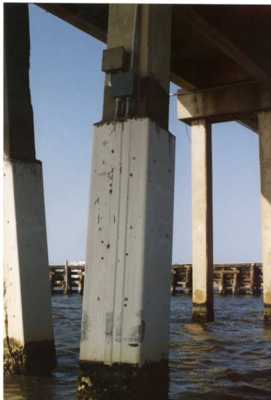
Figure 5: Photograph of an installed zinc mesh jacket.
