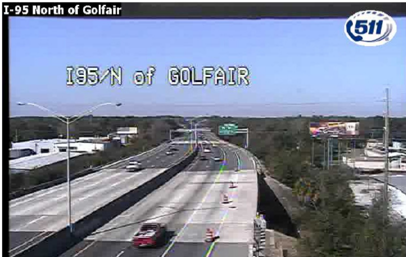
View from FDOT camera at the beginning of the work zone
