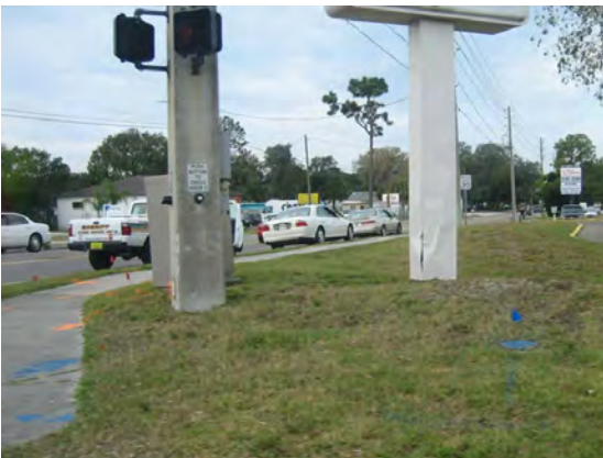
314 - Pasco County, Trouble Creek Road (CR 518) at Madison Street, pushbuttons in northwest corner of intersection cannot readily be accessed by persons with disabilities
