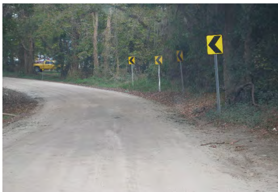
183 - Clay County, CR 15A, Chevrons in place looking east on North Road at second turn
