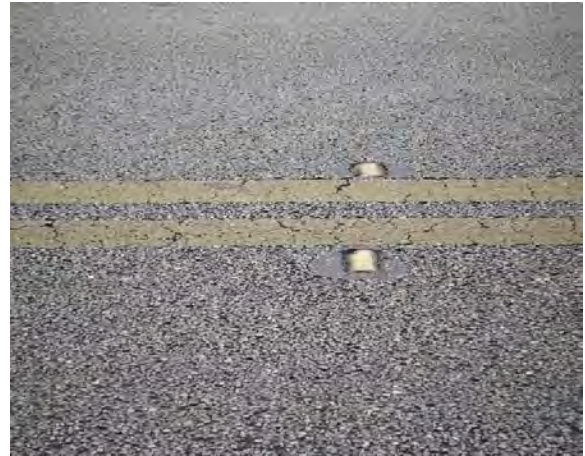
150 - Clay County, CR 209, RPMs buried in pavement
