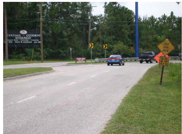
130 - Clay County, Wells Road, Chevrons mounted in double sided guardrail spaced along half of curve
