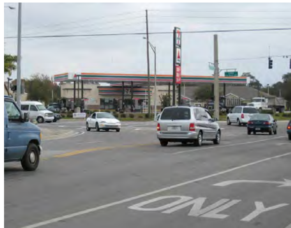
259 - Pasco County, Little Road (CR1) at Embassy Boulevard / Hilltop Drive, vehicles making eastbound left turns spill out into thru lane
