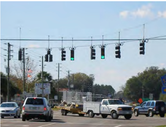
308 - Pasco County, SR 54 at Morris Bridge Road / Eiland Boulevard (CR 579), no approaches have white lights installed to aid red light running enforcement
