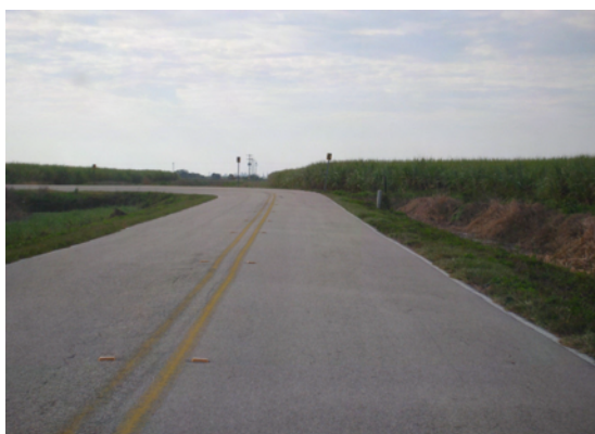
340 – Glades County, CR 720, power line and service road making public road appear to go straight
