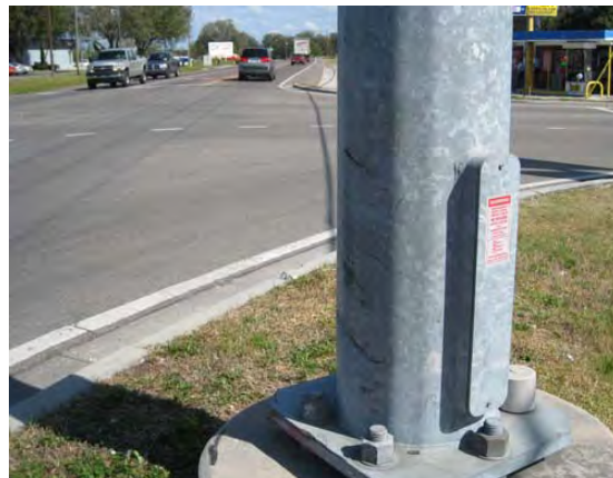
305 - Pasco County, SR 54 at Morris Bridge Road / Eiland Boulevard (CR 579), traffic signal pole on southwest corner of intersection appears to have been struck by vehicle
