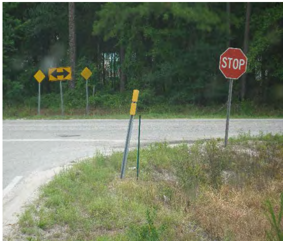
87 - Clay County, STOP sign is 18 feet from the edge line on CR 226
