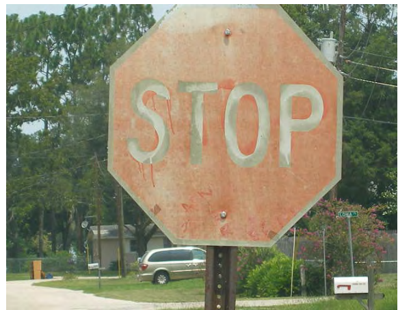
141 - Clay County, Parkwood Drive at Hilltop Drive, northbound STOP sign is faded
