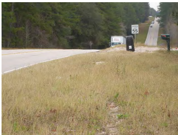
173 - Clay County, CR 215 sight distance at 12 feet from edge of pavement, 5 feet 8 inches above roadway, distance from photo location to 55 mph sign is approximately 400 feet
