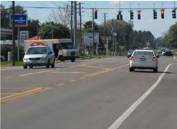
288 - Pasco County, SR 54 at Morris Bridge Road / Eiland Boulevard (CR 579), left turn queues stack past marked left turn storage west/northbound, turn lane storage westbound limited by business turn lanes
