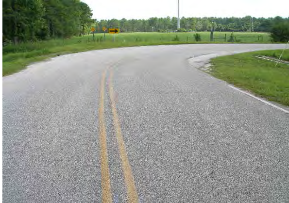
115 - Clay County, Mallard Road and CR 218, pavement markings through turn are worn
