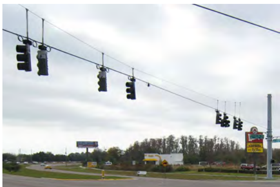
321 - Pasco County, Little Road (CR 1) at Rancho del Rio Drive, no backplates for traffic signal heads
