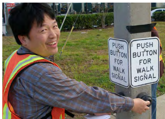
271 - Pasco County, Ridge Road (CR 587) at Regency Boulevard, pushbuttons not up to current standards making it difficult for pedestrians to tell which button controls which crossing
