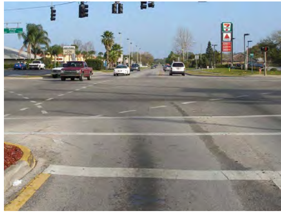
267 - Pasco County, Ridge Road (CR 587) at Regency Boulevard, skip guide lines provided at intersection for southbound thru movement, but no markings provided for northbound movement
