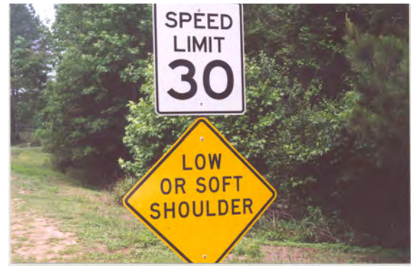
337 – Gadsden County, example of sign mixing
