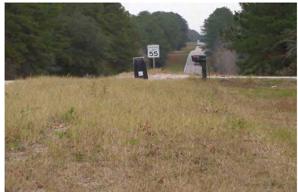
172 - Clay County, view of shoulder condition looking north from east side at Chicory Avenue. Shoulder is approximately 12 inches above the CR 215 edge of pavement
