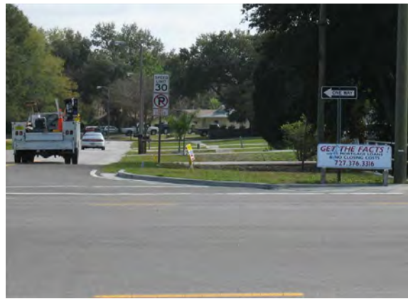
281 - Pasco County, Little Road (CR 1) at Saint Lawrence Drive, one way signs at intersection do not appear to meet MUTCD standards for median openings 30 feet wide or greater
