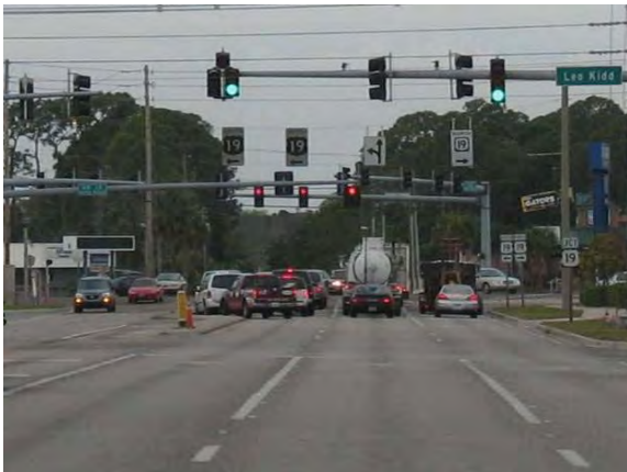
274 - Pasco County, Ridge Road (CR 587) at Leo Kidd Avenue , two signal heads for three thru lanes
