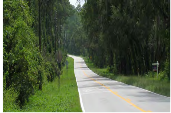
362 – Hernando County, Powell Road at Saturn Road, paved shoulders currently absent for both intersection approaches
