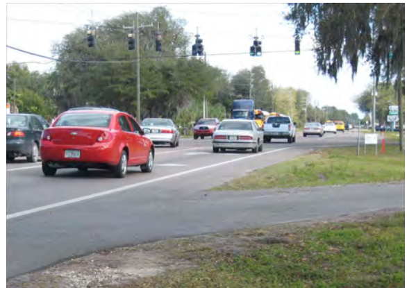
330 - Pasco County, SR 54 at Dean Dairy / Coats Road, view of street name signs eastbound and westbound limited by overhanging tree limbs; lack of signs indicating name of upcoming signalized intersection along corridor
