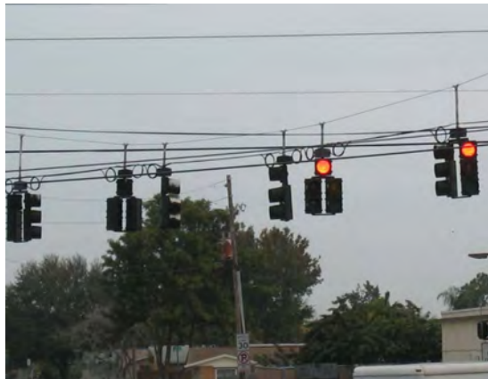
309 - Pasco County, Trouble Creek Road (CR 518) at Madison Street, no backplates for traffic signal heads and overhead cables impede signal indication view for northbound approach
