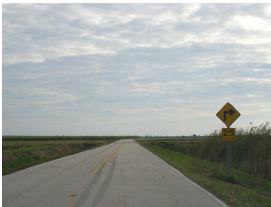
338 – Glades County, CR 720, looking east from just west of first curve, (note skid marks on pavement and lack of shoulders and presence of deep, shallow side ditches)
