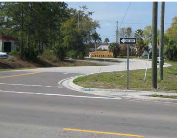
282 - Pasco County, Little Road (CR 1) at Saint Lawrence Drive, unmarked horizontal curves present at far side of intersection for eastbound and westbound approaches
