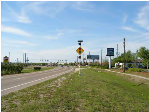
191 - Pasco County, Little Road at Rancho Del Rio Drive after flashers were installed
