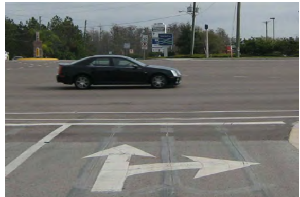
322 - Pasco County, Little Road (CR 1) at Rancho del Rio Drive, eastbound thru approach does not line up with respective receiving lanes
