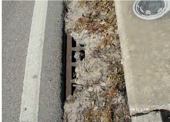
307 - Pasco County, SR 54 at Morris Bridge Road / Eiland Boulevard (CR 579, blocked drain around intersection
