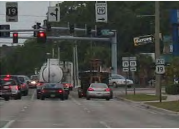
278 - Pasco County, Ridge Road (CR 587) at Leo Kidd Avenue, US 19 junction sign close to intersection not allowing drivers time to change to appropriate lane
