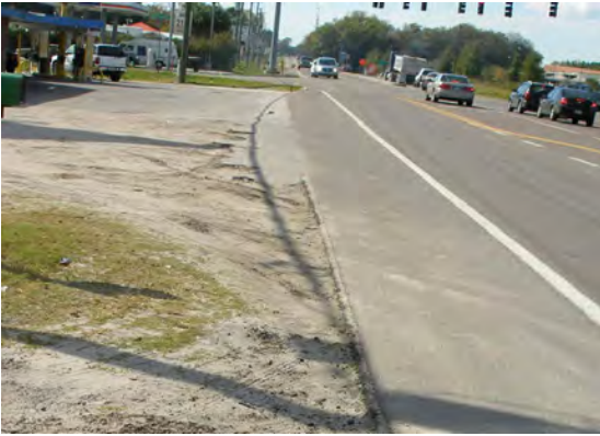
300 - Pasco County, SR 54 at Morris Bridge Road / Eiland Boulevard (CR 579), southeast quadrant of intersection appears to be one continuous unrestricted driveway
