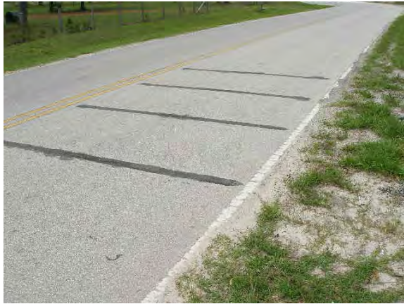
206 - Clay County, Thunder Road, rumble strips on the northbound approach to the STOP condition at the first turn
