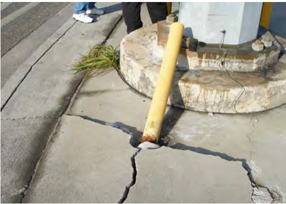
268 - Pasco County, Ridge Road (CR 587) at Regency Boulevard, bollards protecting utility pole by 7-Eleven driveway on westbound intersection approach have been damaged
