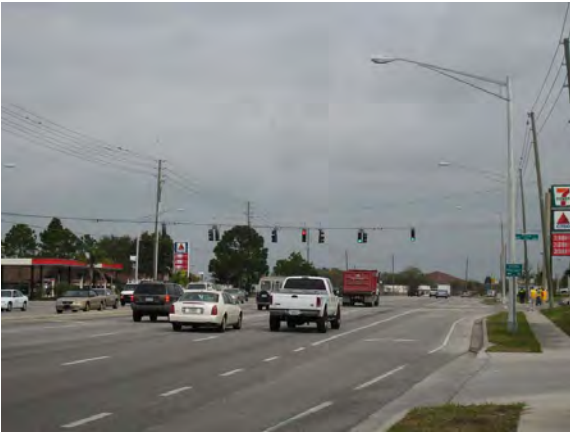
266 - Pasco County, Ridge Road (CR 587) at Regency Boulevard, no signs indicating name of next signalized intersections along corridor
