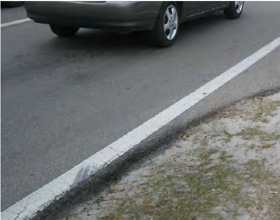
312 - Pasco County, Trouble Creek Road (CR 518) at Madison Street, pavement drop-off on westbound approach to business driveway where no shoulder is present on Trouble Creek Road
