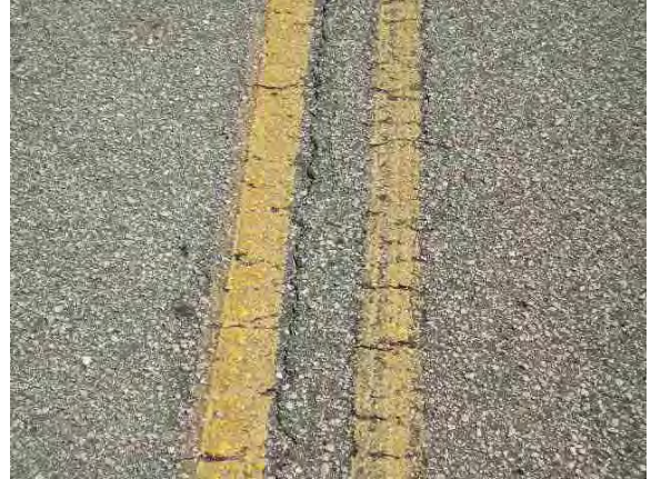
104 - Clay County, CR 315C and Bellamy Road, typical condition of centerline in the entire reviewed section
