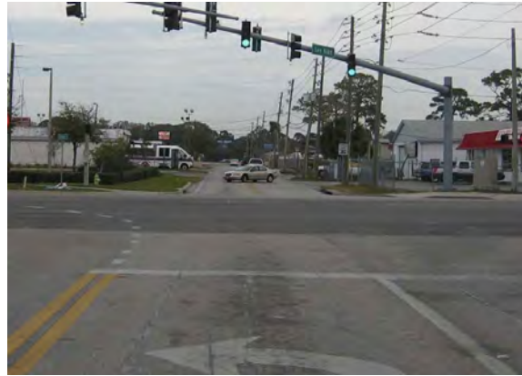
279 - Pasco County, Ridge Road (CR 587) at Leo Kidd Avenue, southbound thru lane lines up with northbound left turn lane
