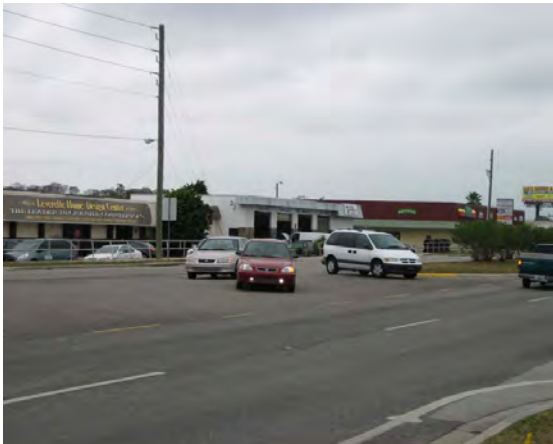
244 - Pasco County, Ridge Road (CR 587) at Sterling Lane, drivers stack in the center of the full median opening
