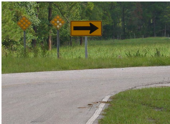
113 - Clay County, Mallard Road and CR 218, missing object marker, centerline and edge line through turn
