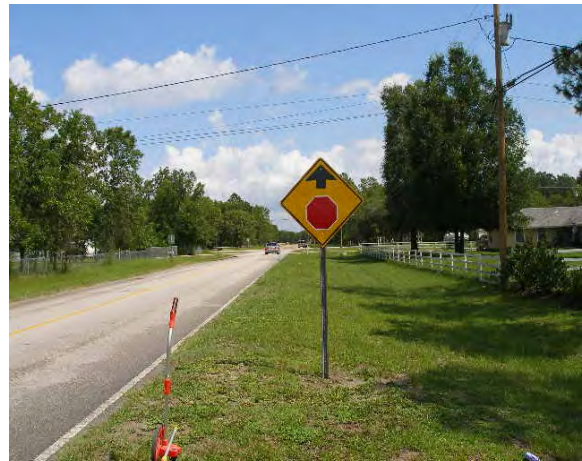
124 - Clay County, N Mimosa Avenue intersection with John's Cemetery Road, STOP Ahead is a 30" sign mounted 5 feet above the top of the edge of pavement
