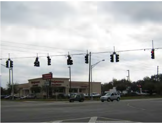
250 - Pasco County, Little Road (CR1) at Embassy Boulevard / Hilltop Drive, traffic signal heads do not have blackplates
