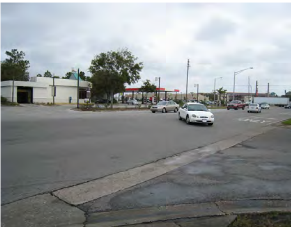
258 - Pasco County, Little Road (CR1) at Embassy Boulevard / Hilltop Drive, vehicles conflicting with each other at full median opening for driveway approximately 200 feet west of CR1 and Embassy Boulevard intersection
