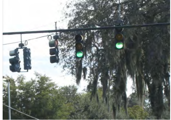
328 - Pasco County, SR 54 at Dean Dairy / Coats Road, overhead cables impede view of traffic signal on southbound approach plus traffic signals blend in with background
