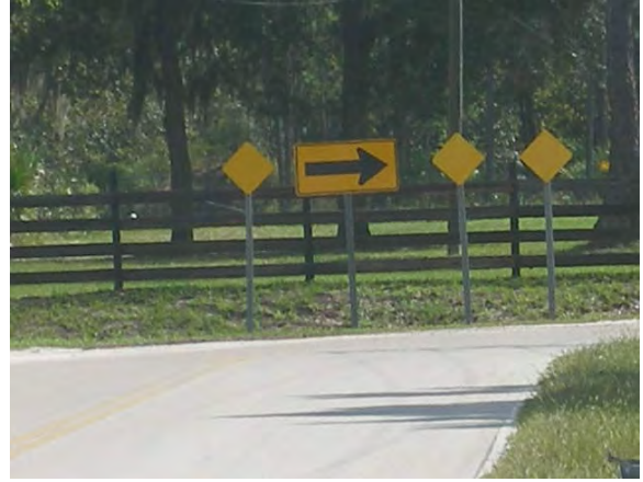
205 - Clay County, Thunder Road, turn assembly signage has not been brought to standard per Florida DOT Design Standard Index No. 17349, Case I
