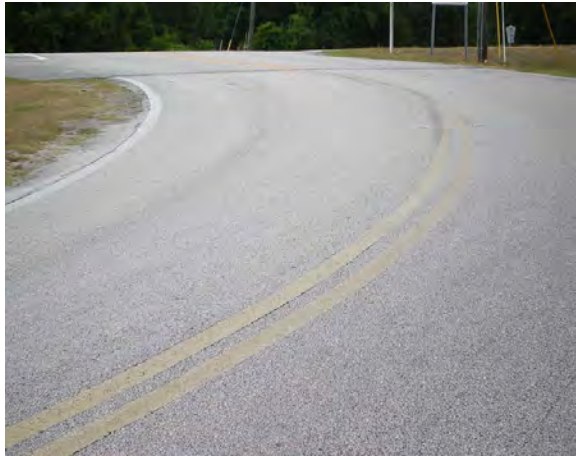
149 - Clay County, CR 209, faded double solid yellow centerline
