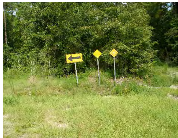
120 - Clay County, Mallard Road and CR 218, one object marker missing
