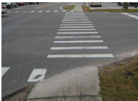
315 - Pasco County, Trouble Creek Road (CR 518) at Madison Street, ramps leading to pedestrian crossings on all four corners of intersection do not have truncated domes installed
