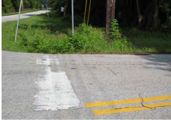
342 – Hernando County, Mondon Hill Road and McIntyre Road, worn STOP Bar
