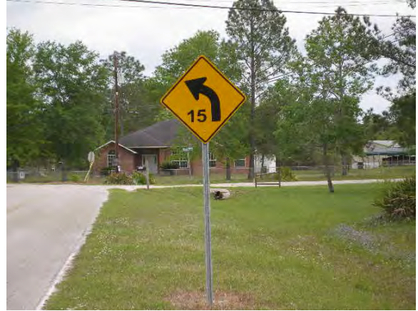
197- Clay County, Mallard Road ½ mile south of CR 218, new curve sign with advisory speed determined by using a ball bank indicator
