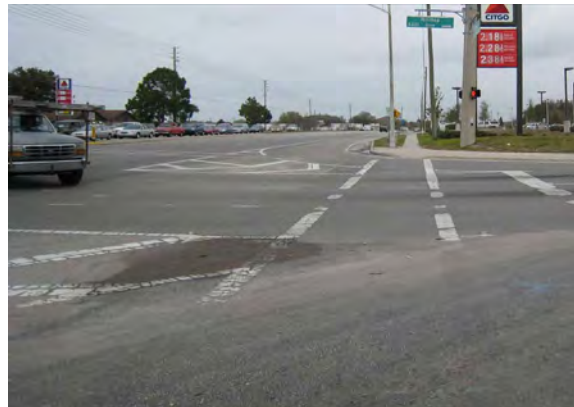
257 - Pasco County, Little Road (CR1) at Embassy Boulevard / Hilltop Drive, pavement markings worn and RPMs missing
