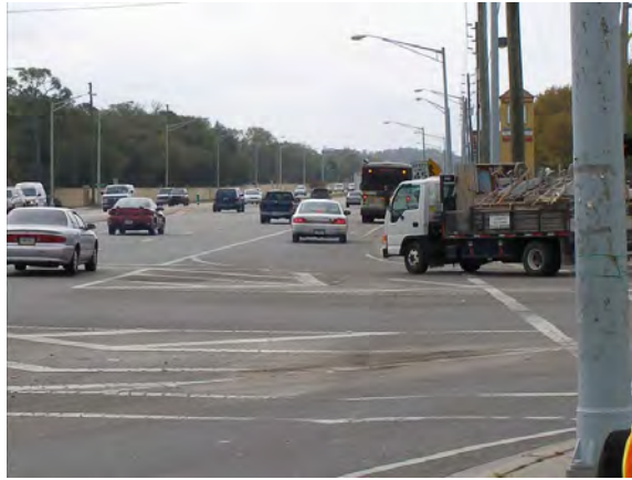
261 - Pasco County, Little Road (CR1) at Embassy Boulevard / Hilltop Drive, vehicle and bus conflict accentuated by driveways on the north and south side of intersection in merge lanes beyond the bus stops
