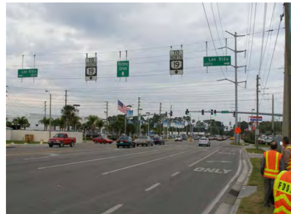
192 - Pasco County, Ridge Road at Leo Kid Avenue, overhead signs potentially take away driver attention from traffic signals, overhead street name signs reduce driver attention to traffic signal at Leo Kidd
