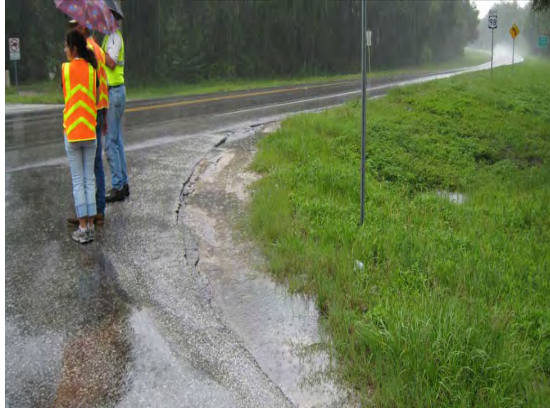
379 – Hernando County, Lake Lindsey Road at Ponce de Leon Boulevard, damaged intersection shoulders along with ponding
