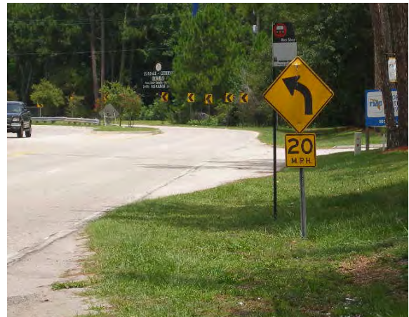
132 - Clay County, Well Road, westbound direction, curve sign is approximately 600 feet west of a signalized intersection, Chevrons continued about half way through the curve
