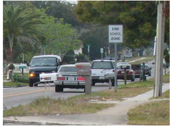
318 - Pasco County, Madison Street at Cecilia Drive, northbound approach into school zone does not seem to be designated by pavement markings
