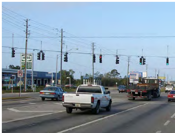
263 - Pasco County, Ridge Road (CR 587) at Regency Boulevard, traffic signal heads do not have blackplates
