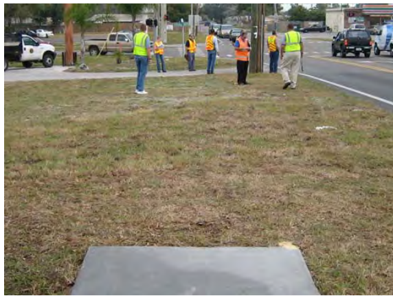
313 - Pasco County, Trouble Creek Road (CR 518) at Madison Street, sidewalk not continuous on southwest corner of intersection
