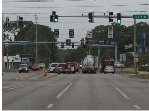
273 - Pasco County, Ridge Road (CR 587) at Leo Kidd Avenue , no traffic signal heads have backplates
