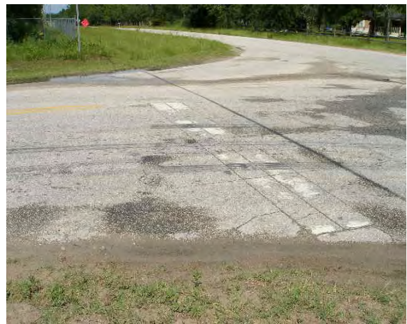
126 - Clay County, N Mimosa Avenue intersection with John's Cemetery Road, STOP bar is worn
