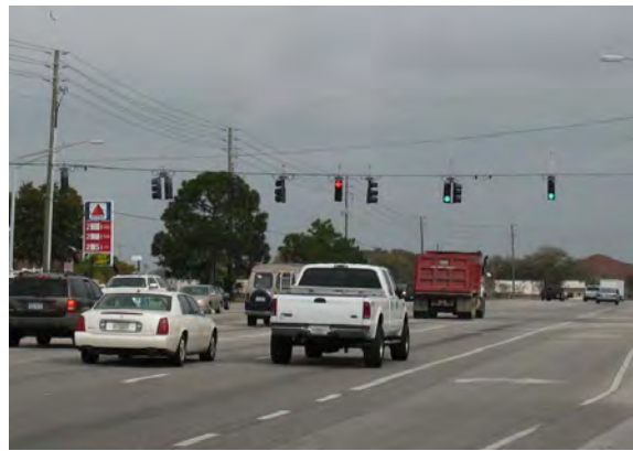
251 - Pasco County, Little Road (CR1) at Embassy Boulevard / Hilltop Drive, north and southbound approaches each have two signal heads serving the three thru lanes
