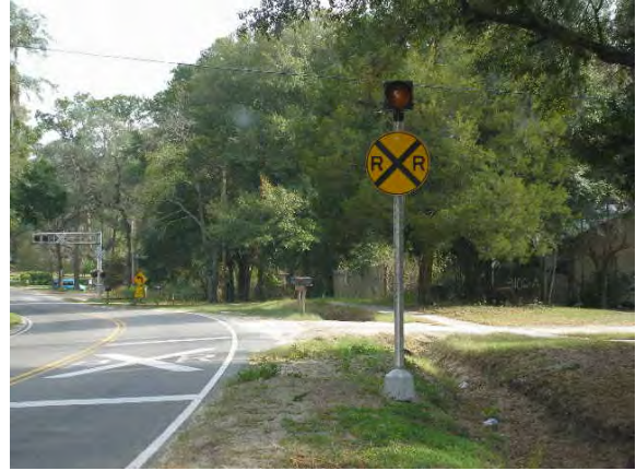
186 - Clay County, CR 224A (Peoria Road) at RXR, replaced RXR warning sign with new sign mounted with warning light
