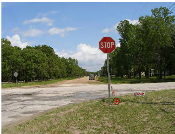
125 - Clay County, N Mimosa Avenue intersection with John's Cemetery Road, STOP sign is a 30" sign in excellent condition
