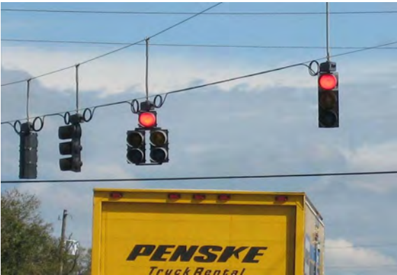
286 - Pasco County, SR 54 at Morris Bridge Road / Eiland Boulevard (CR 579), no backplates on traffic signal head
