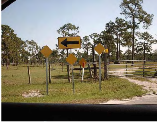
56 – Okeechobee County, 128 Terrace SE with new object markers
