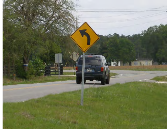
201 - Clay County, CR 739A (Sandridge Road) near Feed Mill Road, original sign upgraded to high intensity grade sheeting and relocated
