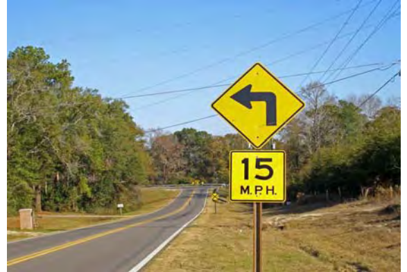
76 - Gadsden County, CR 268, Martin Luther King Boulevard at Brick Yard Road, new turn sign with 15 mph advisory speed sign attached
