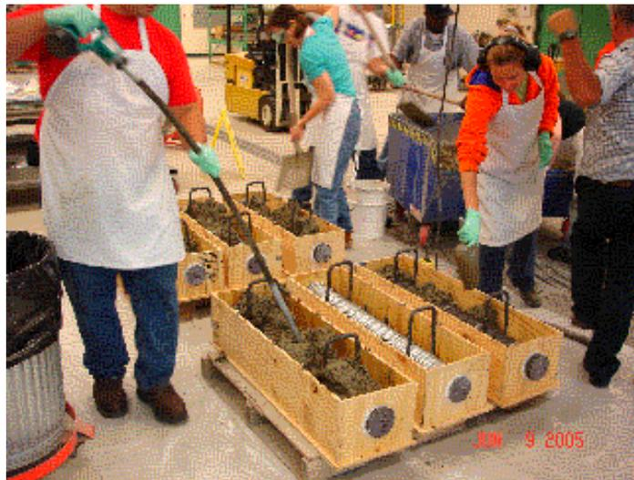
**Figure 4. FDOT and UF Personnel Pour Concrete into Slab Forms**
