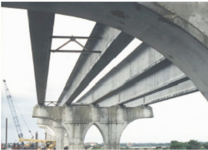
Long girders on bearing supports
