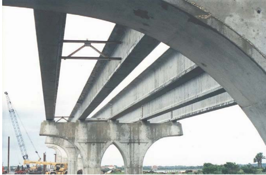
Figure 1.4 Florida bulb-tee girders placed on bearings (Vilano Beach Bridge, Florida / Photo credit: Florida DOT)
