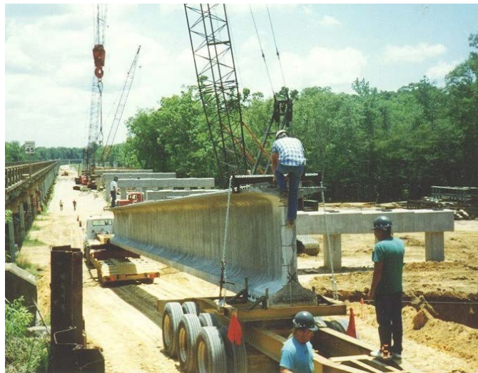
Figure 1.3 Transport of Florida bulb-tee girders to bridge construction site (State Road 20 Bridge over the Apalachicola River, Florida / Photo credit: Florida DOT)
