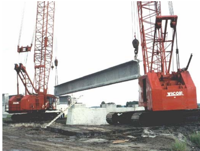
Figure 1.2 Lifting Florida bulb-tee girders for placement onto supports (Vilano Beach Bridge, Florida / Photo credit: Florida DOT)
