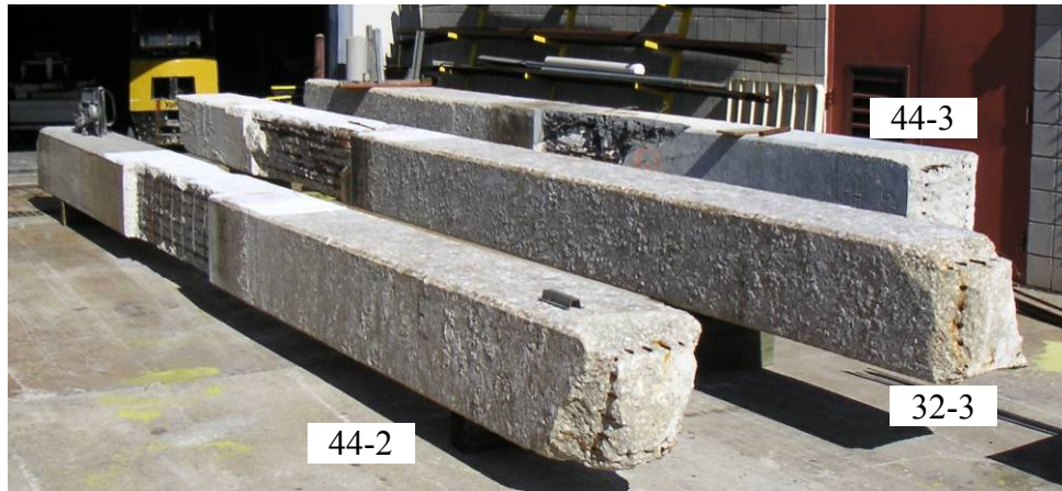
Figure 27 – Piles being excavated to examine corroded strand.
