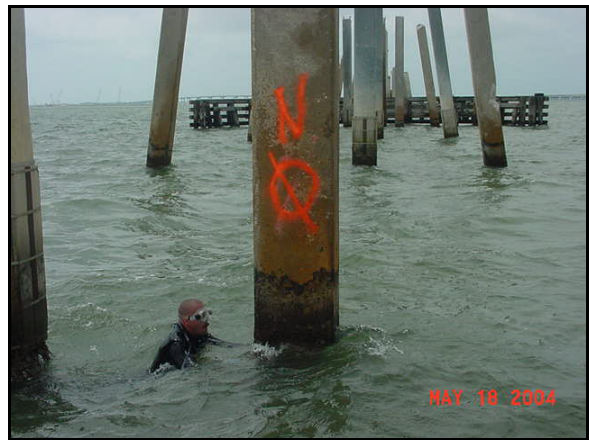
NORTH FACE PILE 39-2
