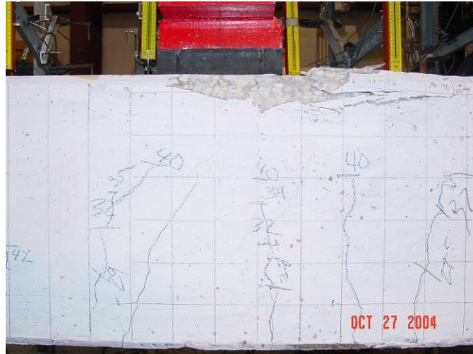
Figure 20 – Compression zone crushing and flexural cracking in pile 44-2
