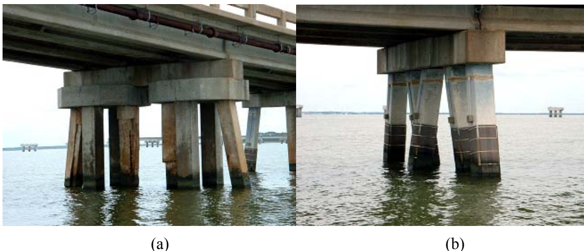
Figure 3 – Prestressed pile bents before bridge demolition. (a) “crutch bents” installed to relieve piles damaged by corrosion (b) cathodic protection system on existing piles
