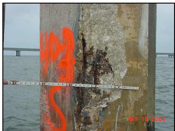
SOUTHEAST CORNER PILE 40-3J
