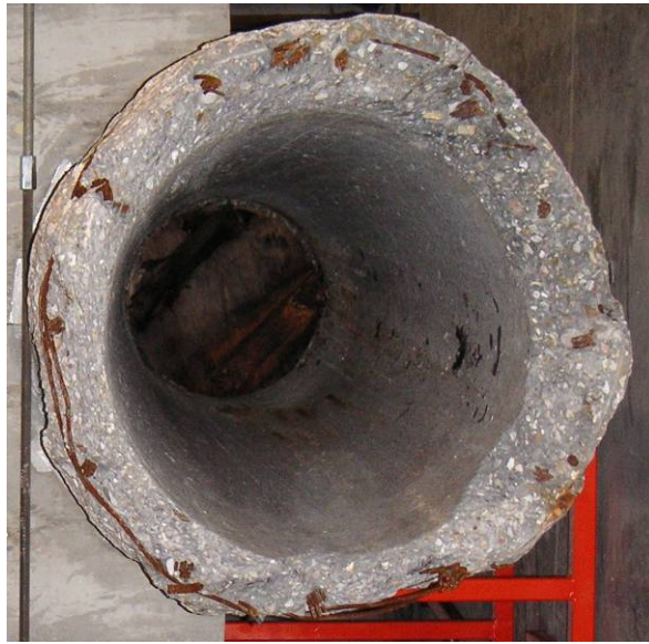
Figure 39 – Open end of pile
