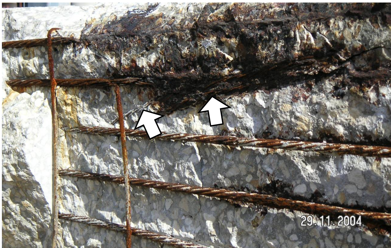
Figure 29 – Severely corroded strand from pick up point on Pile 32-3J. Prestressing strand in this area has been completely consumed by corrosion. Moderate to severe corrosion on the remaining strands as they enter the splash zone.
