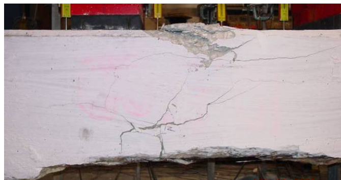
Figure 22 – Combination of strand rupture and crushing of compression zone on pile 40-3J. Spalling seen on bottom of pile was caused by corrosion of the strand in service.
