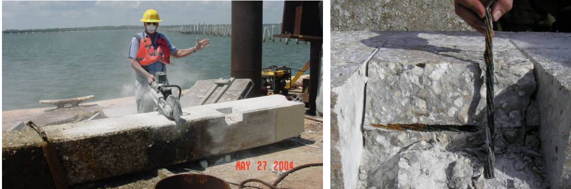
Figure 12 – Saw cut and strand removal
