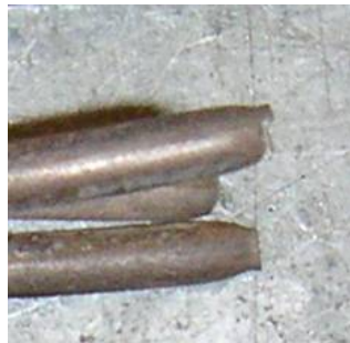
Figure 34 – Failure mode of uncorroded prestressing strand sample taken from pile 44-2. Ductile necking of the cross section and cup/cone fracture surface are shown.
