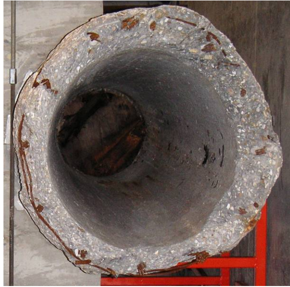
Figure 39 – Open end of pile
