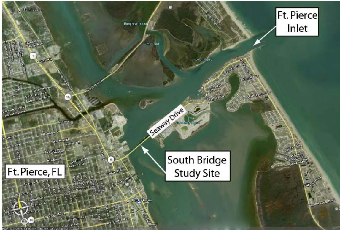
Figure 2 Aerial photograph showing test pier location relative to Fort Pierce Inlet.
