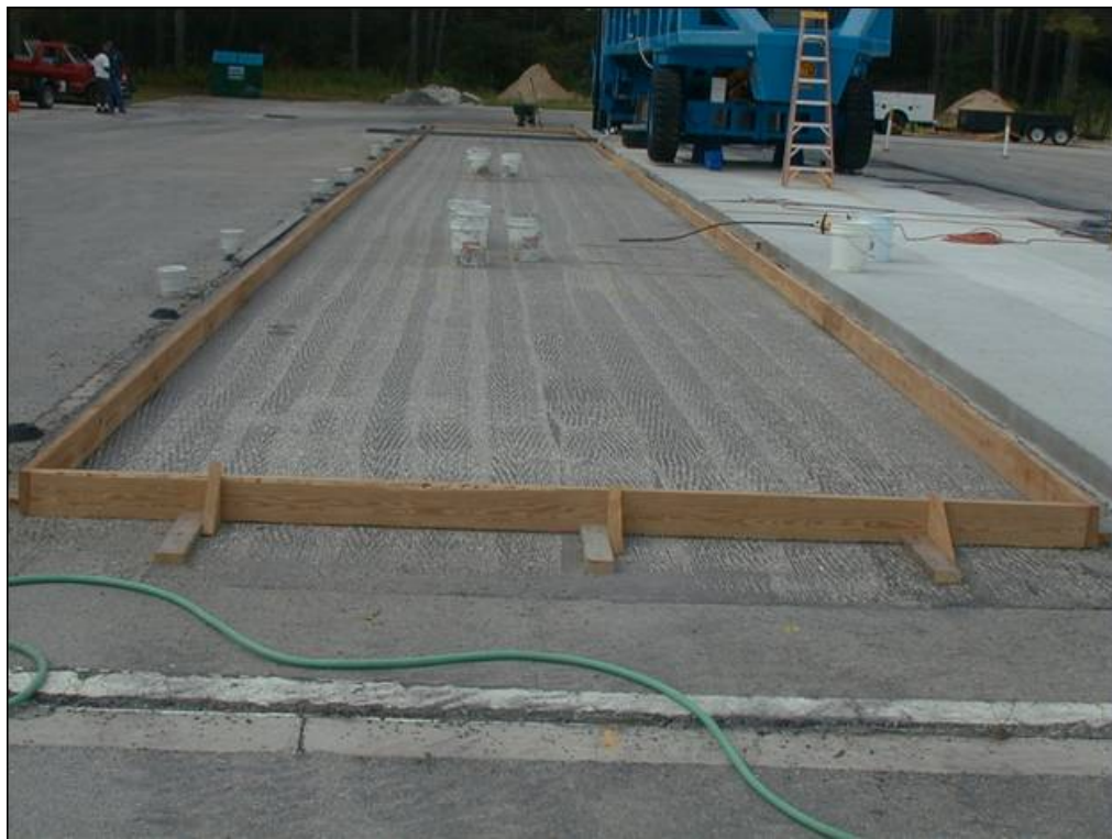
Figure 3.14. Formwork Prepared for Lane 7 in Phase I-b.
