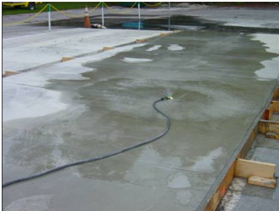
Figure 3.24. Curing of Concrete by Sprinkling with Water.
