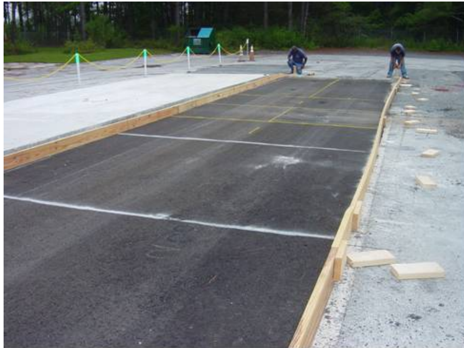
Figure 3.20. Formwork for Test Slabs in Phase II.
