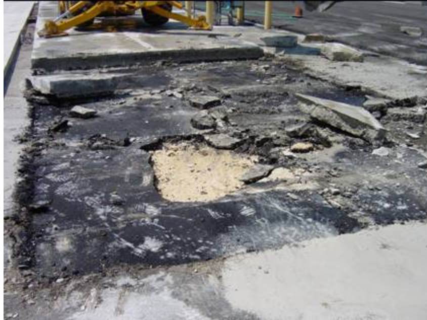
Figure 3.19. Removal of Concrete Slabs from Lane 6 in Phase I-a.
