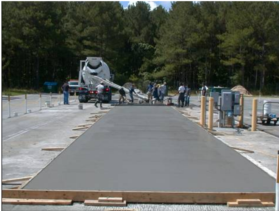
Figure 3.15. After Placement of Concrete on Lane 6 in Phase I-a.
