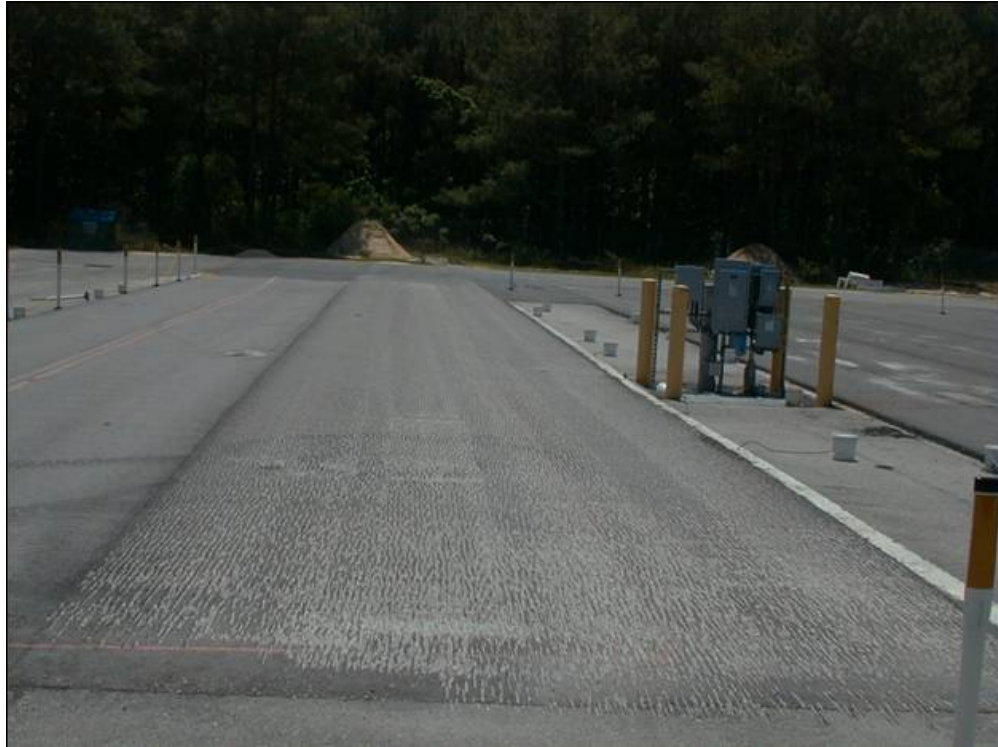
Figure 3.13. Milled Surface Before Concrete Placement on Lane 6 in Phase I-a.
