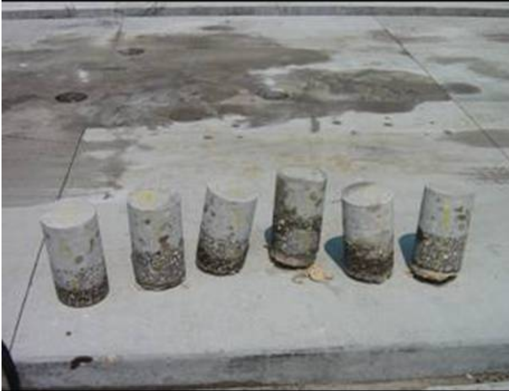
Figure 5.1. Cores Samples from Lane 6 in Phase I-a After HVS Loading.
