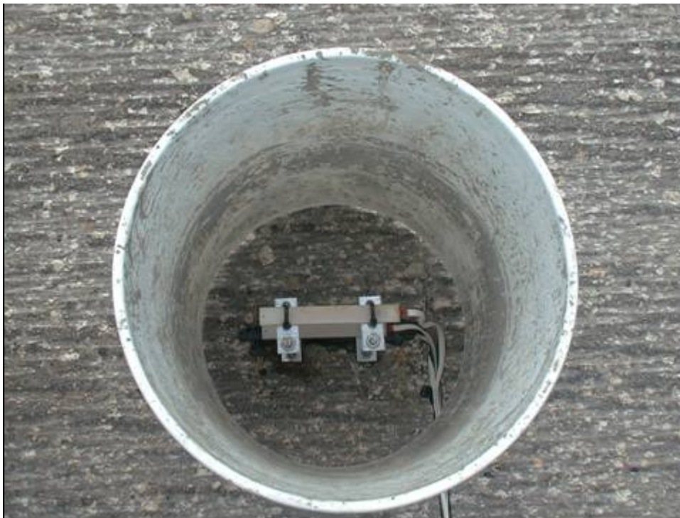
Figure 3.18. Strain Gages in a Protective PVC Pipe Before Placing Concrete.
