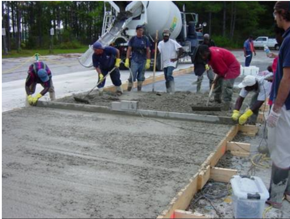
Figure 3.23. Finishing of the Concrete for the Test Track in Phase II.
